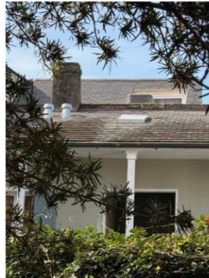
615 DAUPHINE STREET EXISTING ROOFTOP MECHANICAL WELL
