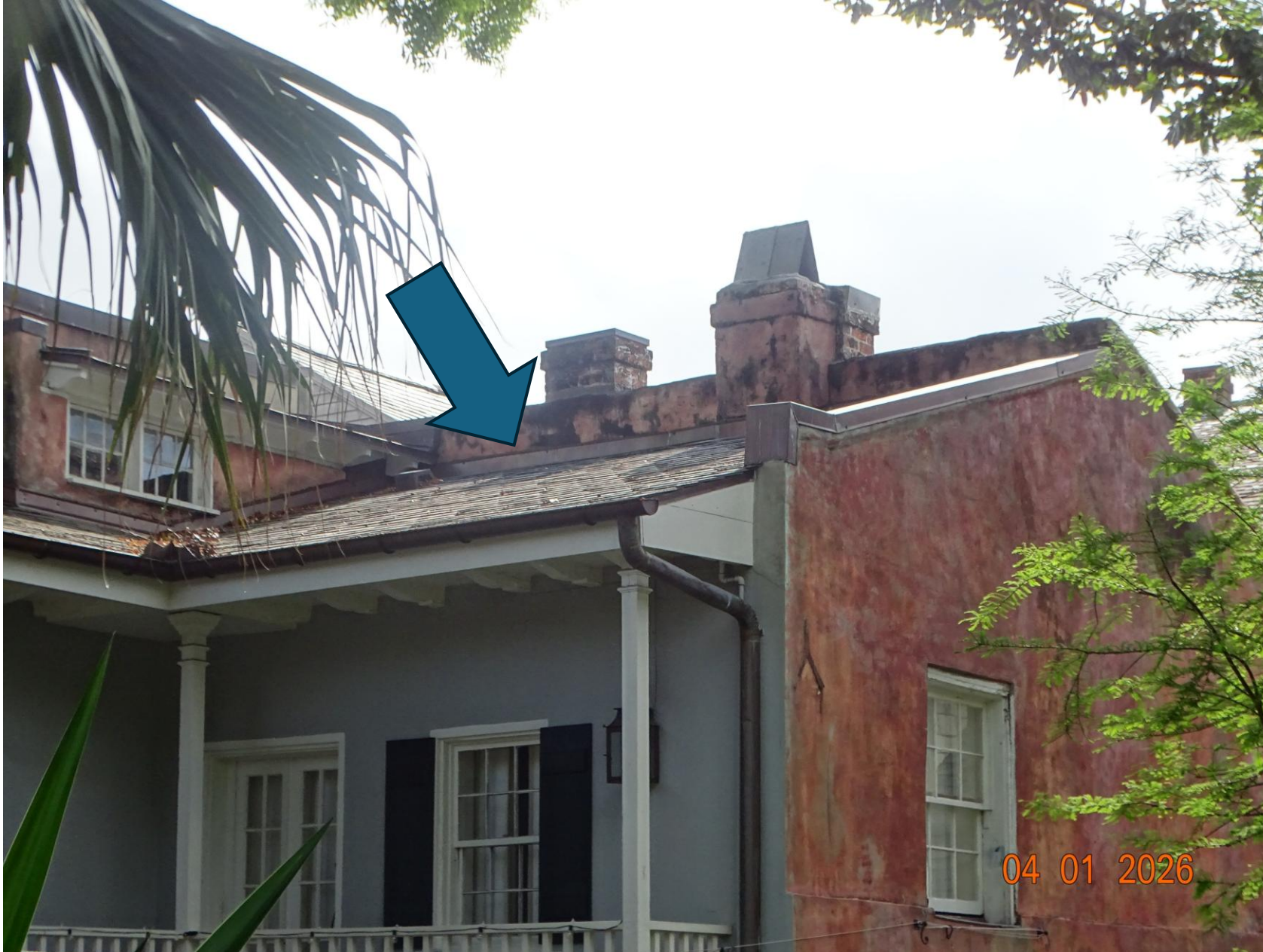
631 Dauphine – Rear roof slope of rear building. Potential secondary mechanical location
