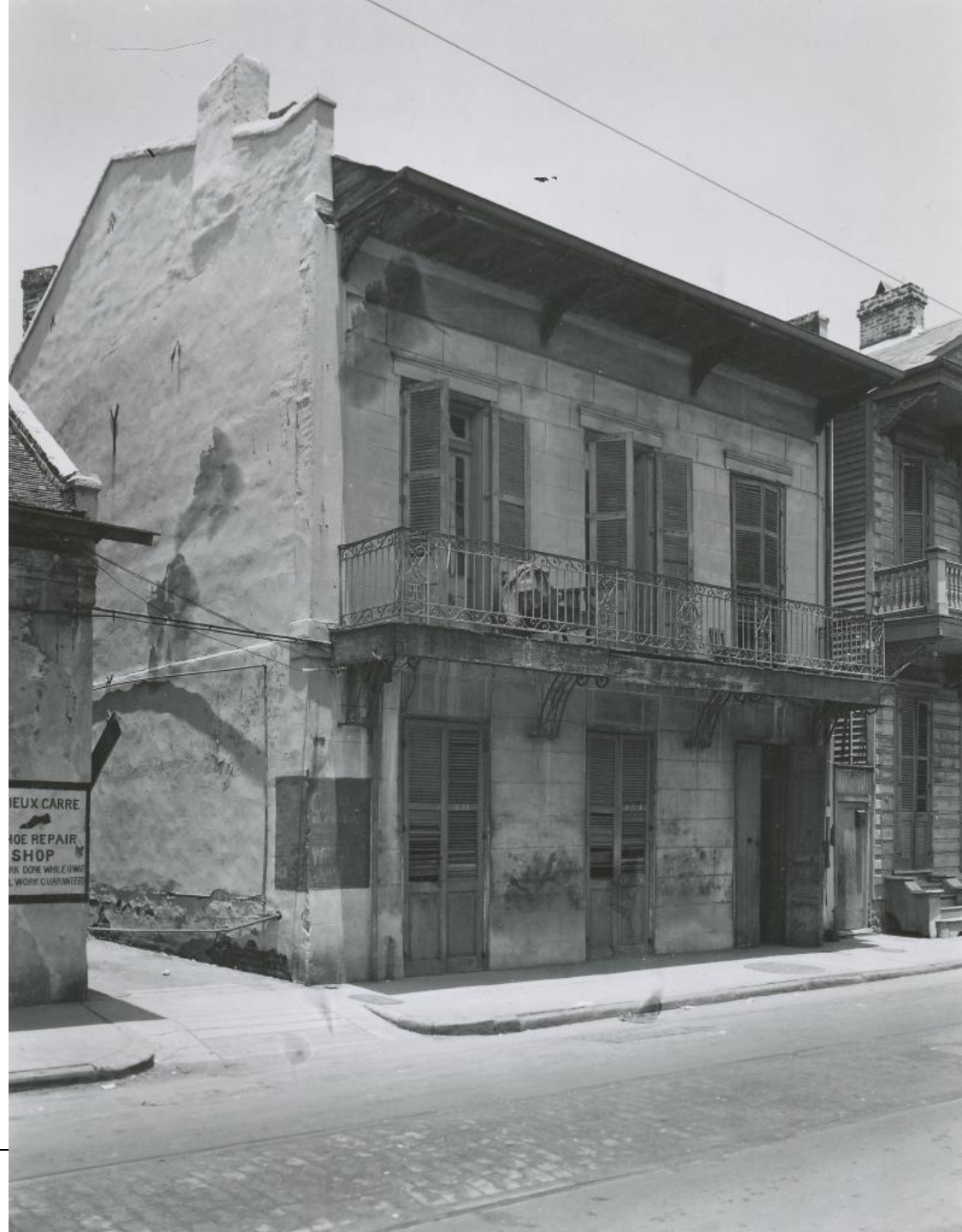
631 Dauphine – ca. 1939 VCC Architectural Committee
