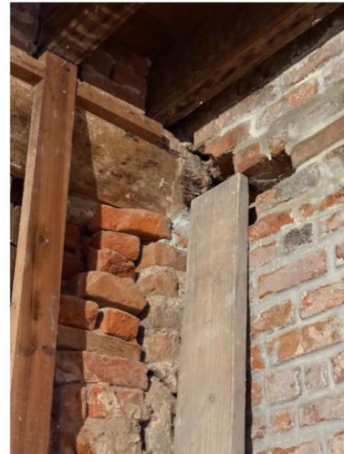
EXISTING INTERIOR LOAD BEARING WALLS
