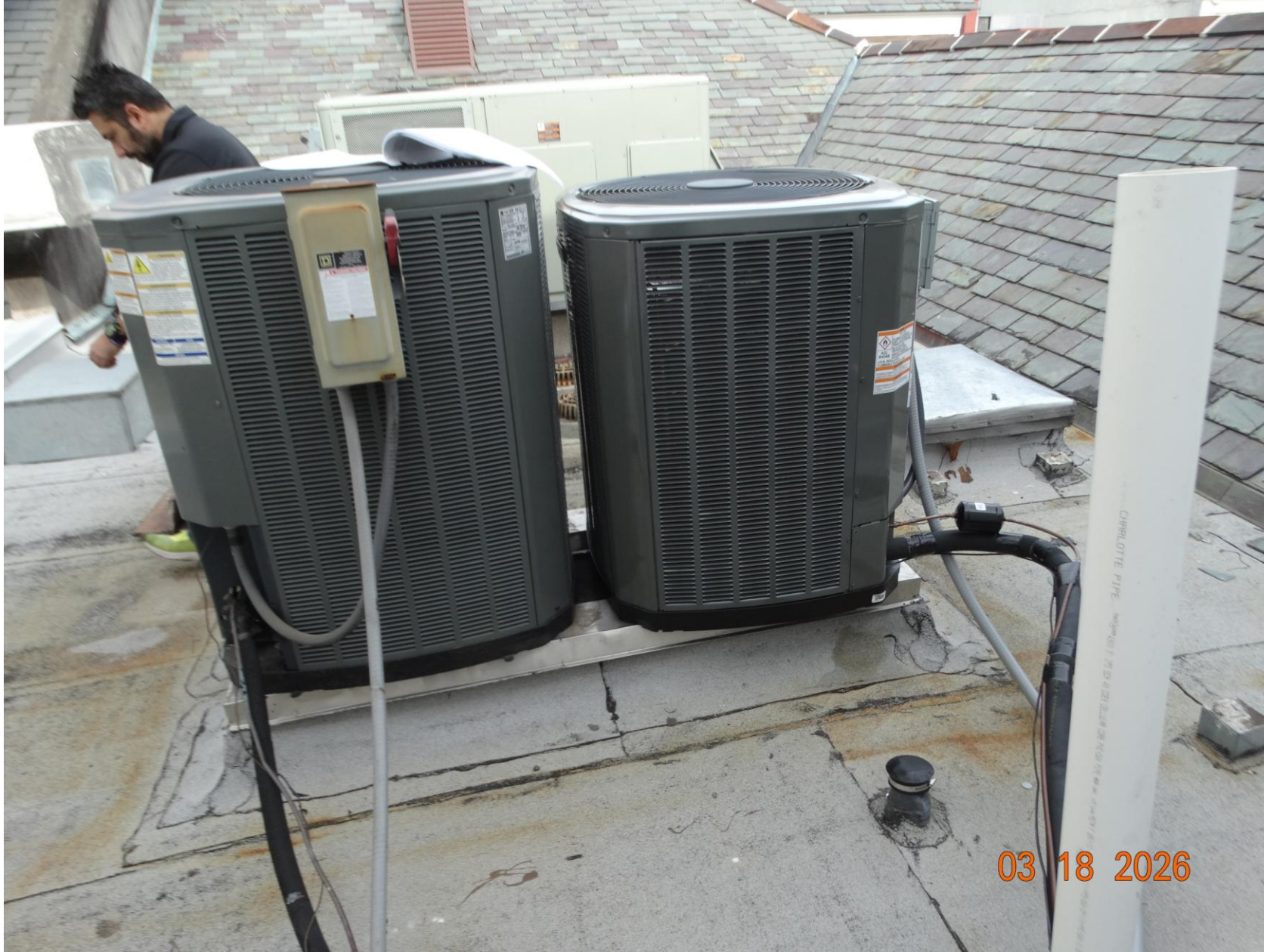
240 Royal – as-built roof conditions
