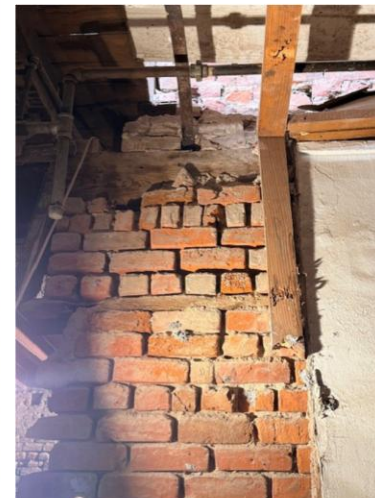
EXISTING INTERIOR LOAD BEARING WALLS
