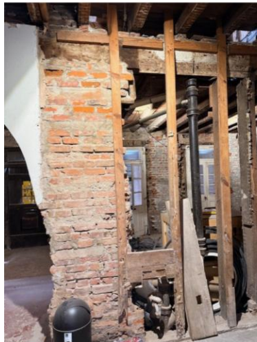
EXISTING INTERIOR LOAD BEARING WALLS
