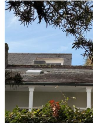
615 DAUPHINE STREET EXISTING ROOFTOP MECHANICAL WELL
