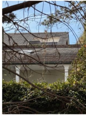
615 DAUPHINE STREET EXISTING ROOFTOP MECHANICAL WELL
