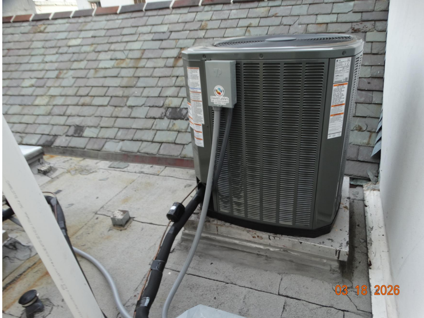
240 Royal – as-built roof conditions
