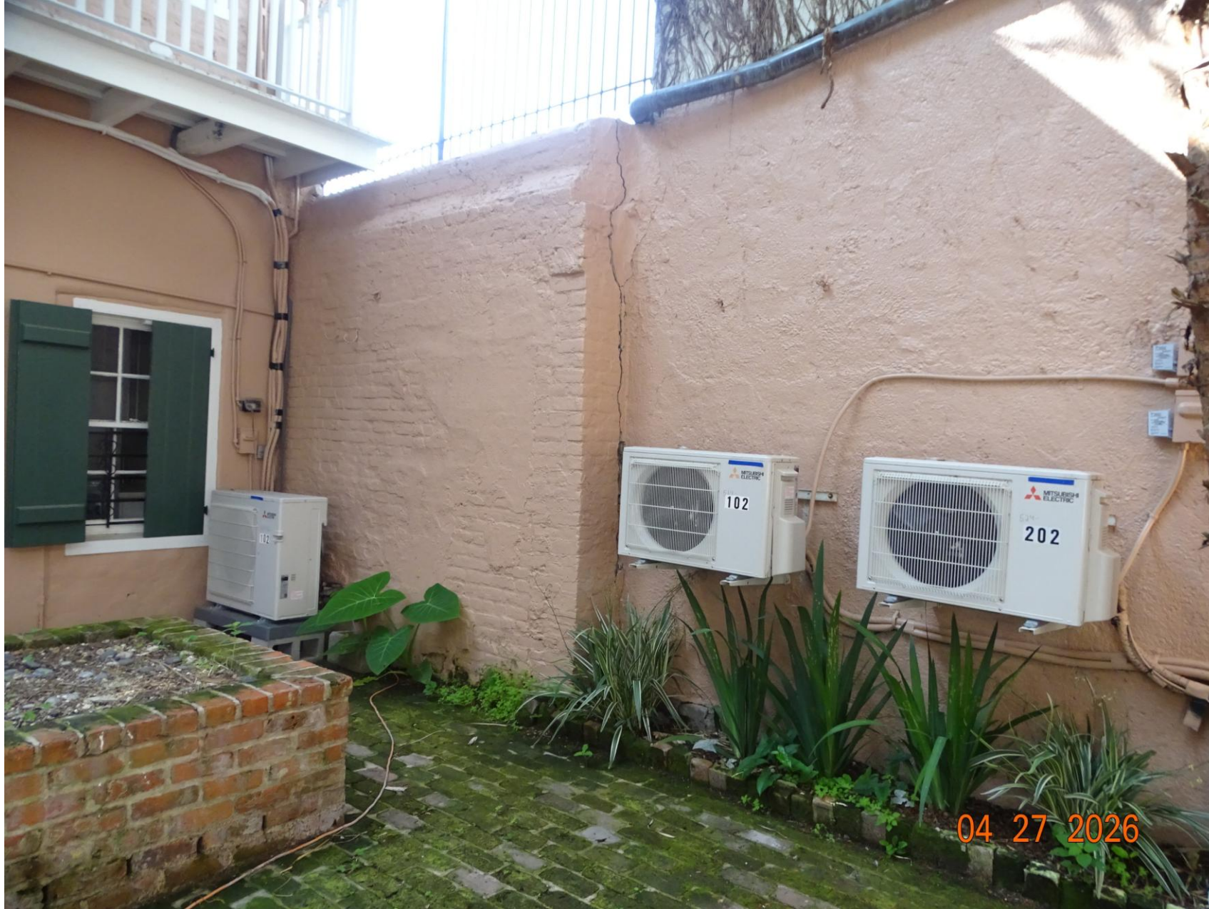
518 Governor Nicholls – After Renovation
