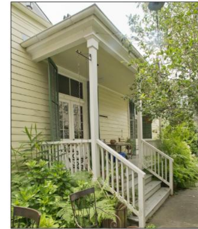
Simplified, but compatible trim and details used at this side porch addition include the wood cornice, support posts and railings.
