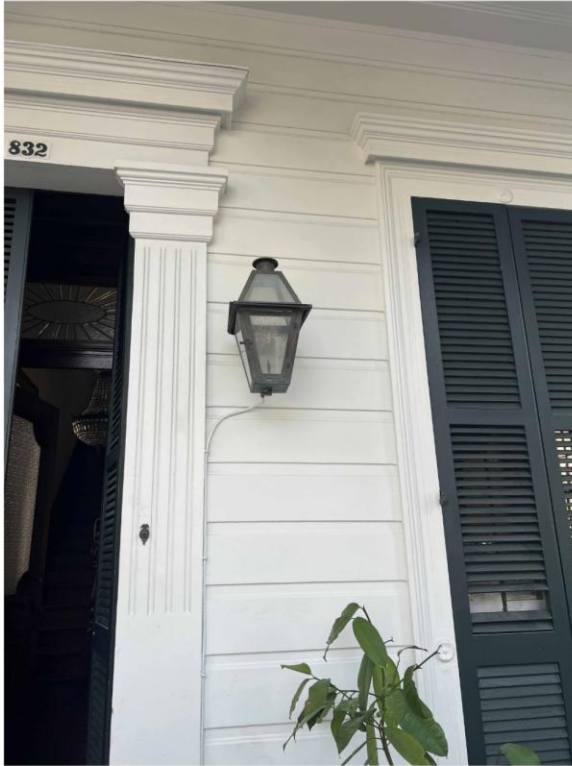
PHOTO A (EXISTING GAS LANTERN)
