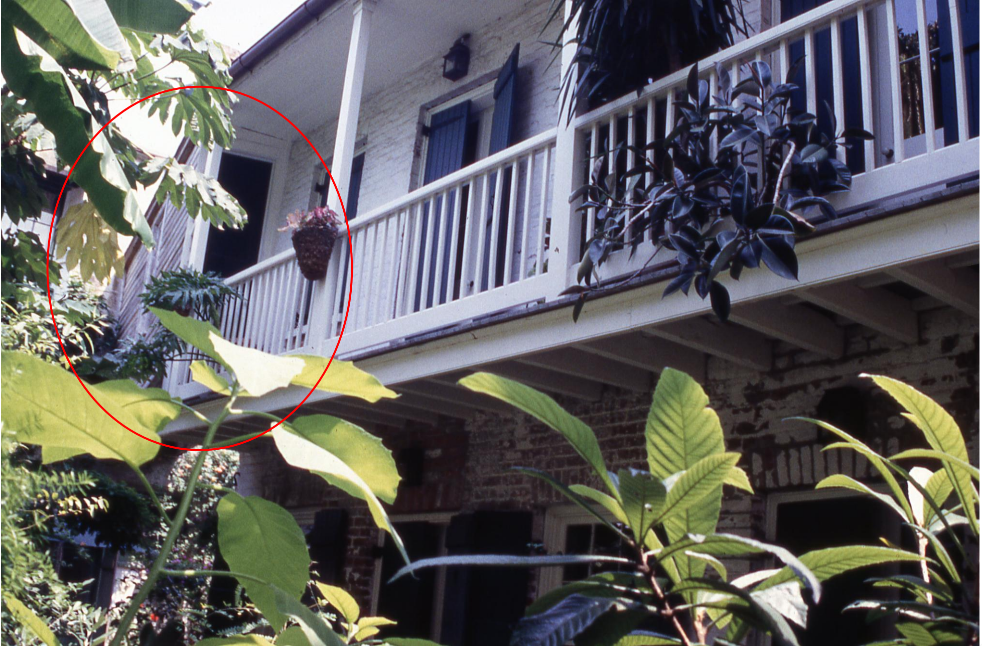
1028 Bourbon, Linking Structure, 1998
