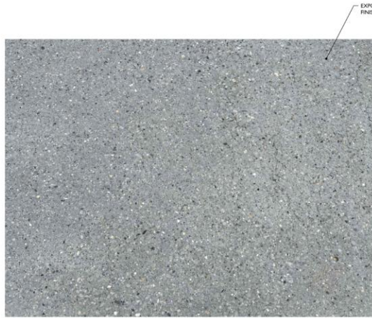
EXPOSED AGGREGATE PAVEMENT FINISH REFERENCE PHOTO. SEE CIVIL FOR DETAILING.
