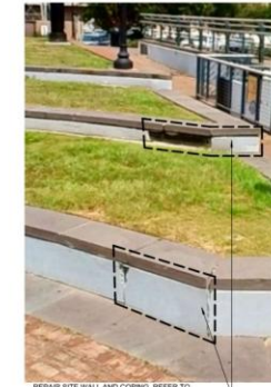
12 EXISTING SITE WALL TO REPAIR 8 12" x 1'-0"
