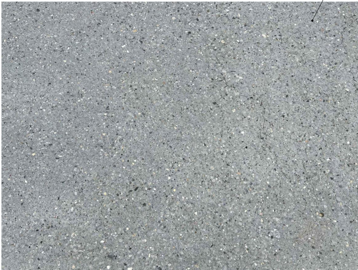
EXPOSED AGGREGATE PAVEMENT FINISH REFERENCE PHOTO, SEE CIVIL FOR DETAILING.
