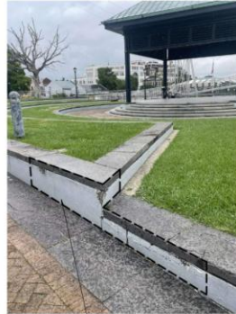
09 EXISTING SITE WALL TO REPAIR 5 12" x 1'-0"
