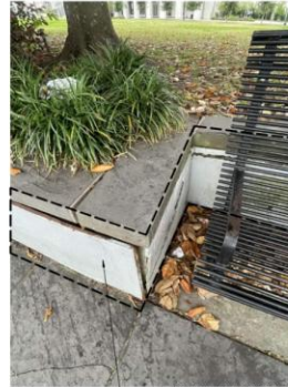
06 EXISTING SITE WALL TO REPAIR 3 77" x 12" x 1'-0"
