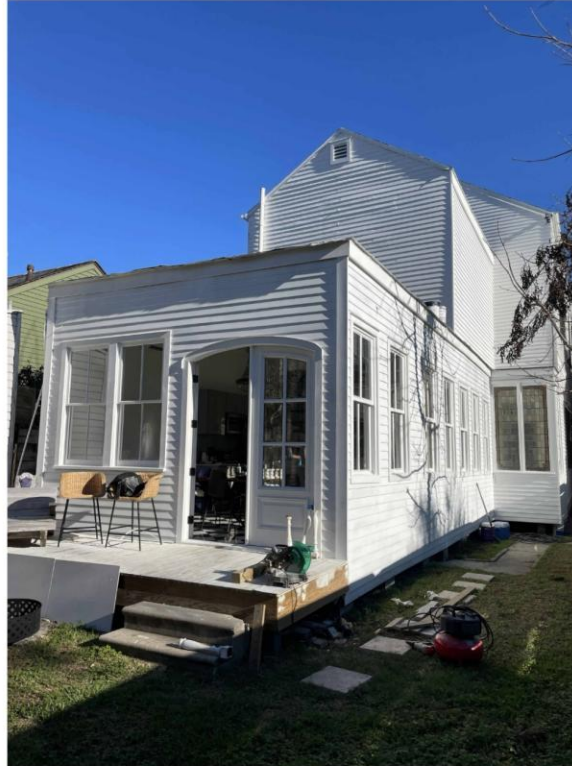
PHOTO B (EXISTING REAR ADDITION)
