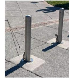
8 EXISTING STAINLESS STEEL REMOVABLE BOLLARD 1'-0" x 1'-0"
