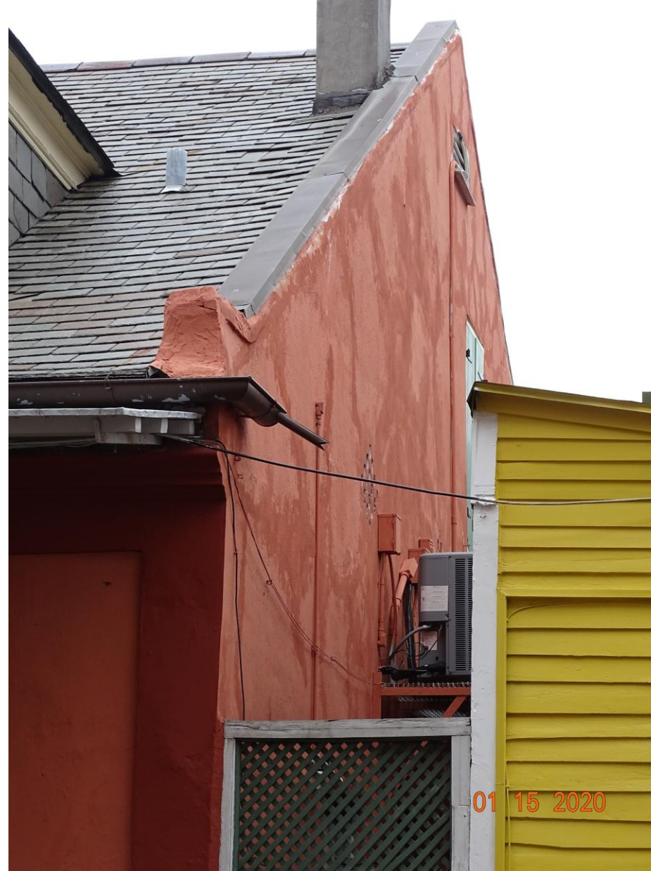
923-29 Dauphine (photo of 831 Dauphine after partial metal cap removal)
