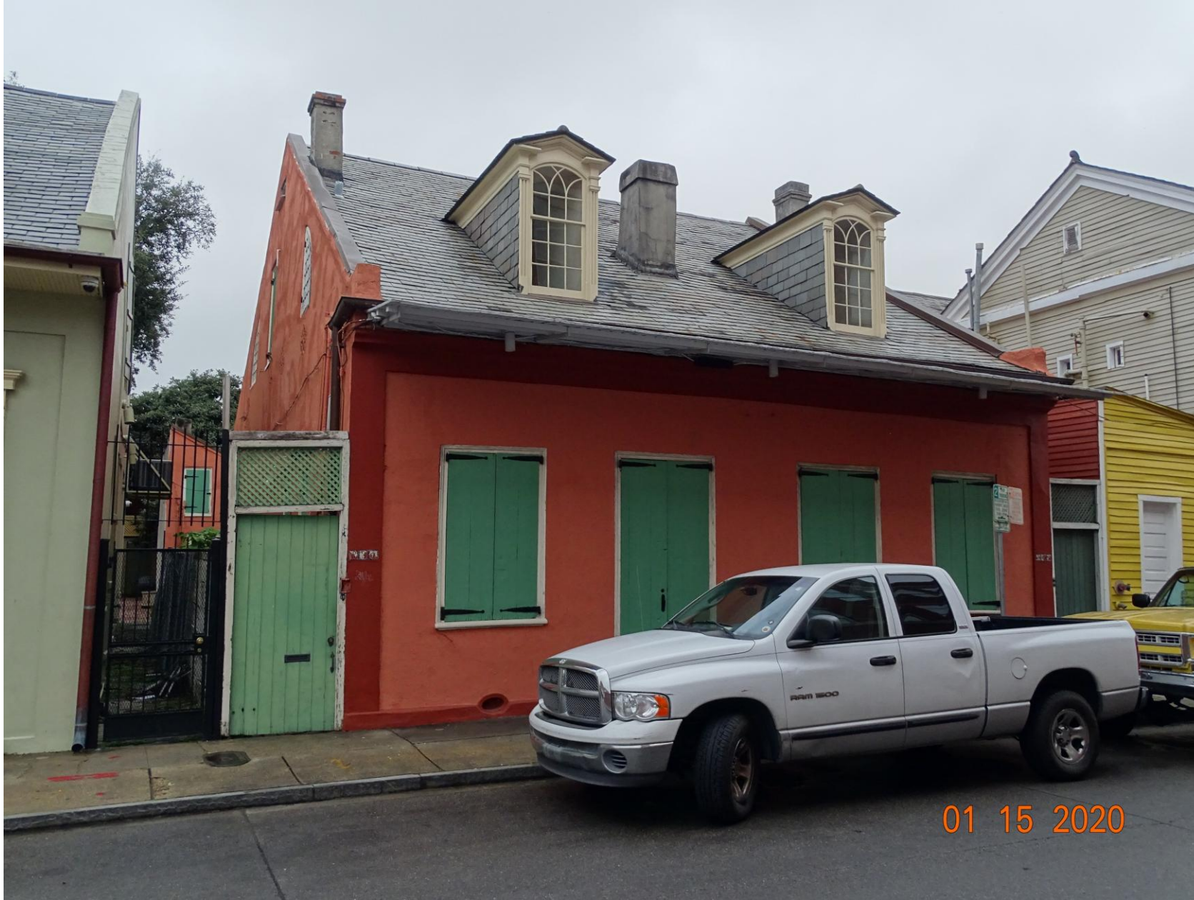
923-29 Dauphine (photo of 831 Dauphine after partial metal cap removal)
