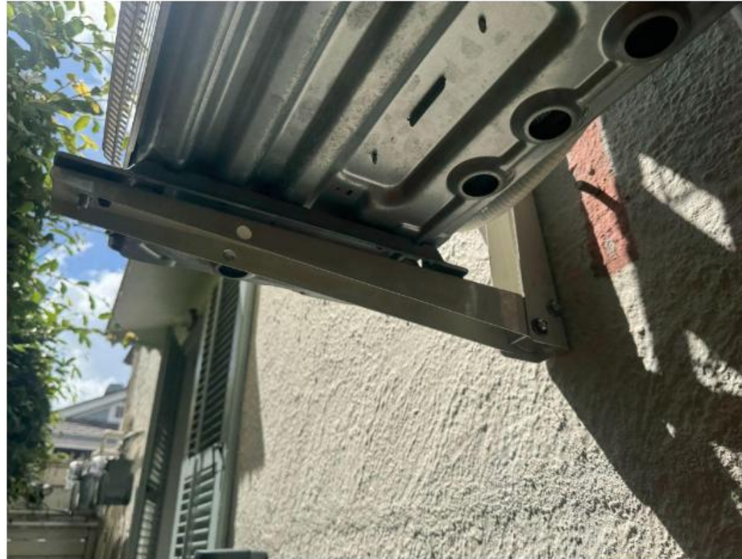
No wall distress present after nearly 10 years of service
