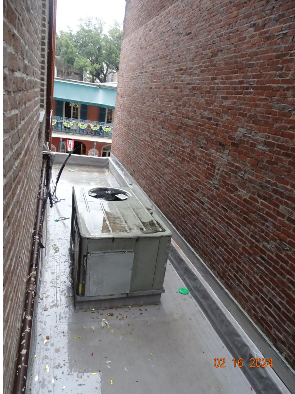
429-433 Bourbon – Roof of one-story portion VCC Architectural Committee
