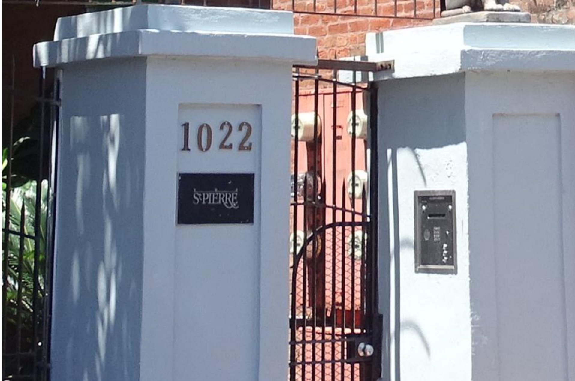
1022 St. Peter – Previously Existing Intercom
