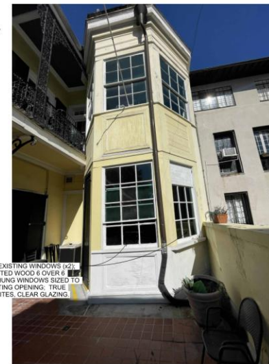
PHOTO OF CURRENT CONDITIONS @ REAR MAIN BUILDING
