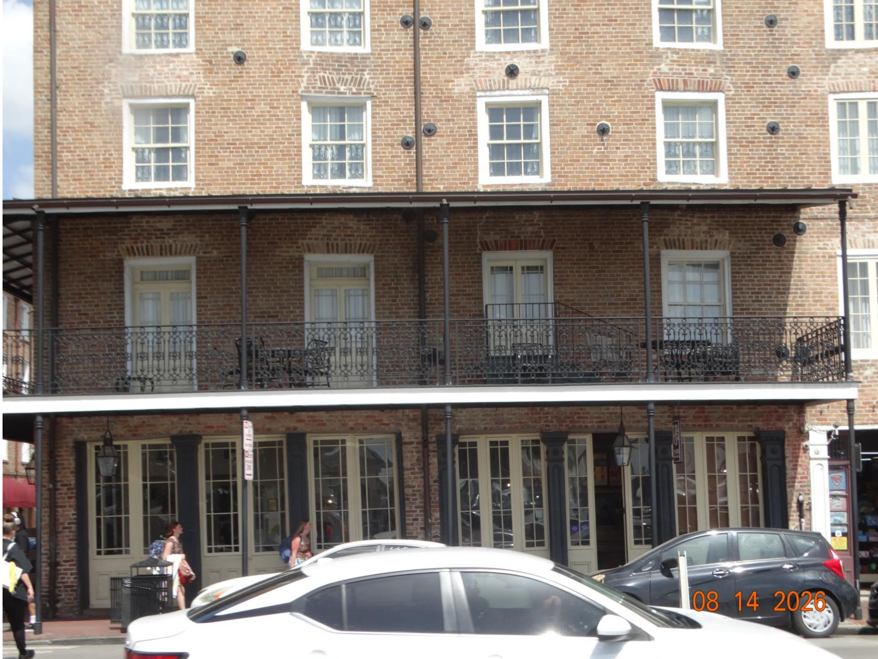
501, 503-05 Decatur VCC Architectural Committee
