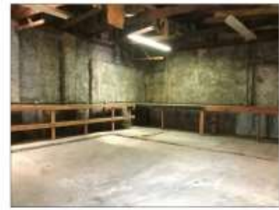
7 EXISTING INTERIOR VIEW REAR STORAGE AREA
