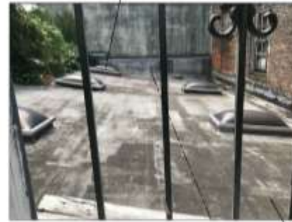
4 EXISTING REAR ROOF
