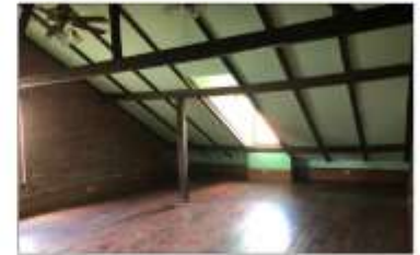
9 EXISTING INTERIOR VIEW 3rd FLOOR
