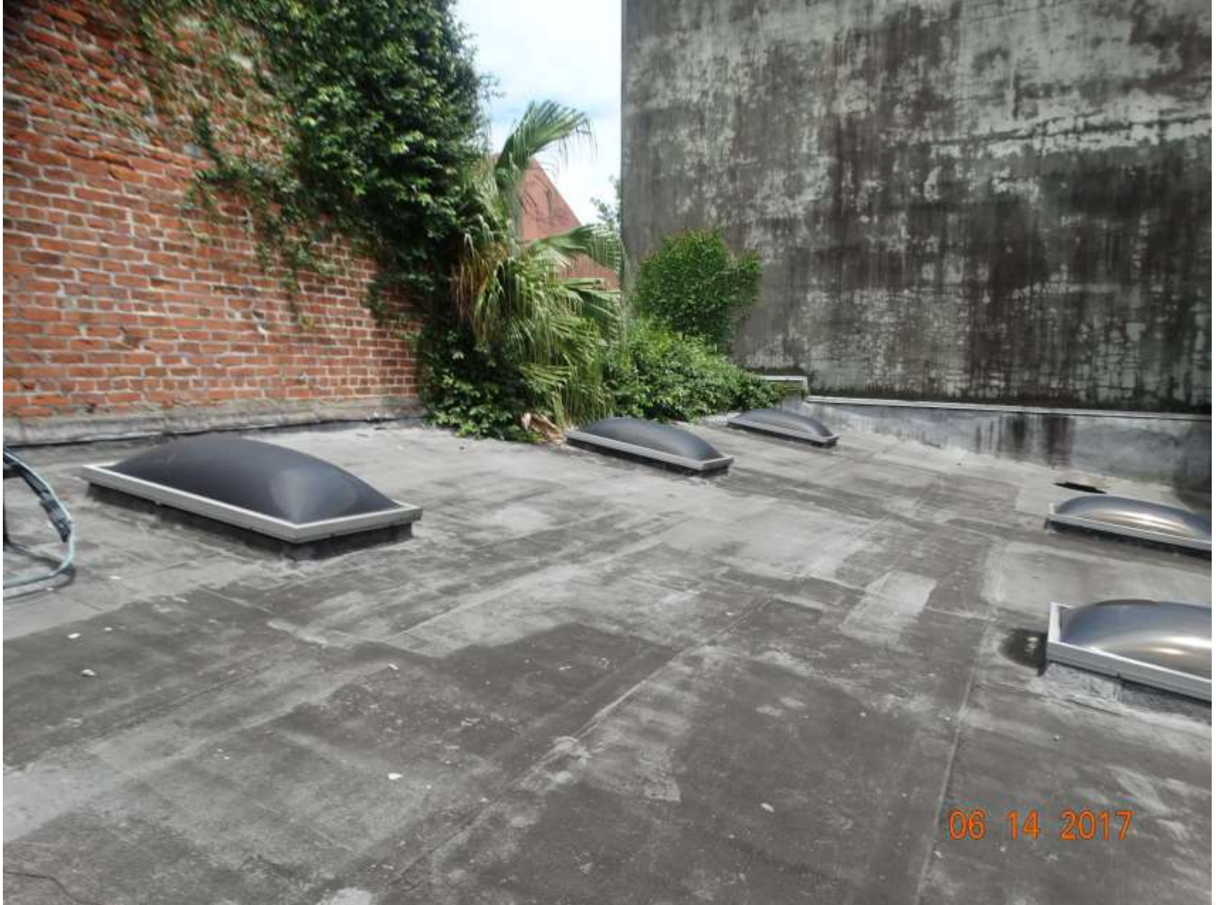
622 N Rampart – existing brown-rated roof
