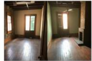
8 EXISTING BEDROOMS VIEW 2nd FLOOR
