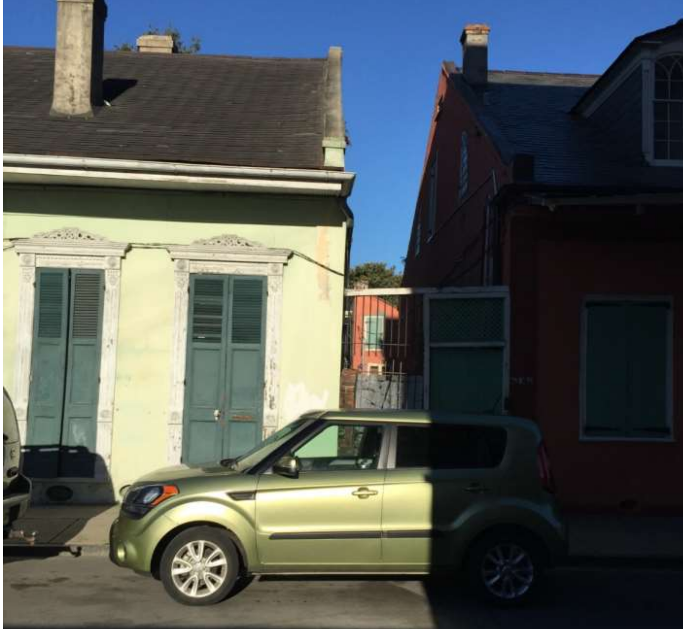
823 Dauphine – before renovation
