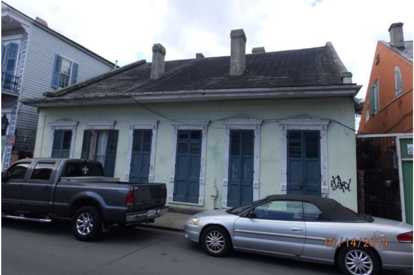
823 Dauphine – before renovation
