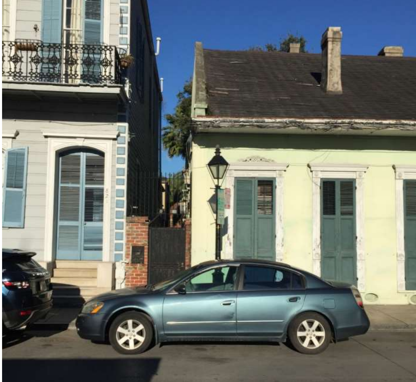
823 Dauphine - – before renovation
