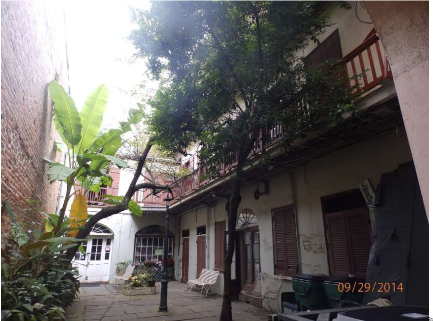
622-624 Royal, existing courtyard
