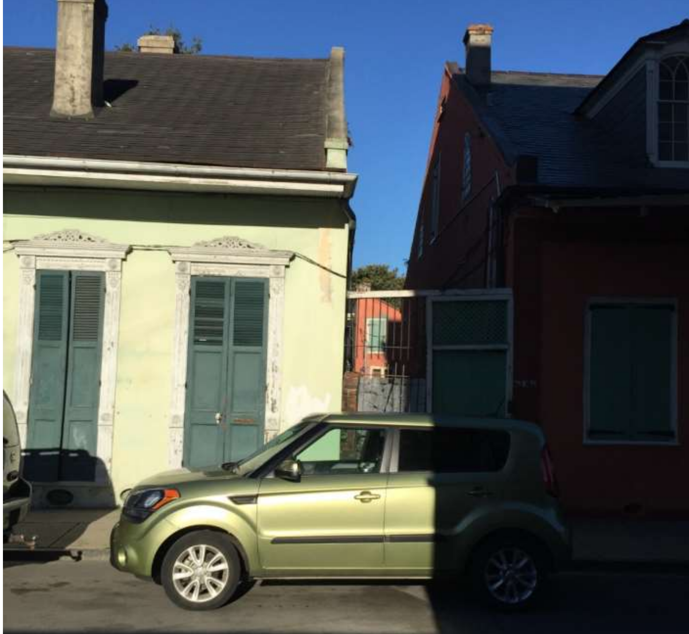
823 Dauphine – before renovation
