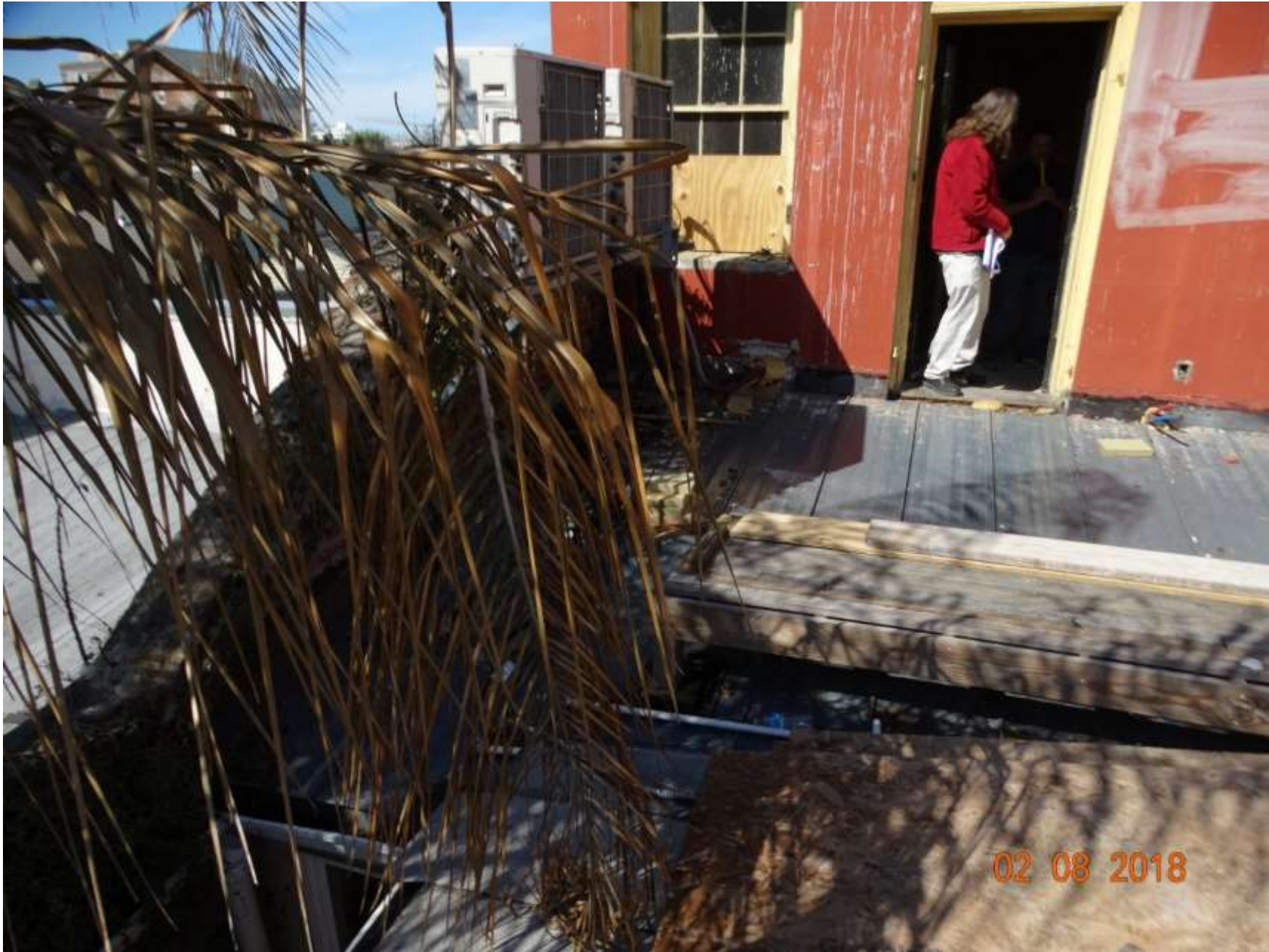
828 Toulouse – 828 rear building – Above Courtyard Infill space
