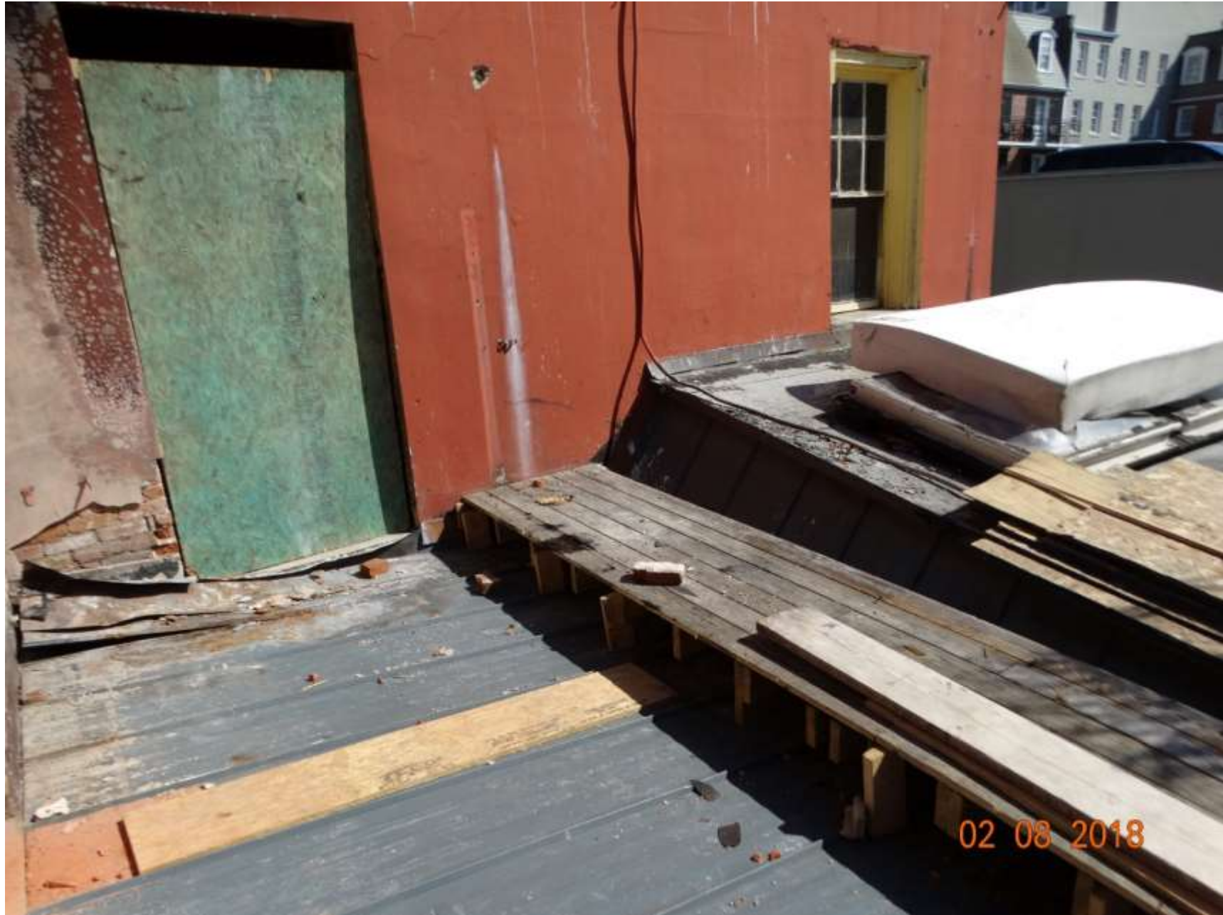
828 Toulouse – 828 rear building – Above Courtyard Infill space
