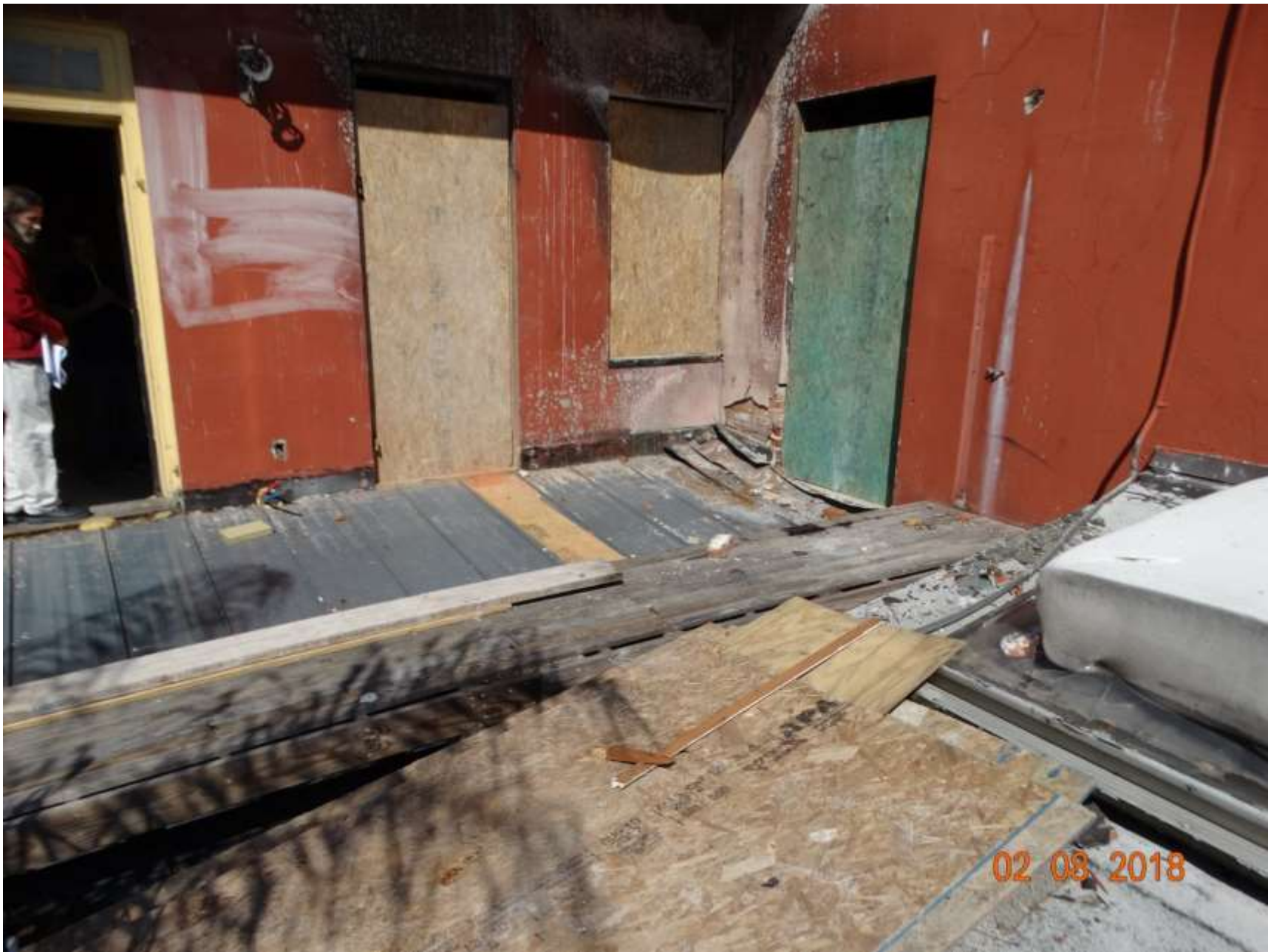
828 Toulouse – 828 rear building – Above Courtyard Infill space
