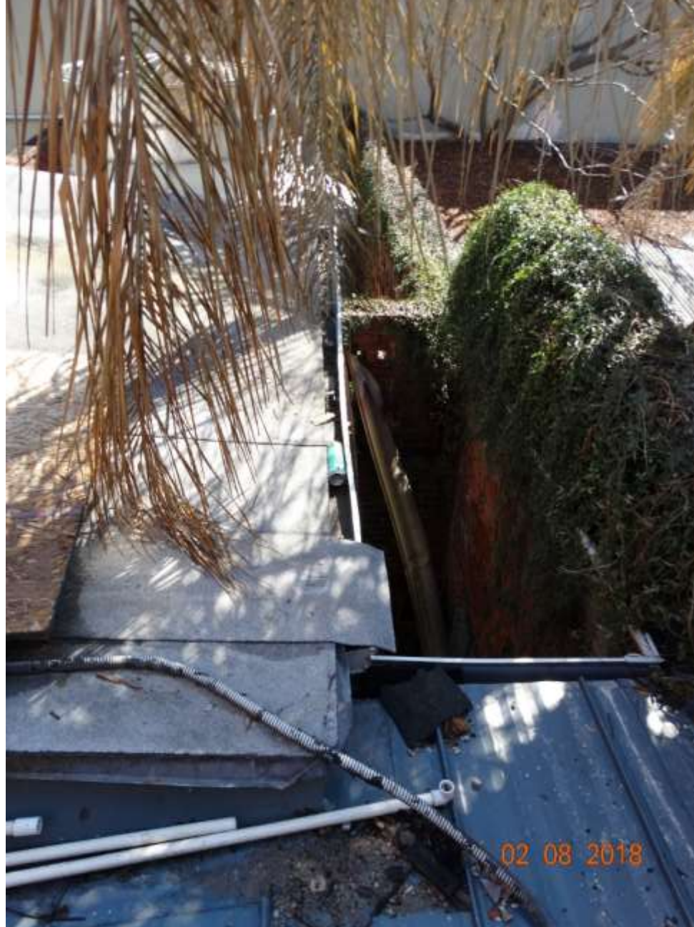
828 Toulouse – 828 rear building – Above Courtyard Infill space
