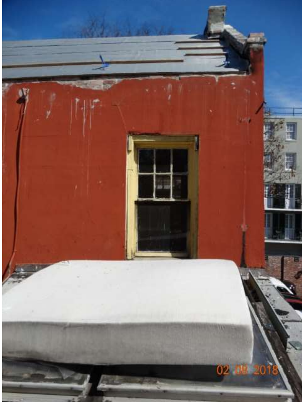
828 Toulouse – 828 rear building – Above Courtyard Infill space
