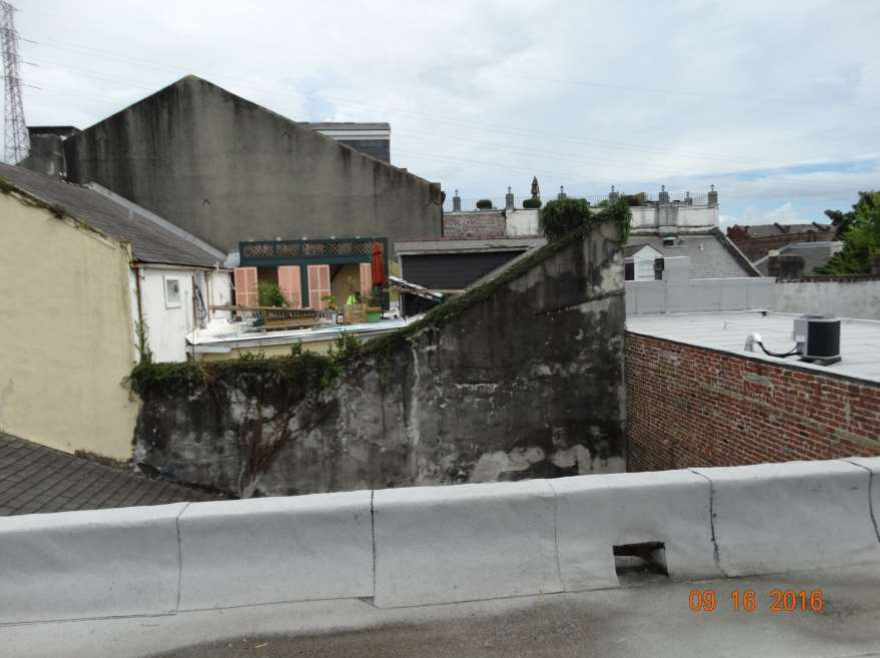
Rooftop Subcommittee Draft Resolution presentation – Examples of activated exterior rooftop additions
