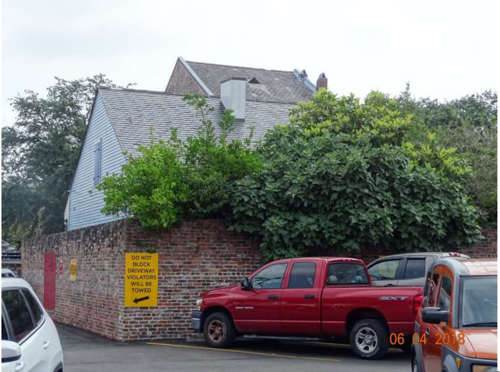
1026 St. Louis – Rear from Parking Lot
