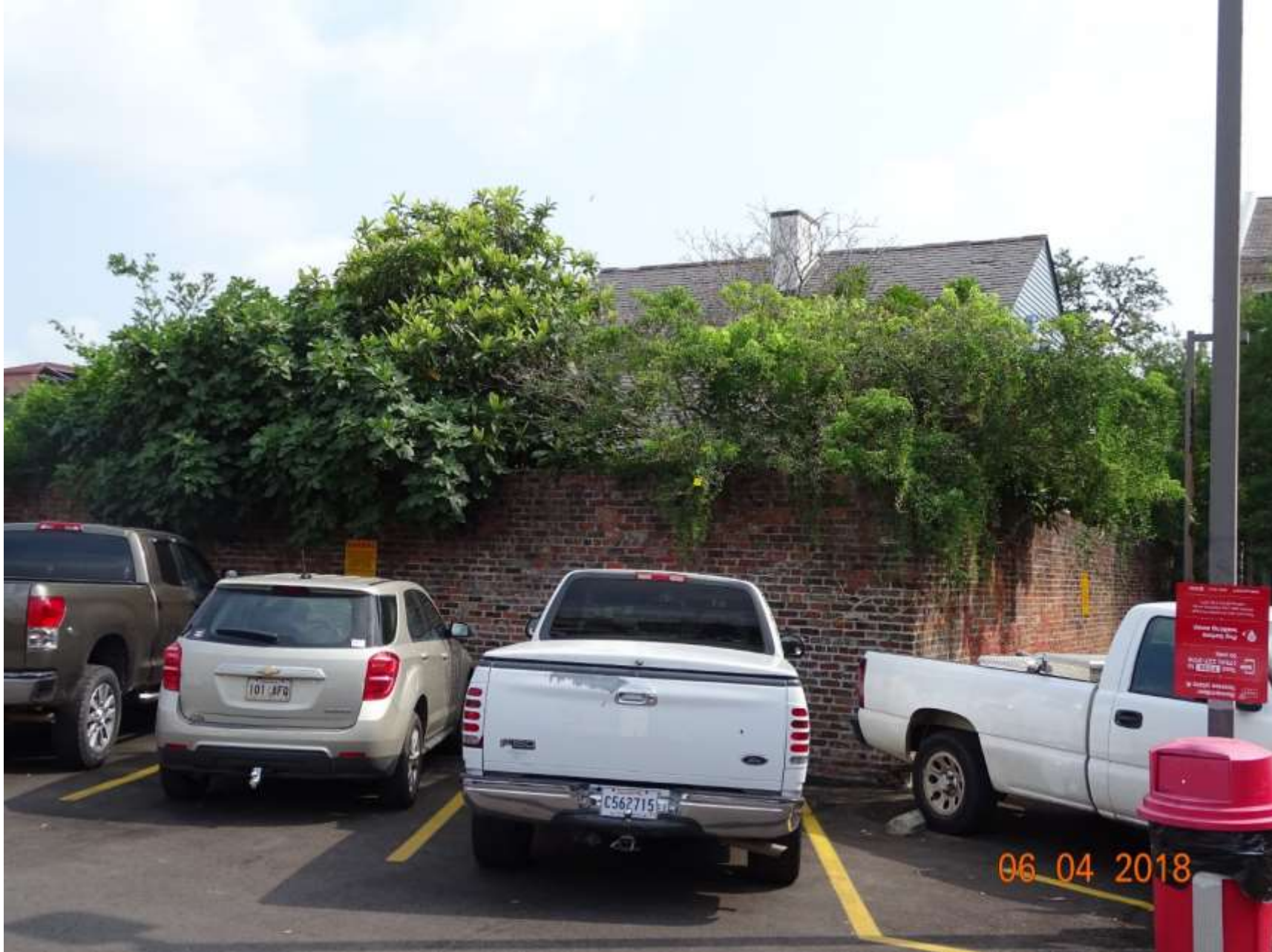
1026 St. Louis – Rear from Parking Lot
