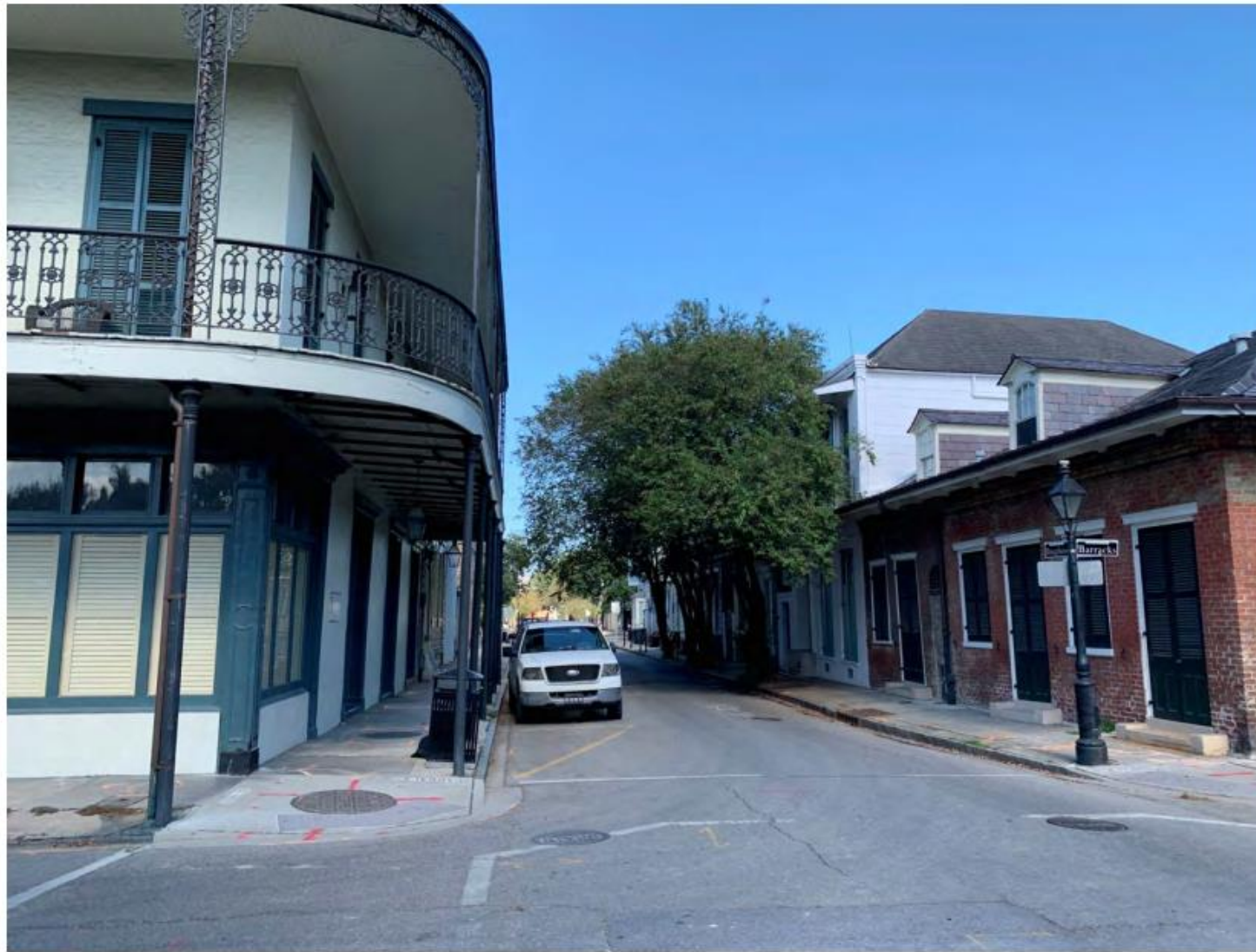
12' EXISTING LAMP POST
