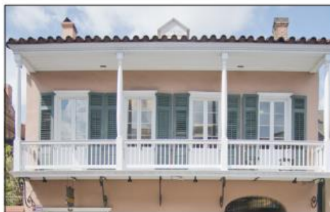
A Creole home, such as this townhouse, often has a simple balustrade and convex bulging posts.
