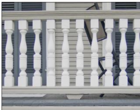
A turned wood balustrade, produced by turning and carving square balusters on a lathe, are appropriate for most Italianate, Queen Anne, Eastlake, Classical Revival and Colonial Revival homes. Historic balusters tend to be wider than many new, mass-produced balusters.
