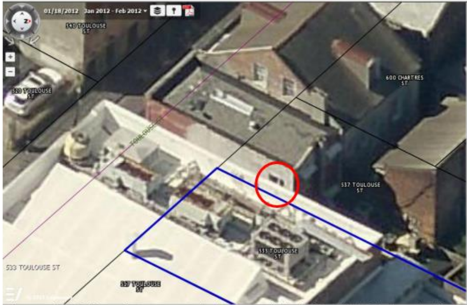
January 18, 2012 – prior to current decking material being installed. The door leading onto the roof is in place.
