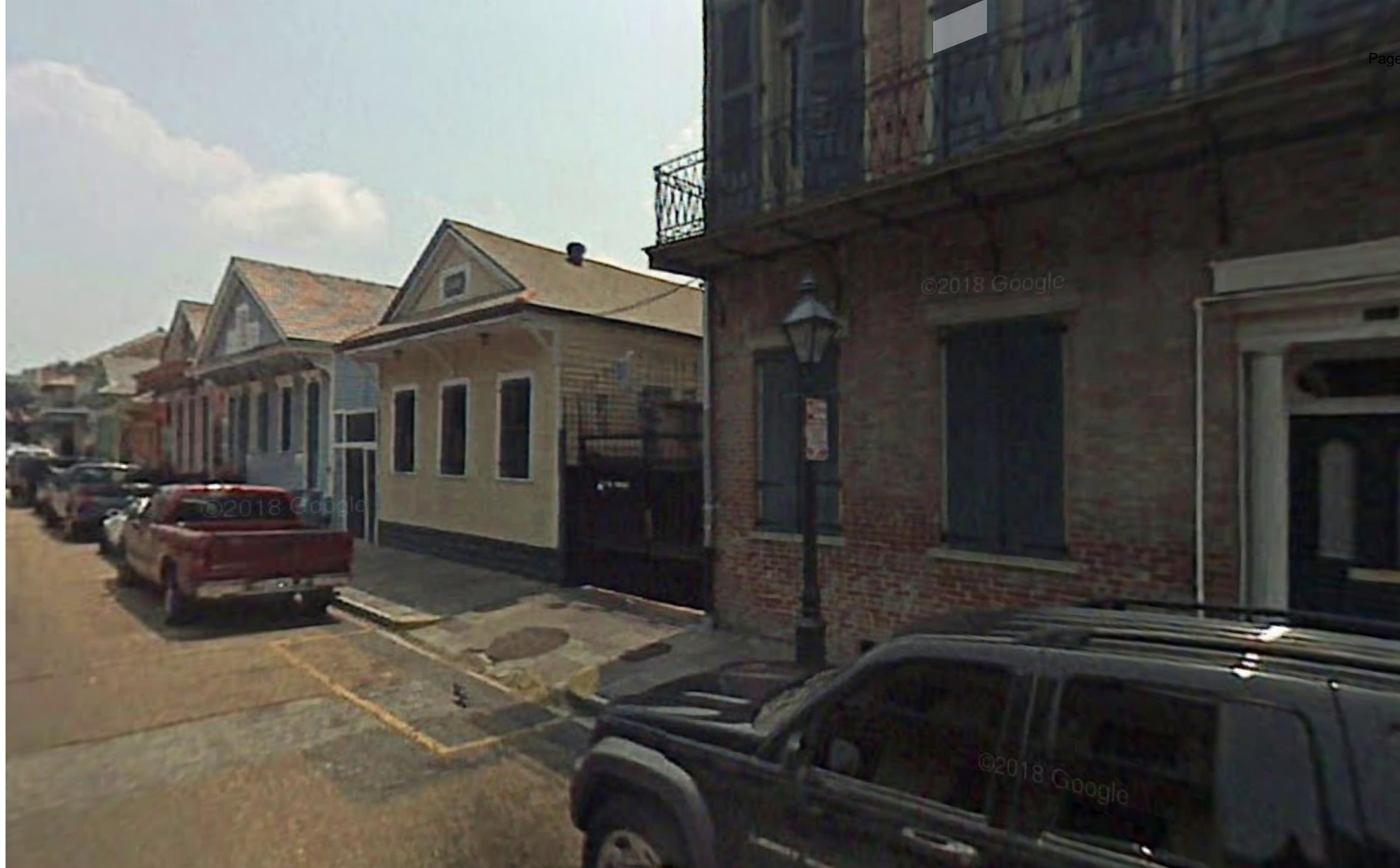
922 St Ann – 2007, prior to wall collapse
