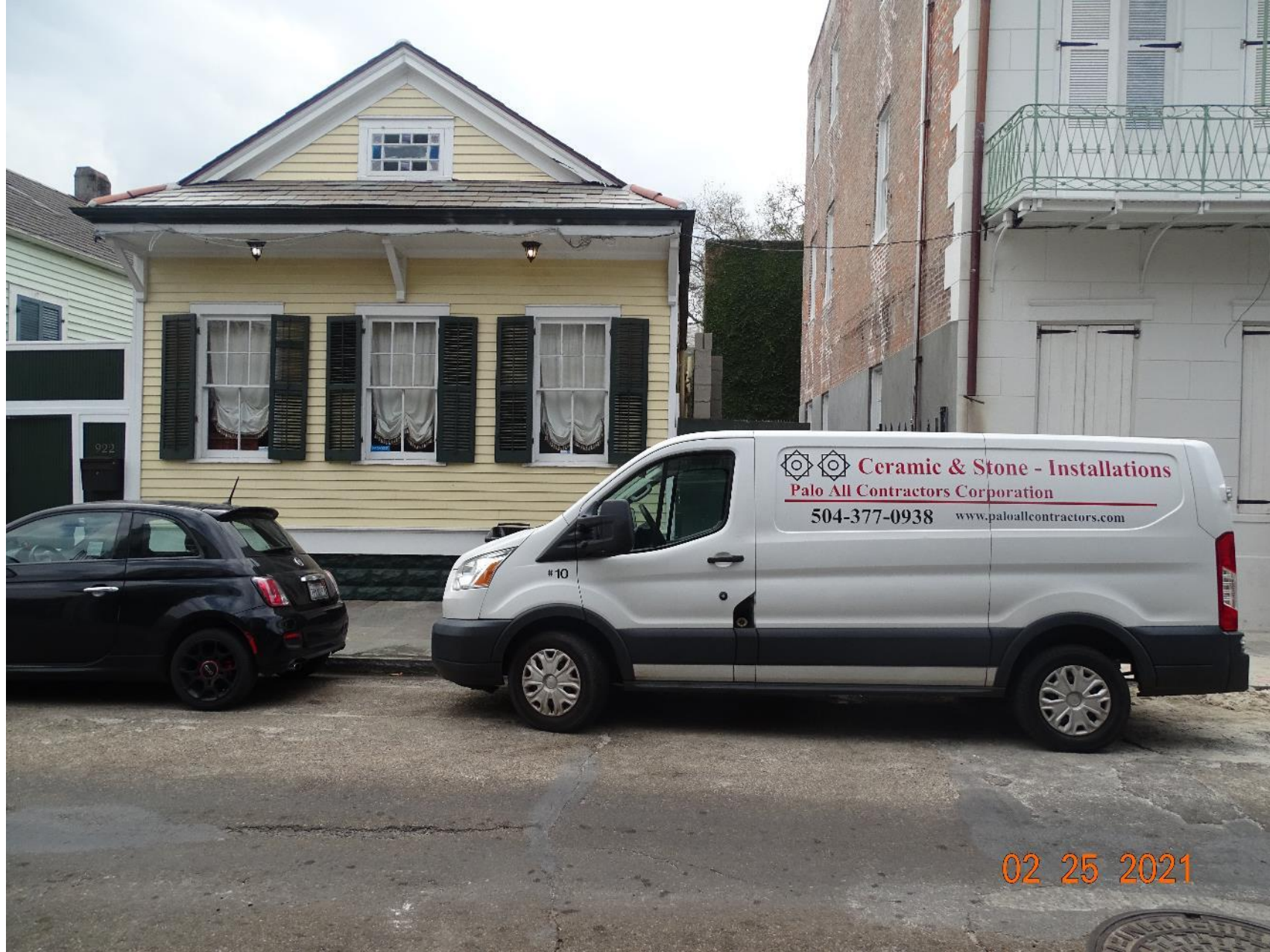
928 St. Ann – 2/25/2021, STOP WORK ORDER PLACED
