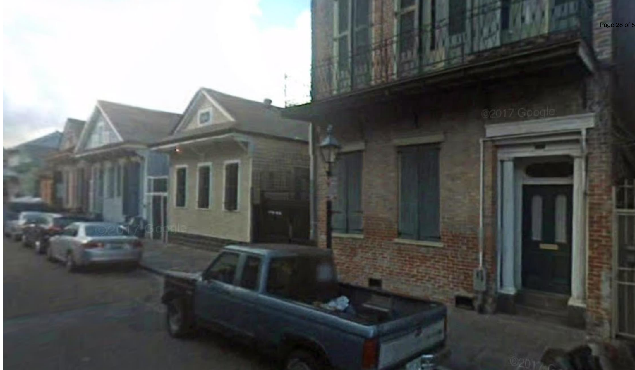
922 St Ann – 2008, prior to wall collapse
