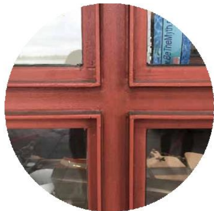
EXISTING PAINTED STEEL
