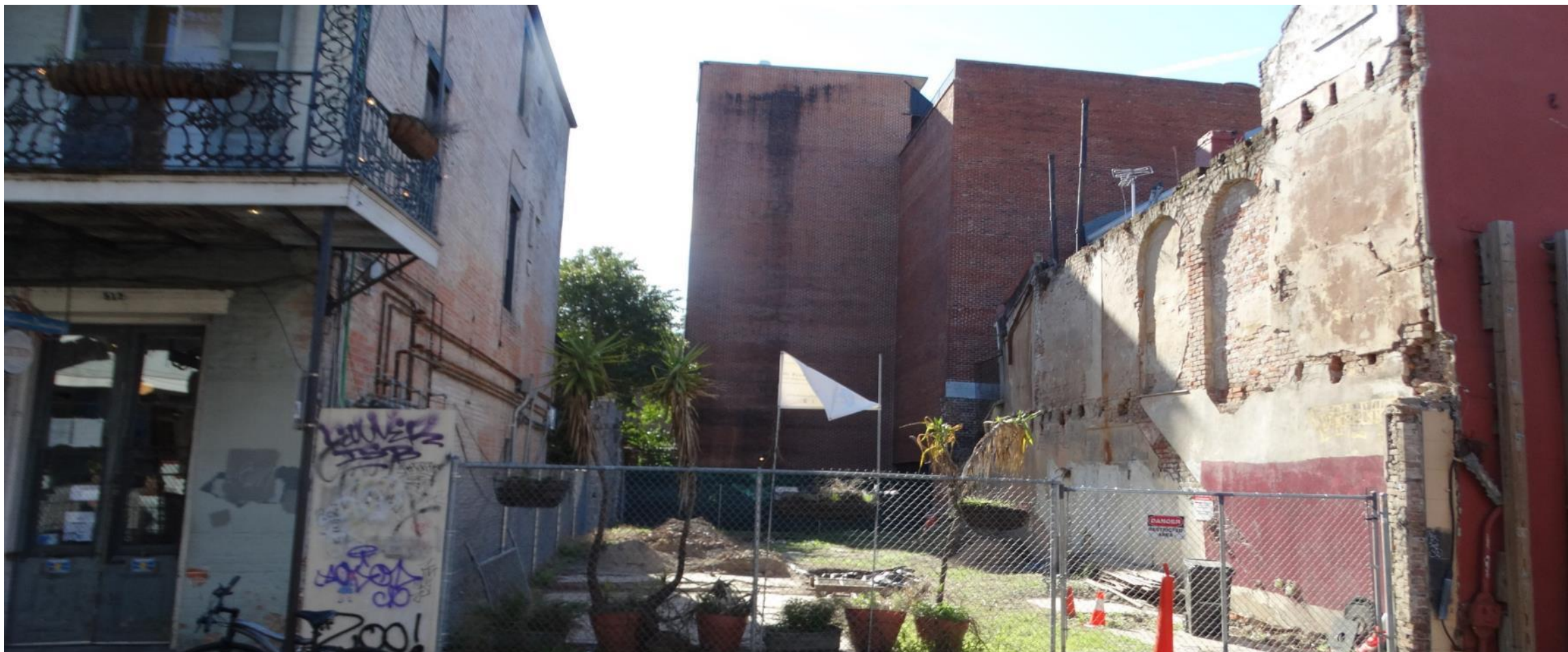
808 Royal – Existing Conditions
