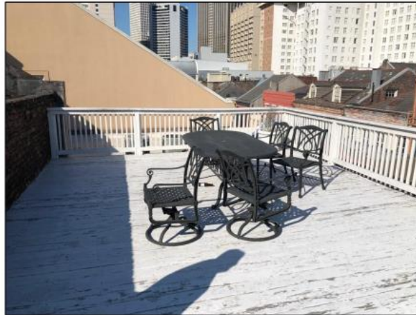
Above view of balcony structure
