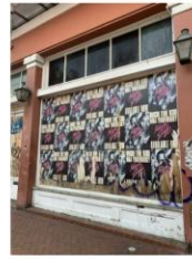
EXISTING STOREFRONT WINDOWS
