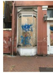
EXISTING STOREFRONT WINDOWS
