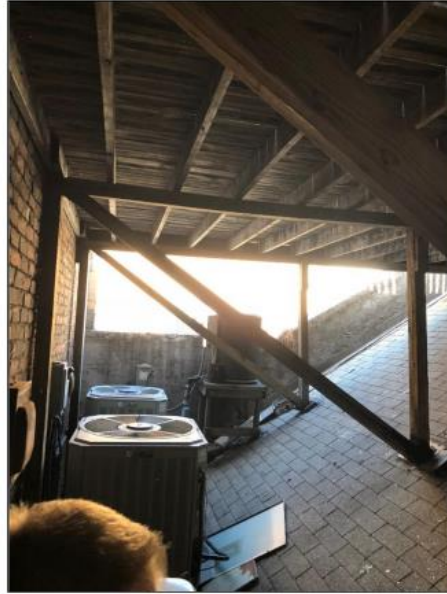
Underneath view of balcony structure
