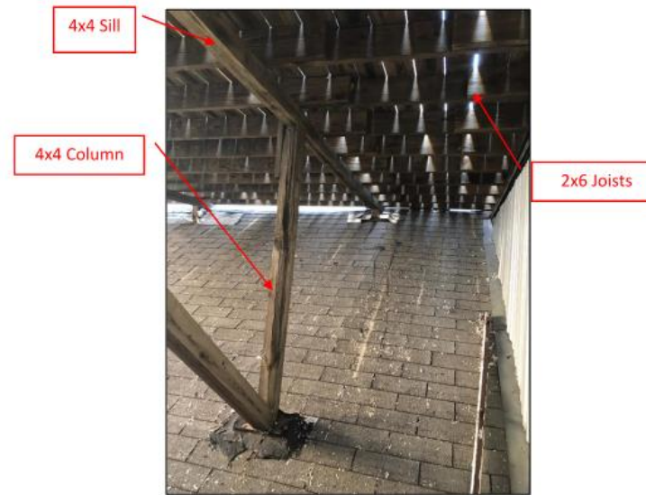
Balcony Structure – Framing Sizes Noted
