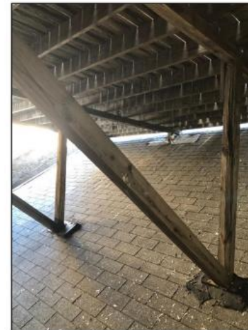
Balcony Structure – Column/Sill Spacing at 8 ft
