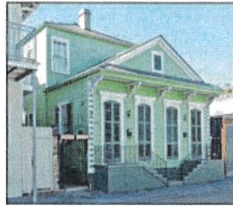
A camelback addition typically is found on a wood-framed shotgun single or double.
