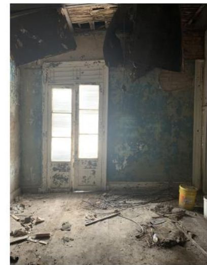
INTERIOR SETTLING LEVEL 3
