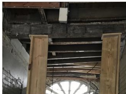
CARRIAGE WAY SETTLING
