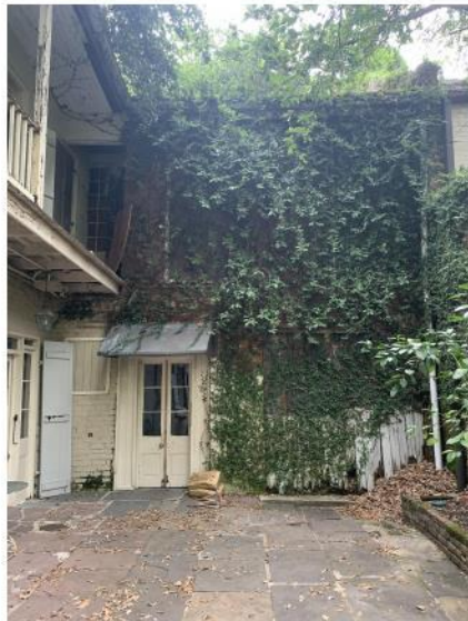
REAR WALL PRIOR TO VINE REMOVAL
