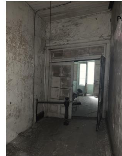
INTERIOR SETTLING LEVEL 2 #3
