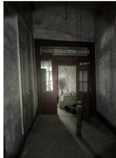
INTERIOR SETTLING LEVEL 2 #1
