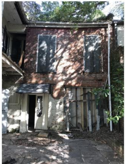
REAR WALL AFTER VINE REMOVAL
