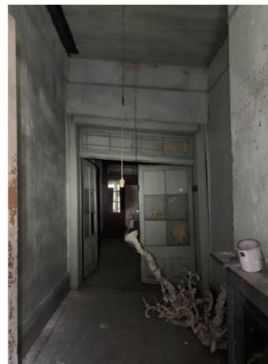
INTERIOR SETTLING LEVEL 2 #2
