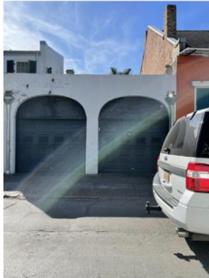
PHOTOGRAPH OF EXISTING GARAGE DOORS
