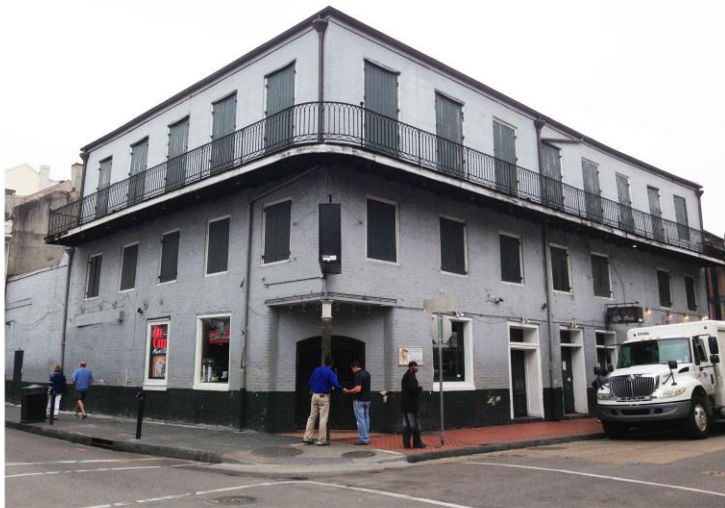
CORNER VIEW - EXISTING
