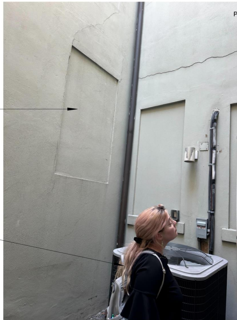
EXISTING CONDITION - IMAGE 2
