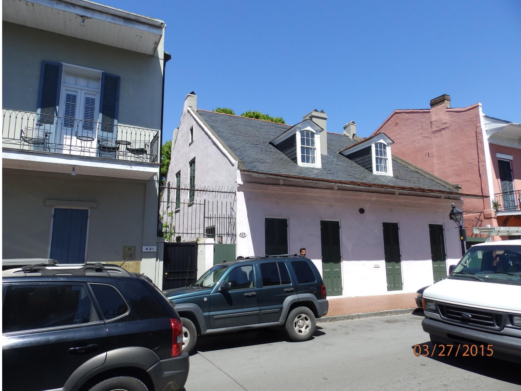
625 Dauphine, 2015 – Prior to Unpermitted Decorative Fixture Installation
