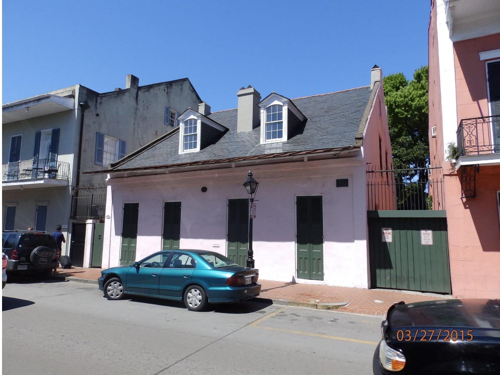
625 Dauphine, 2015 – Prior to Unpermitted Decorative Fixture Installation
