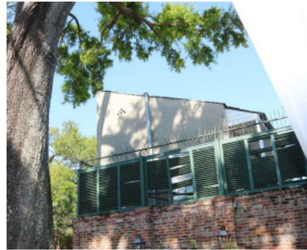
Figure 2 - damaged fencing and hedgehog
