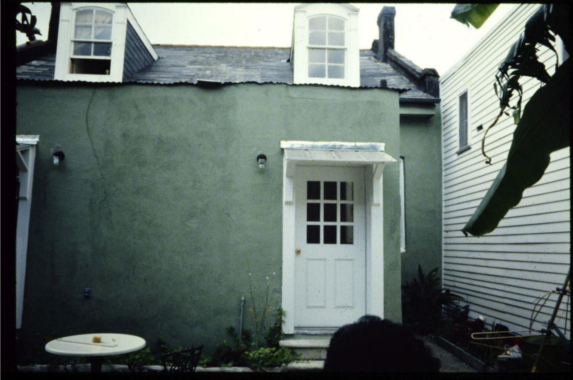
1238 Dauphine – previously existing, narrower dormers
