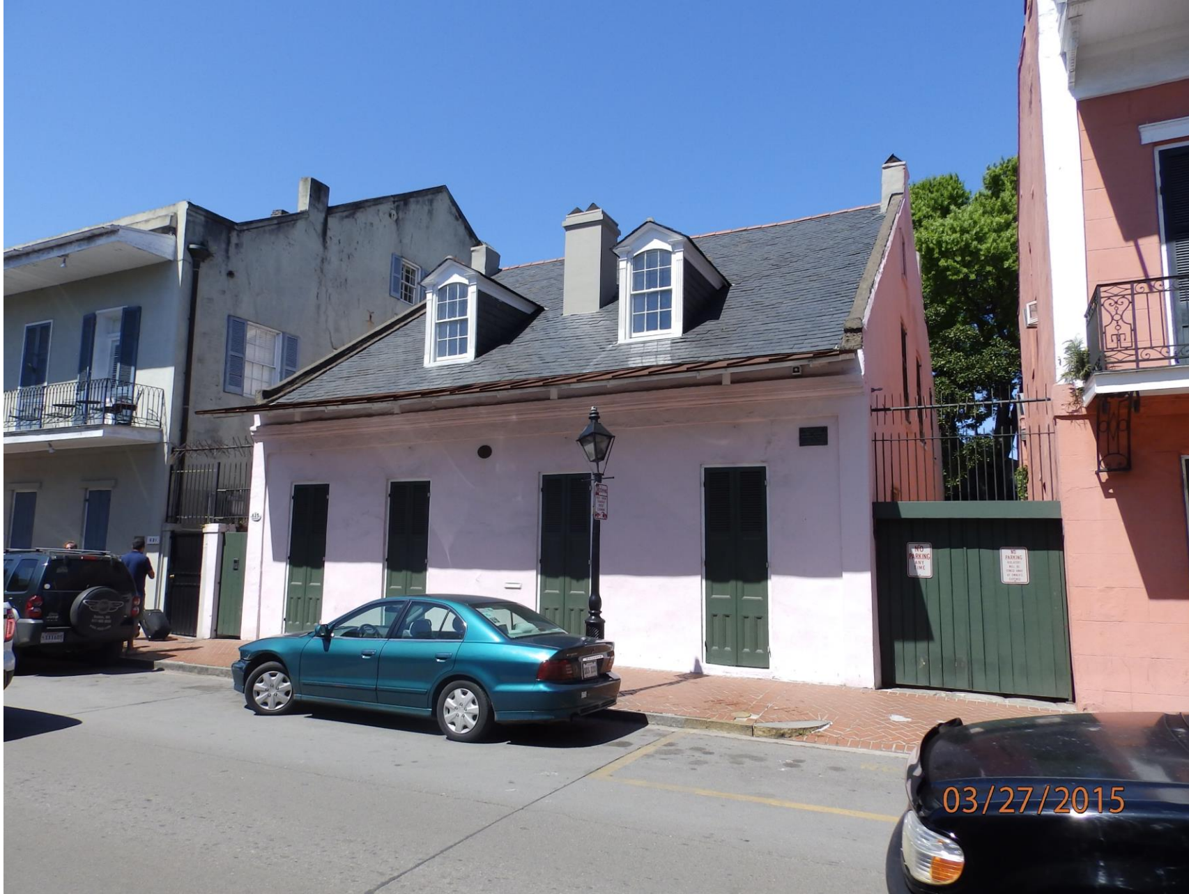
625 Dauphine, 2015 – Prior to Unpermitted Decorative Fixture Installation
