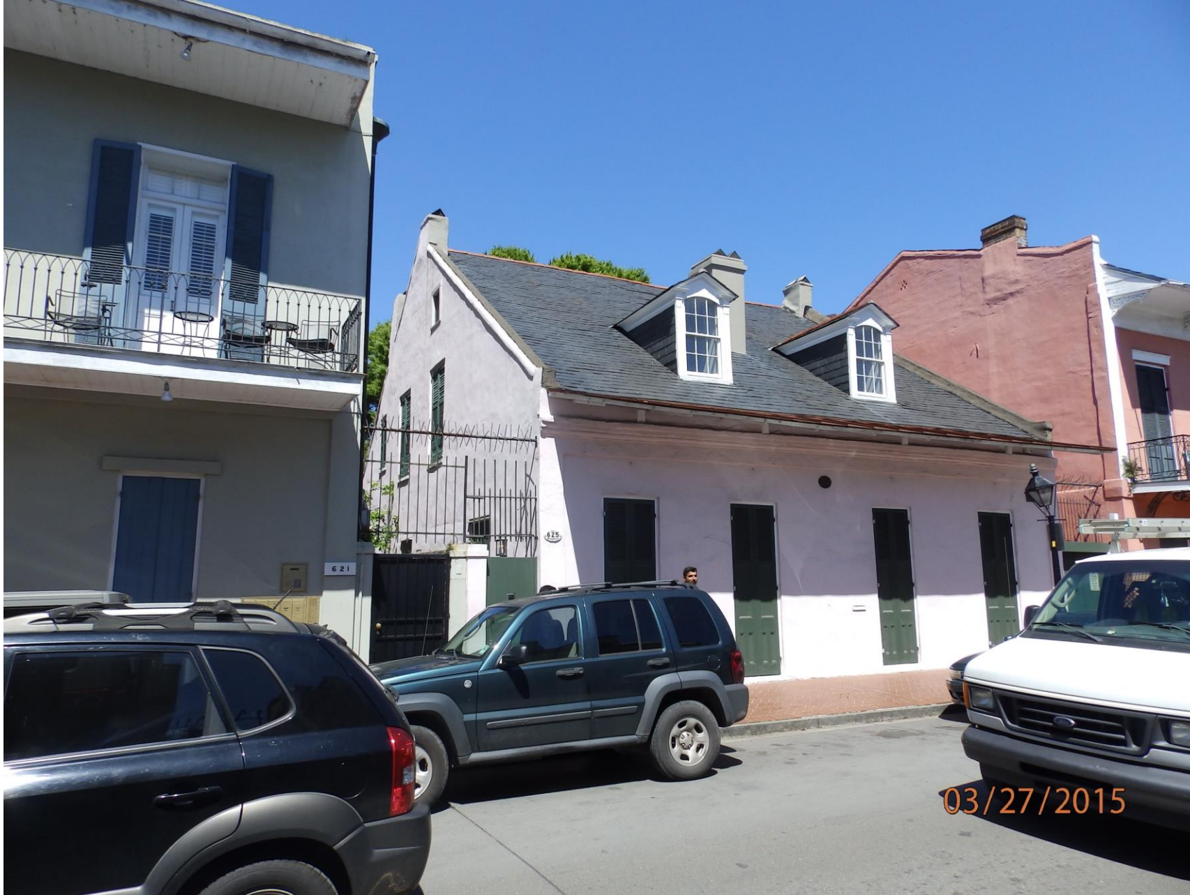
625 Dauphine, 2015 – Prior to Unpermitted Decorative Fixture Installation
