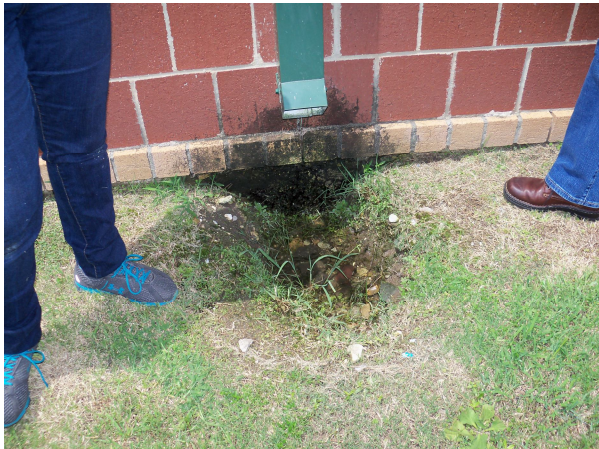
Figure 7. Most downspouts had eroded soil and water accumulated created mosquito breeding areas at Henry Schaumburg. All the holes were filled with sand and covered with a concrete paver to prevent erosion.
