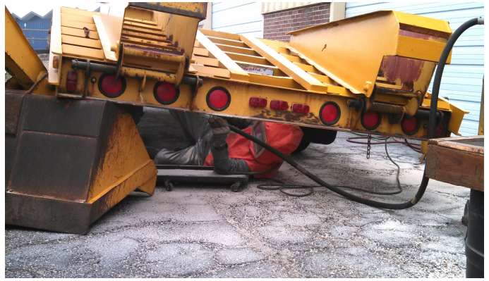
Figure 23. Brooks Hartman wearing protective equipment while sandblasting the undercarriage of the backhoe trailer.
