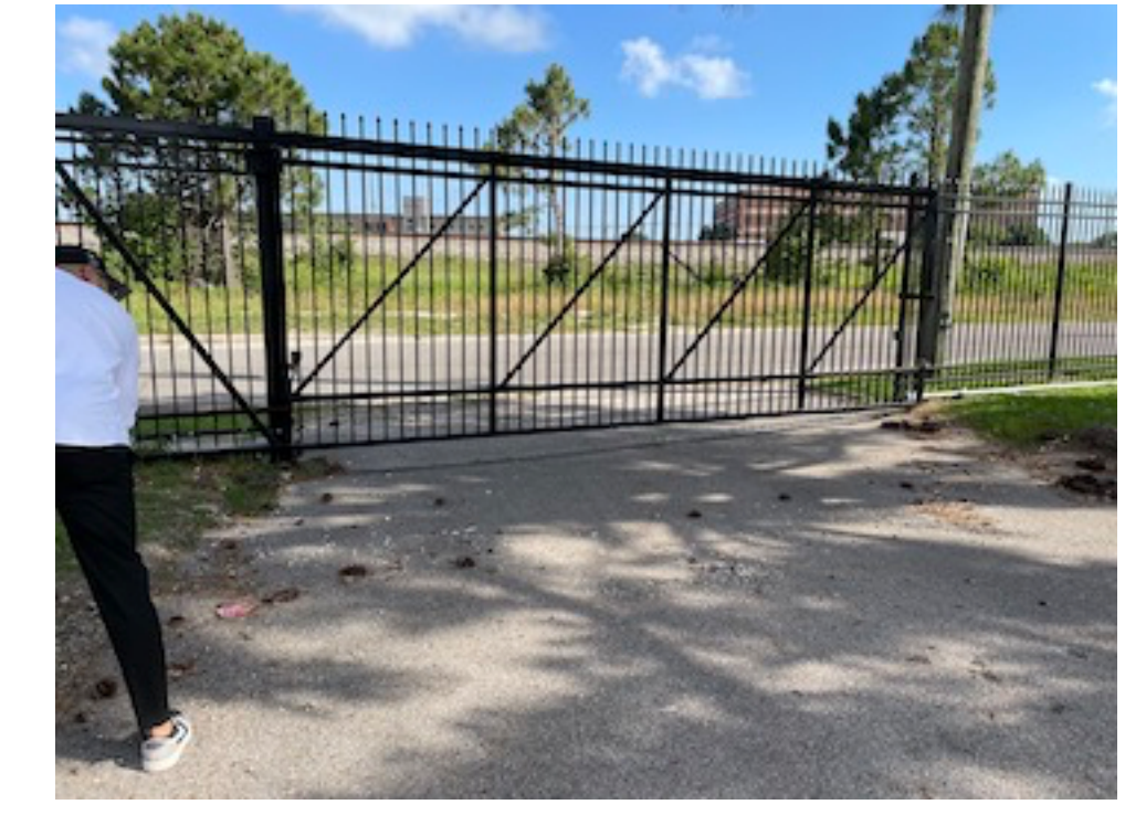
VIEW NORTHEAST GATE
