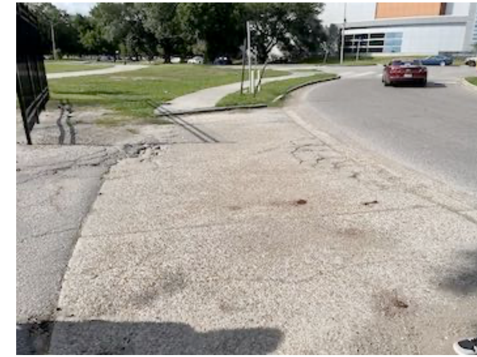
VIEW SOUTHWEST GATE DRIVEWAY APRON
