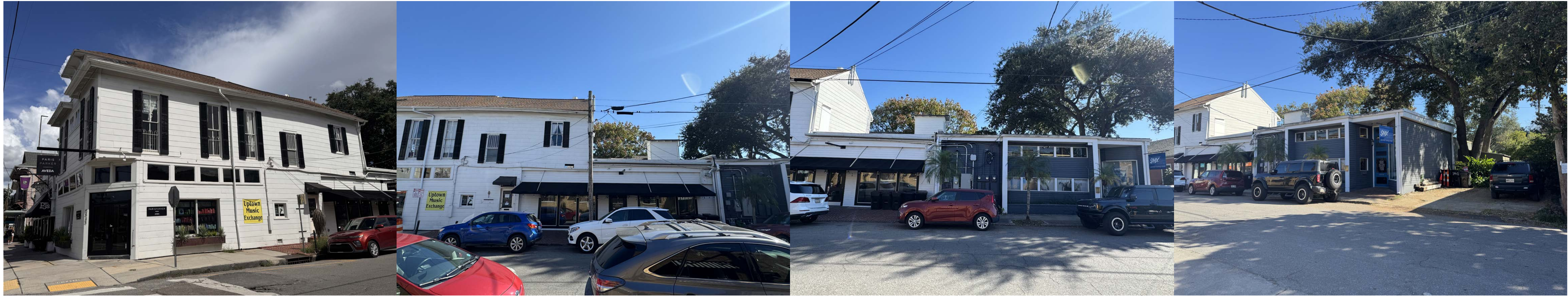
OCTAVIA STREET SIDE - EXISTING PHOTOS
