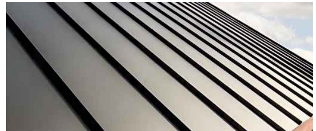
Standing Seam Metal Panel Roof
