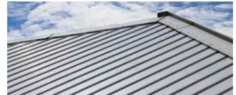
Standing Seam Metal Panel Roof
