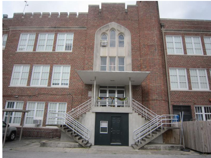
6325 CROMWELL PLACE- HOLY NAME OF JESUS EXISTING BUILDING
