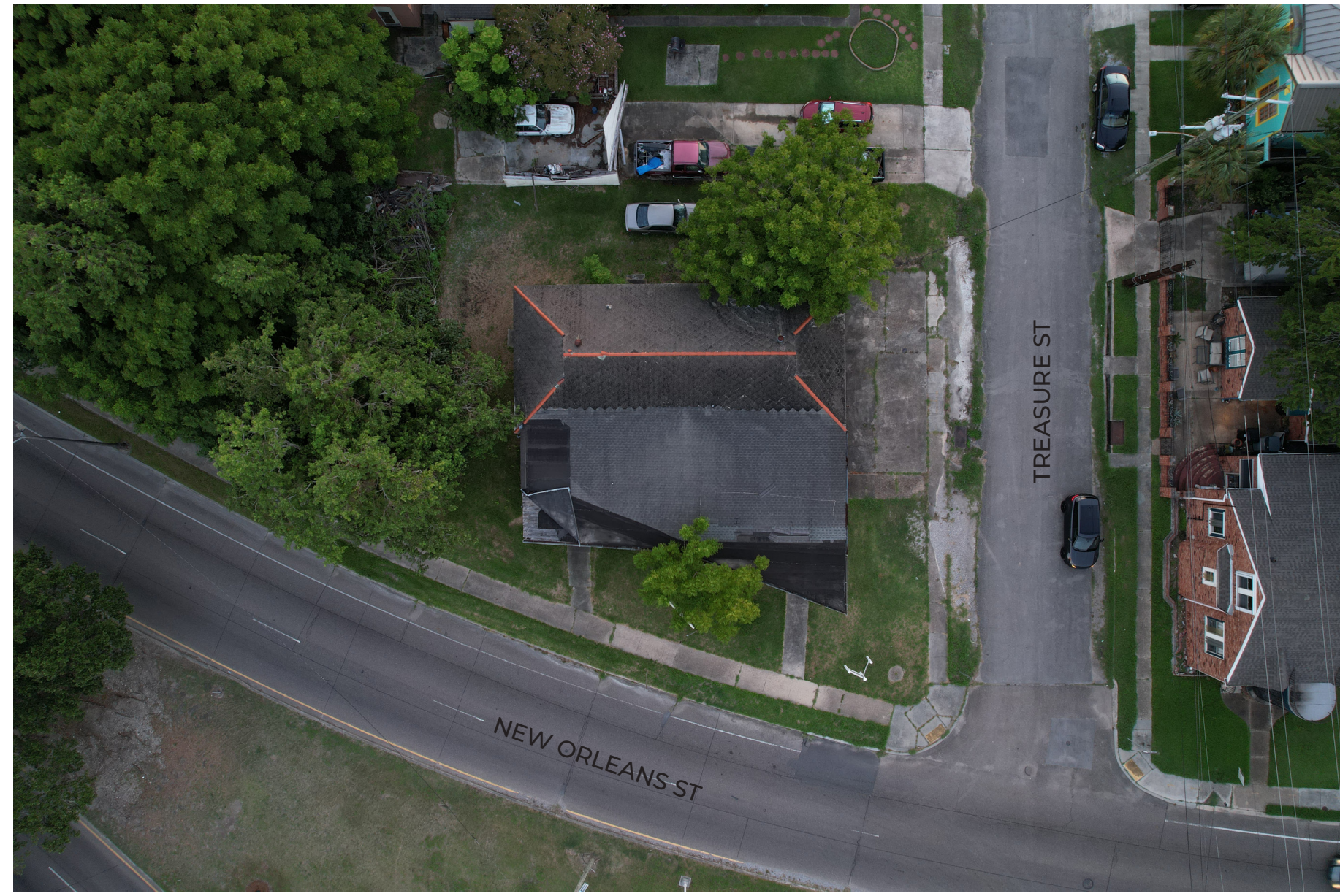
2 SITE PHOTO - AERIAL OF EXISTING CONDITIONS, NEW ORLEANS ST NTS
