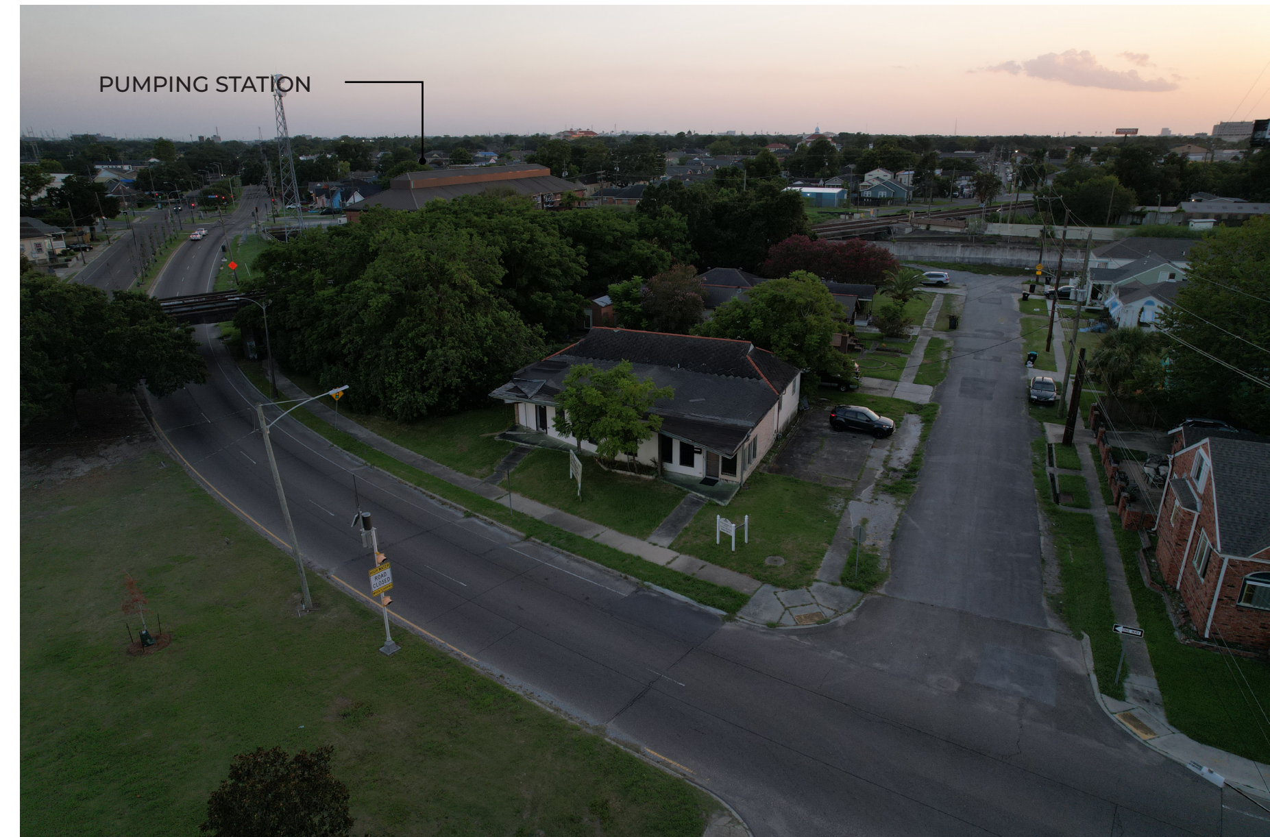
6 SITE PHOTO - AERIAL TOWARDS SW (VIEW TOWARDS PUMPING STATION) NTS
