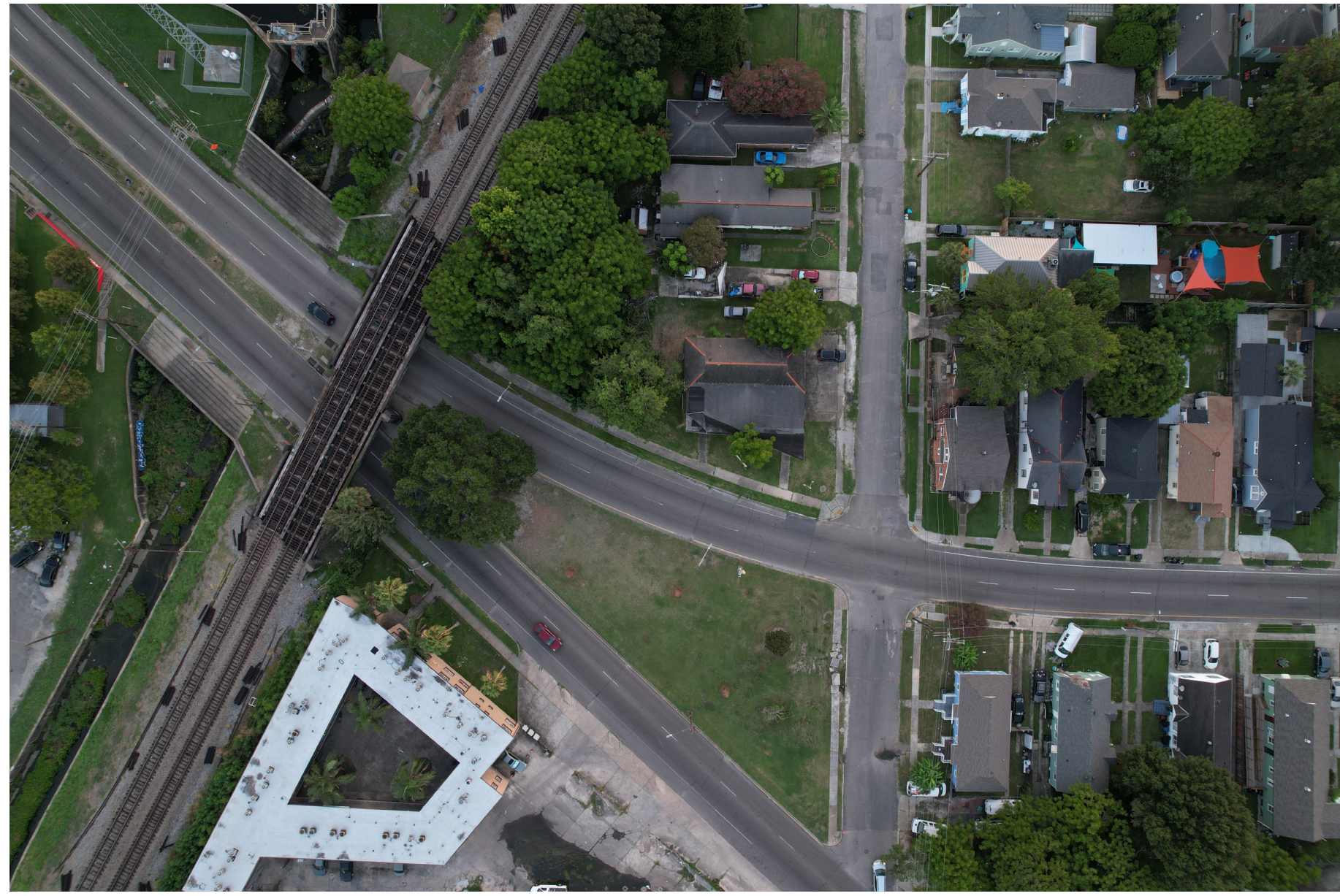
1 SITE PHOTO - AERIAL OF EXISTING CONDITIONS NTS
