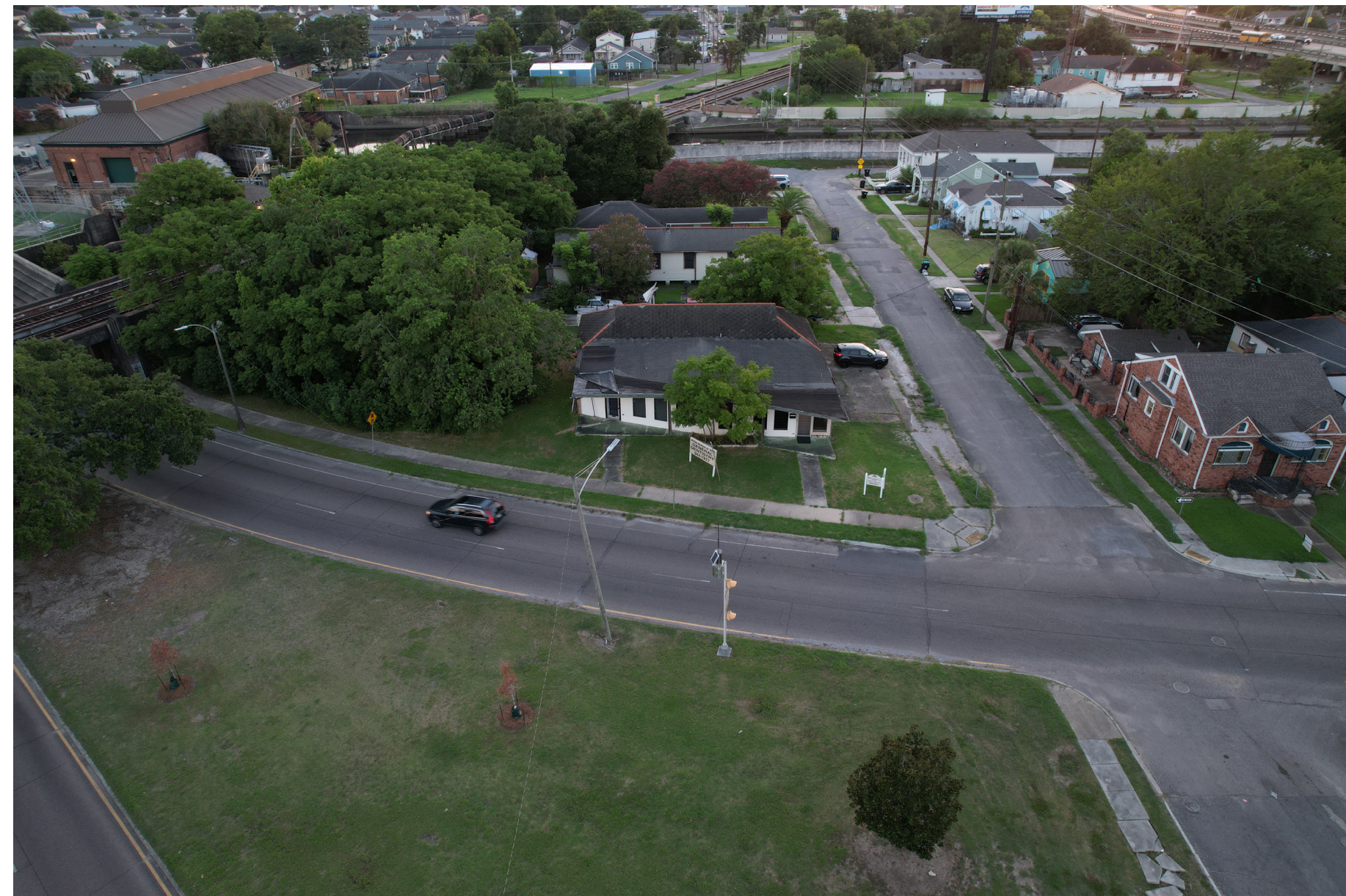
5 SITE PHOTO - AERIAL FROM NEW ORLEANS ST NTS
