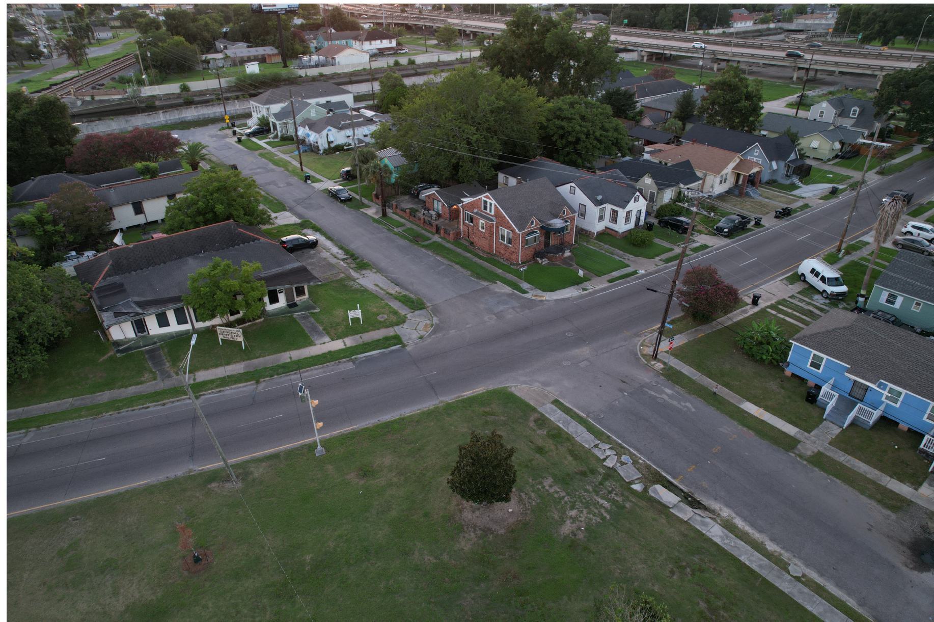
4 SITE PHOTO - INTERSECTION OF NEW ORLEANS ST & TREASURE ST NTS
