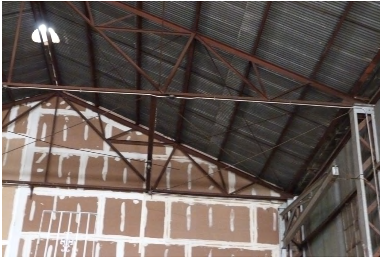
Existing wall on Annunciation Street side: Gypsum board
