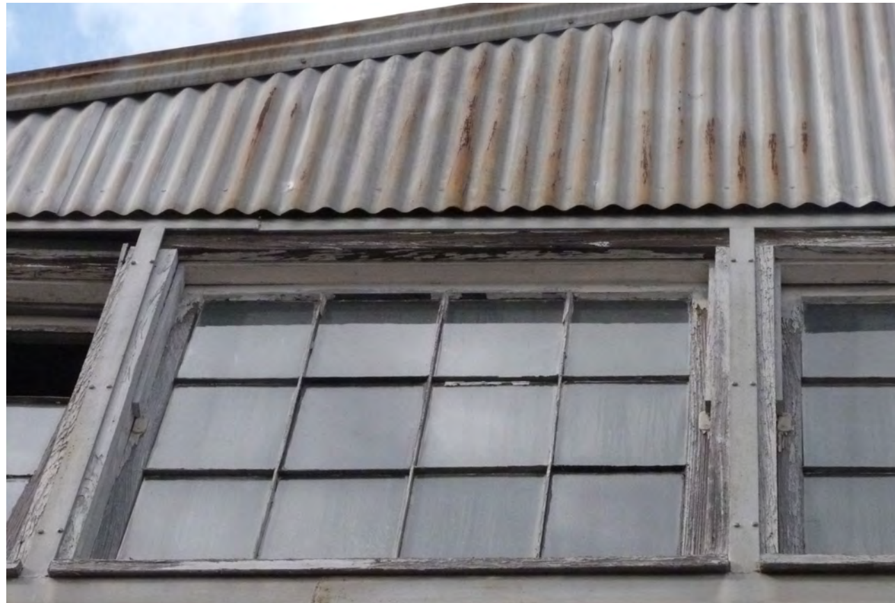
Existing wood framed windows on Tchoupitoulas Street facade
