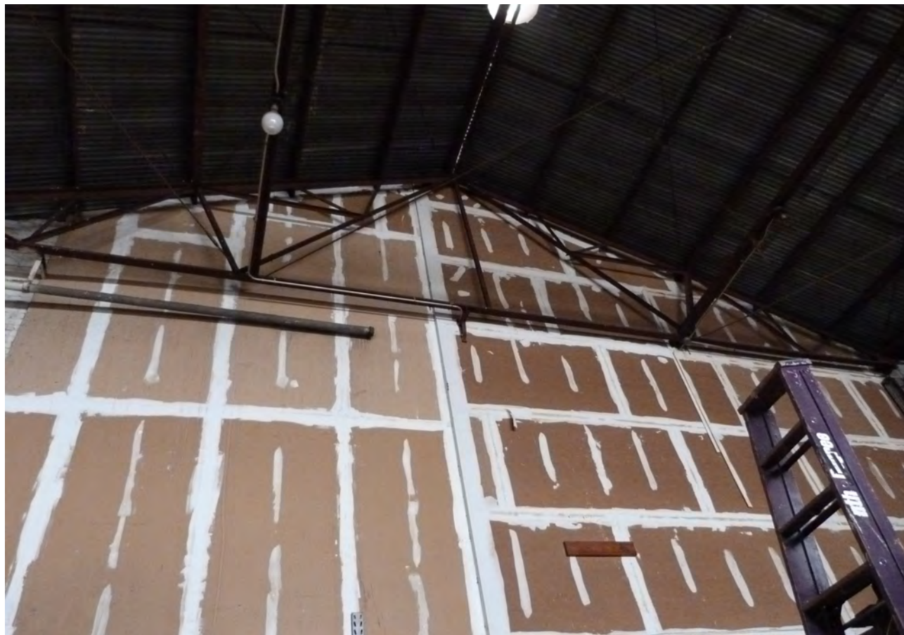
Existing wall on Annunciation Street side: Gypsum board
