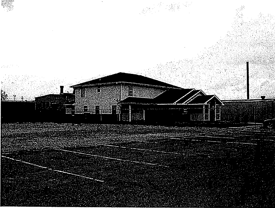
INSIDE SITE TOWARDS ADJOINING PROPERTY
