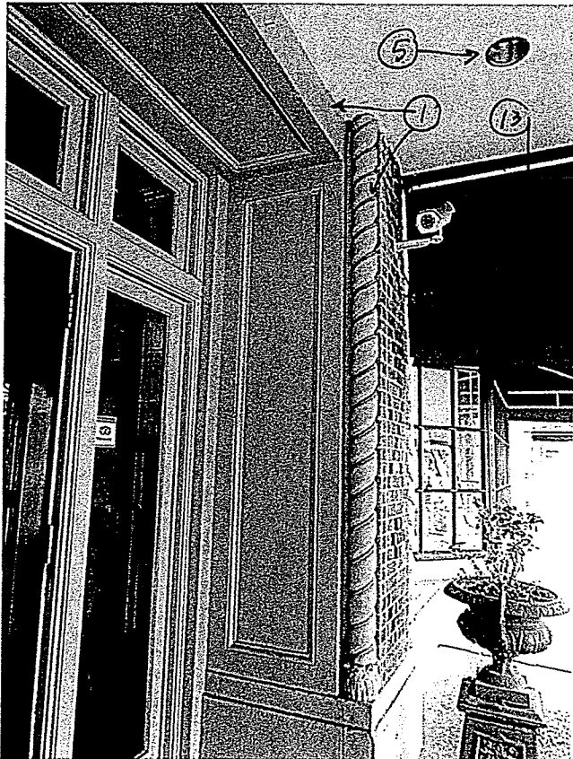
13 REPLACE EXISTING CANVAS BY PRESSED METAL AWNING TO MATCH HISTORIC DETAIL @ MAIN CANOPY.
