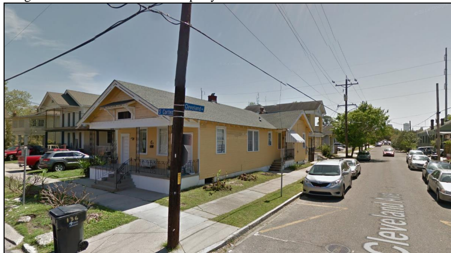
Image #2: Front of Petitioned Property
