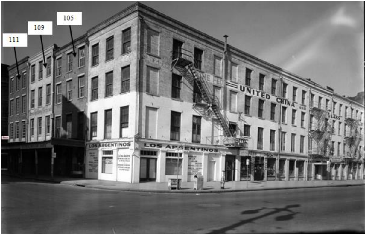
Photo of the corner of Canal and Tchoupitoulas Streets, 1956. Charles Frank.
