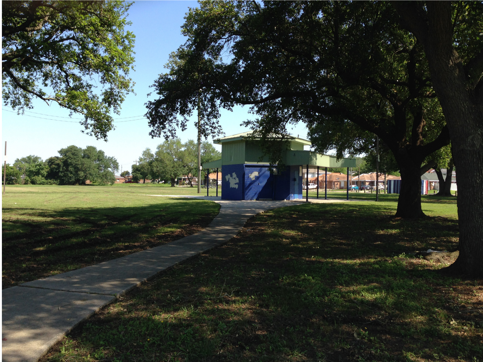
Site Images - Existing Concessions Building to be removed.
