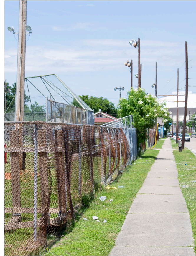
Perimeter fence along S. Derbigny Street
