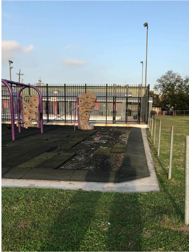
Playground safety surface
