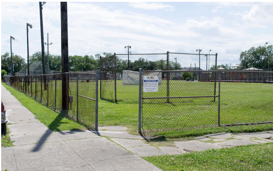
Pedestrian entrance at corner of Third Street and S. Derbigny Street
