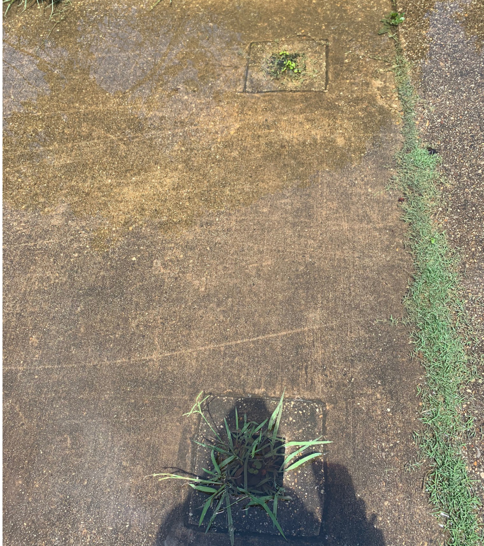
Bollard Footings at Entry Points
