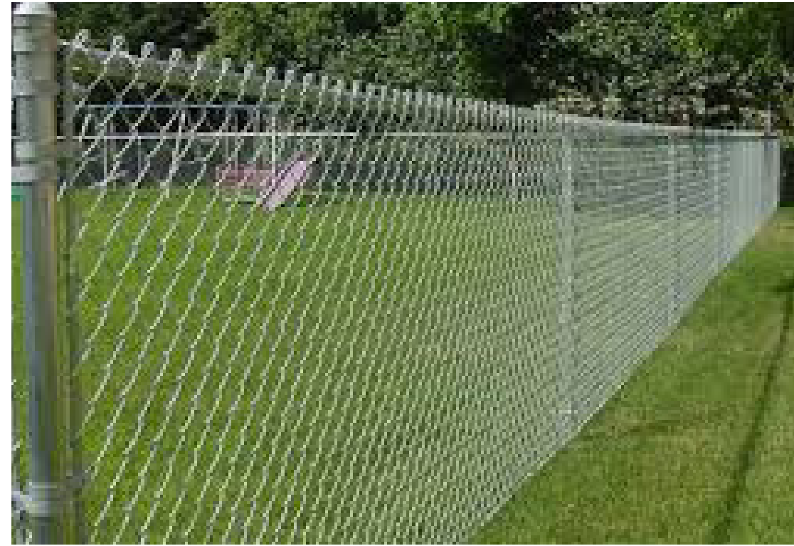
New Chain Link Fence
