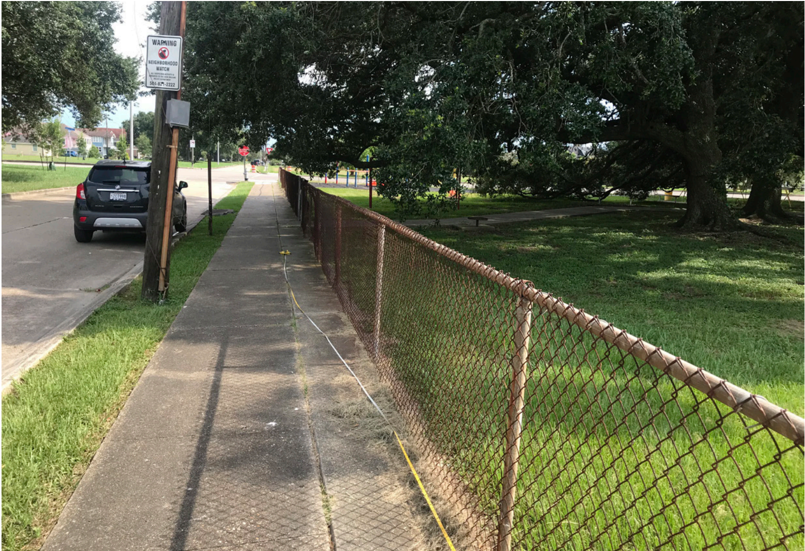
Fence along the rear, west side of the park. Adjacent to existing city fence.
