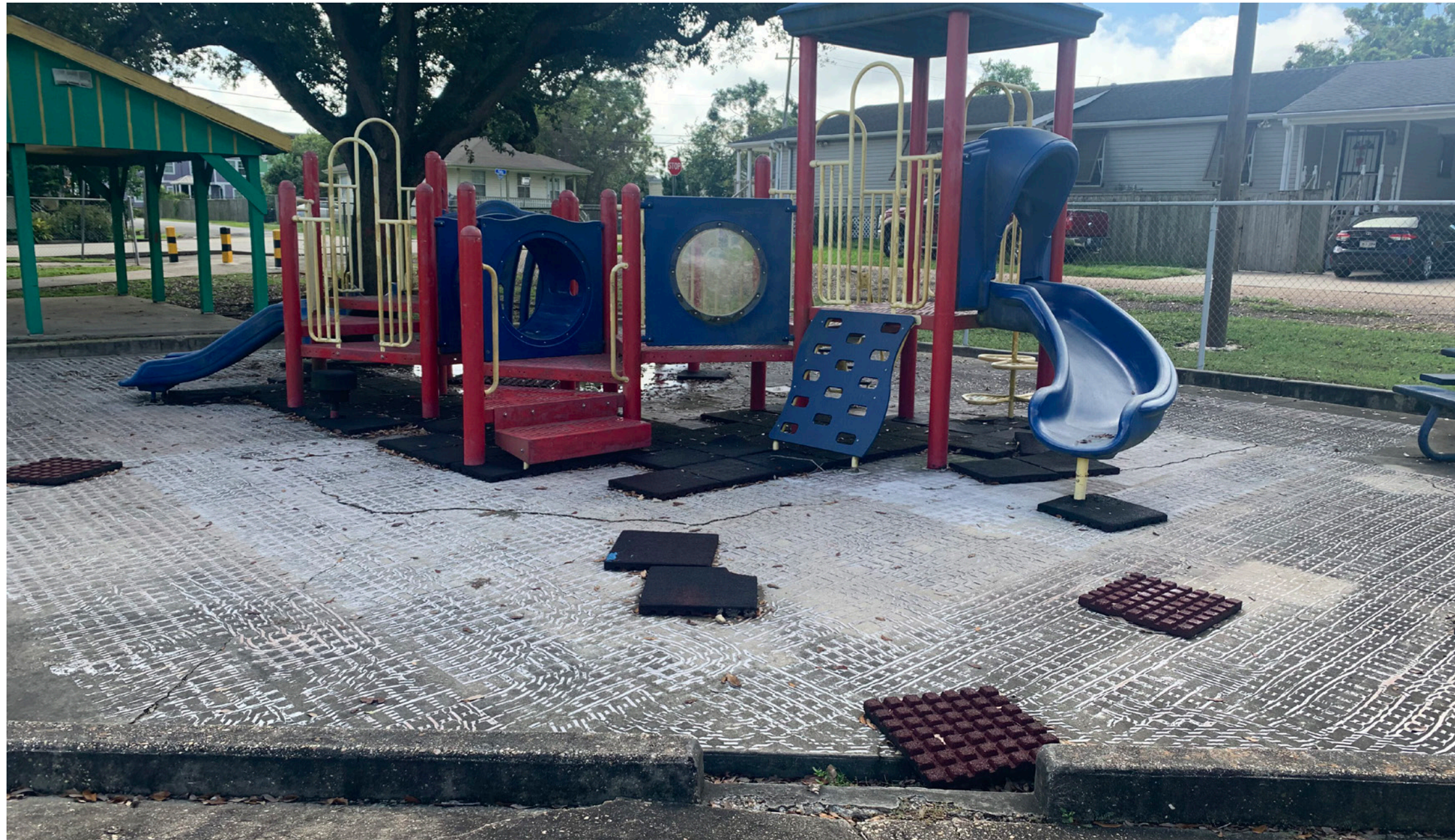
Location of New Poured in Place Safety Surfacing
