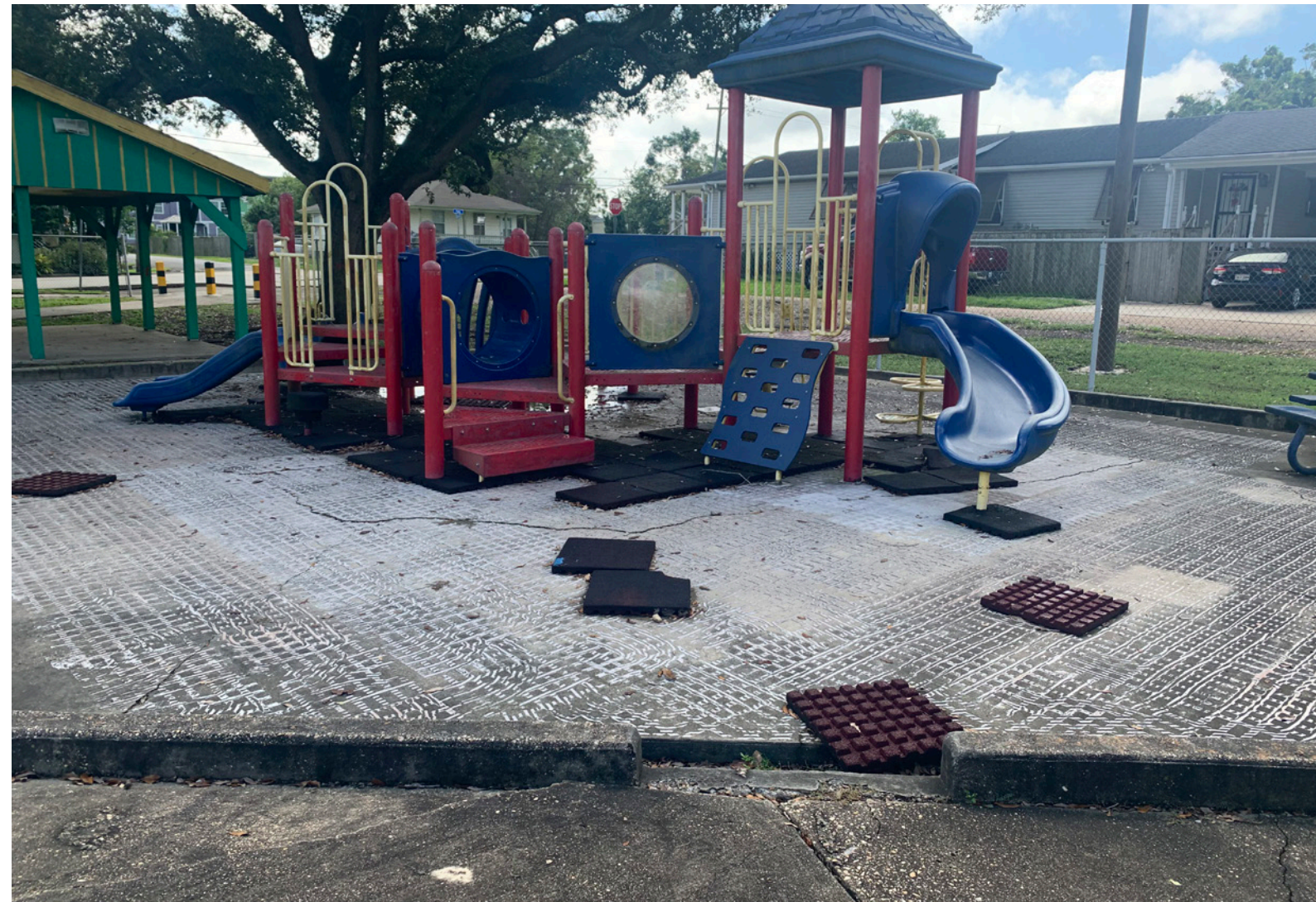
Playset with broken playground tiles.
