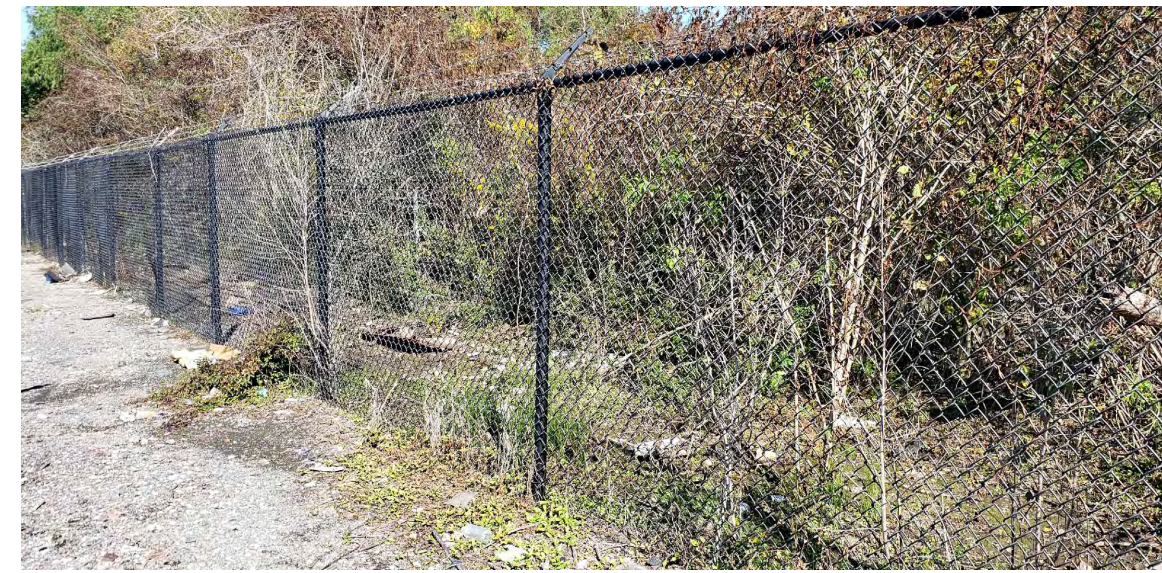
P06 EXISTING CONDITION PHOTO N.T.S.
