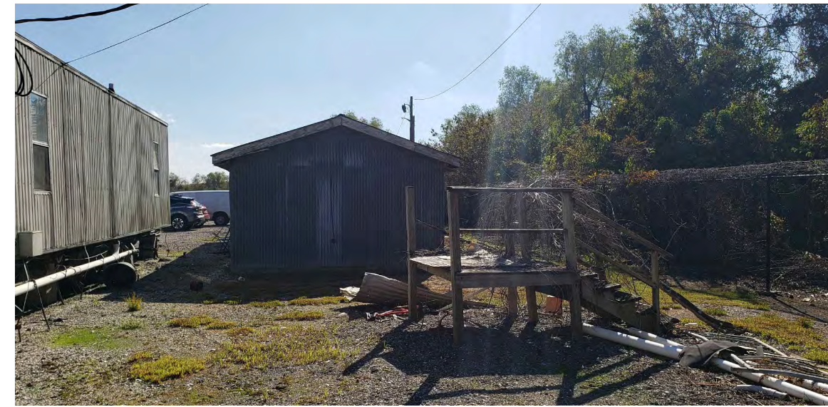
P09 EXISTING CONDITION PHOTO N.T.S.
