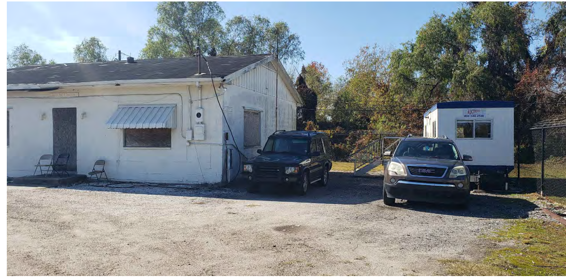
P01 EXISTING CONDITION PHOTO N.T.S.
