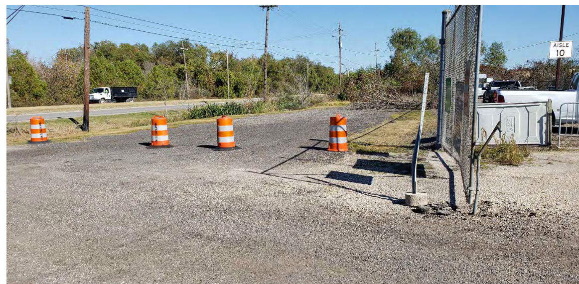
P14 EXISTING CONDITION PHOTO N.T.S.
