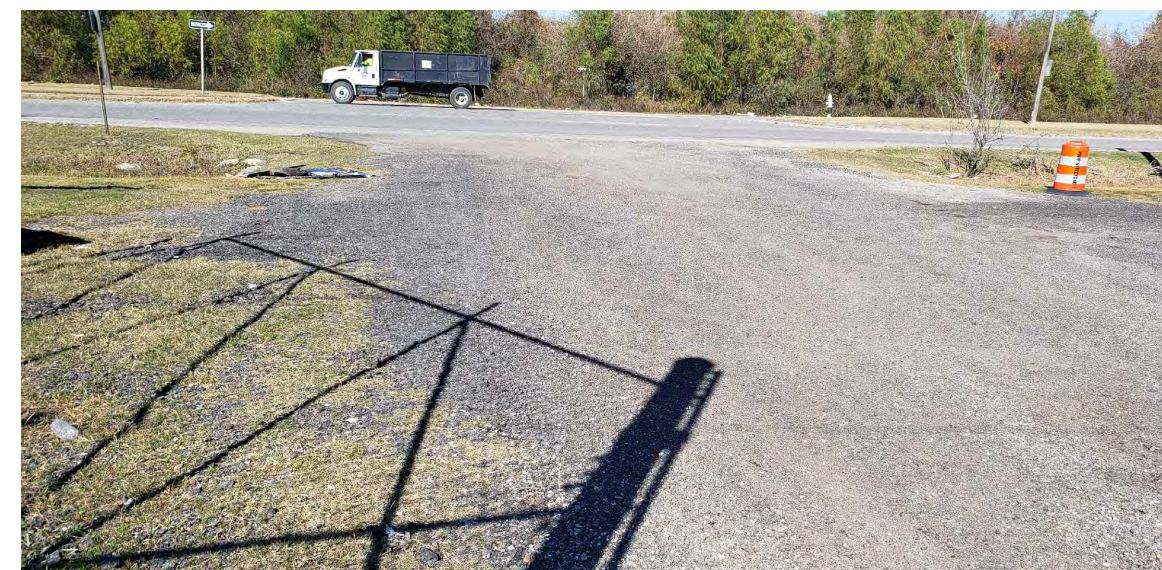
P15 EXISTING CONDITION PHOTO N.T.S.
