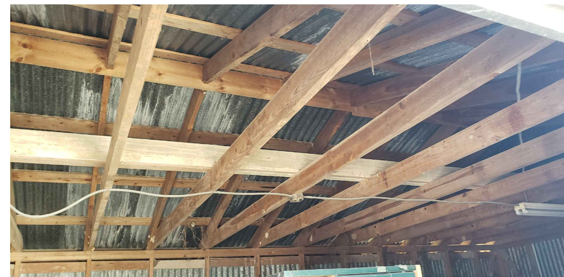
P12 EXISTING CONDITION PHOTO N.T.S.
