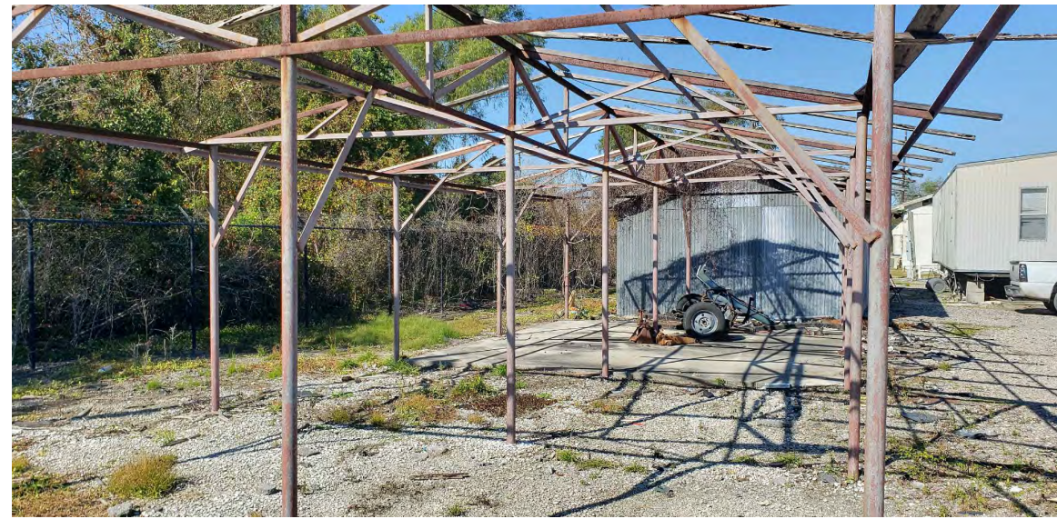
P08 EXISTING CONDITION PHOTO N.T.S.
