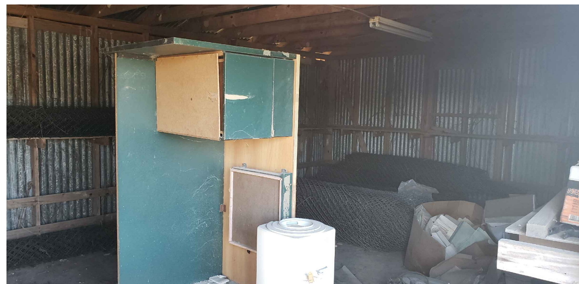
P11 EXISTING CONDITION PHOTO N.T.S.
