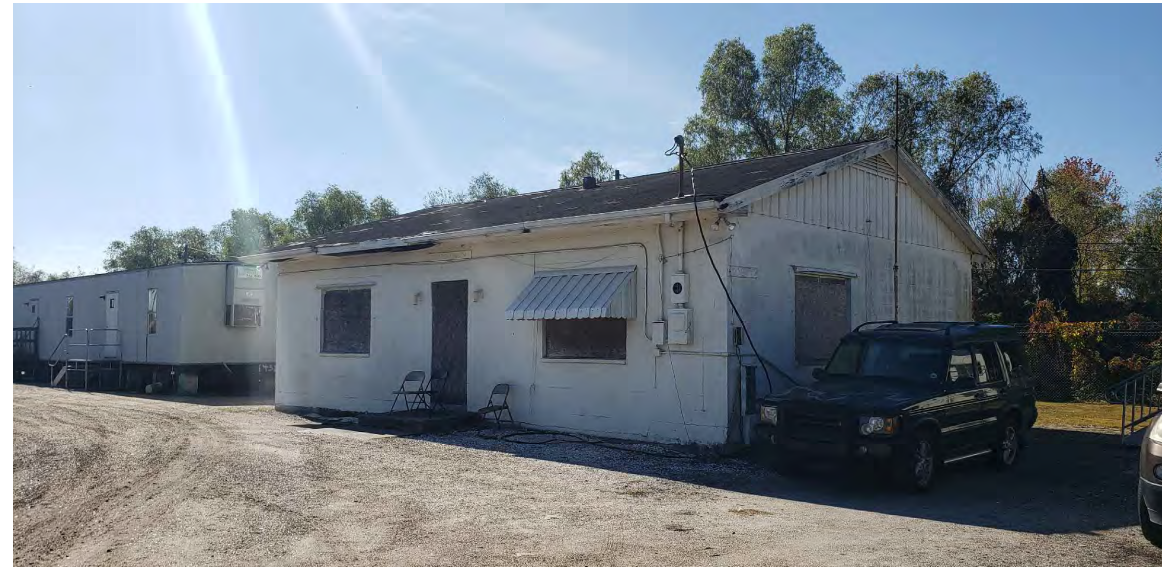
P02 EXISTING CONDITION PHOTO N.T.S.
