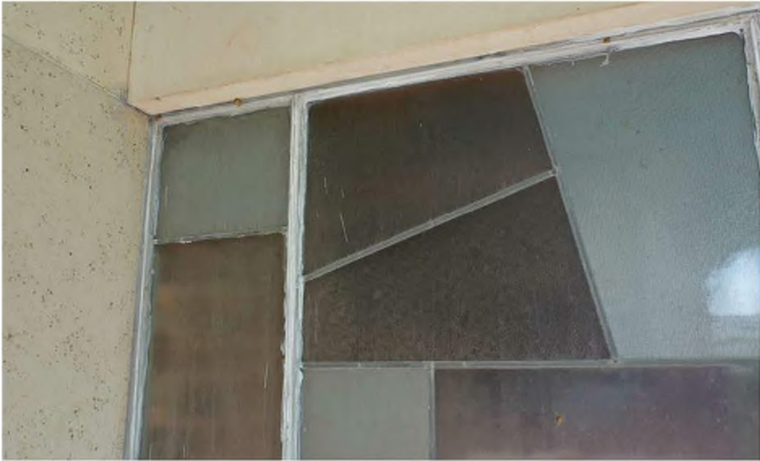
6 EXISTING LEADED GLASS TO REMAIN, TYP. THROUGHOUT. PUTTY & SEALANT TO BE ABATED AND REPLACED WITH NEW (TYP.)
