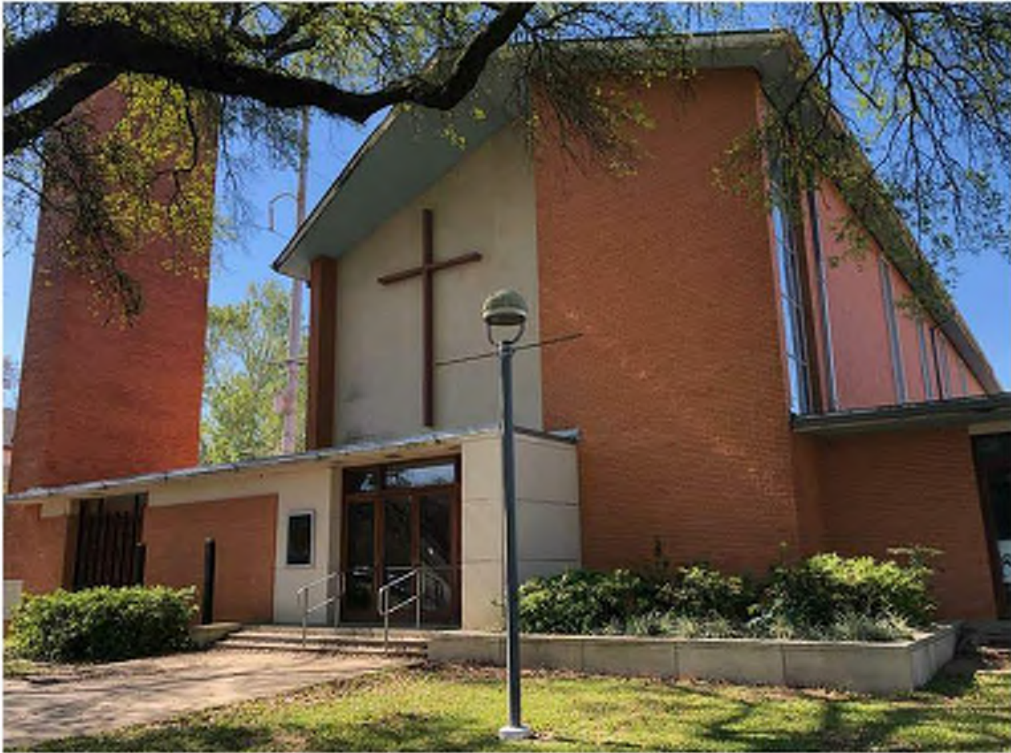
1 CANAL STREET FACADE, SHOWING ENTRY TO SANCTUARY. DAMAGED WOOD STOREFRONT DOORS TO BE REPLACED IN KIND; BRICK AND CAST STONE TO BE CLEANED AND REPAIRED WHERE NOTED (RE: BUILDING ELEVATIONS). DAMAGED TO CAST STONE CROSS TO BE REPAIRED, NEW IN-GROUND LED UPLIGHTING TO BE INSTALLED (RE: SITE PLAN). ENTIRE BUILDING TO BE ROOFOFF (RE: ROOF DRAWINGS & SPECIFICATIONS.)
