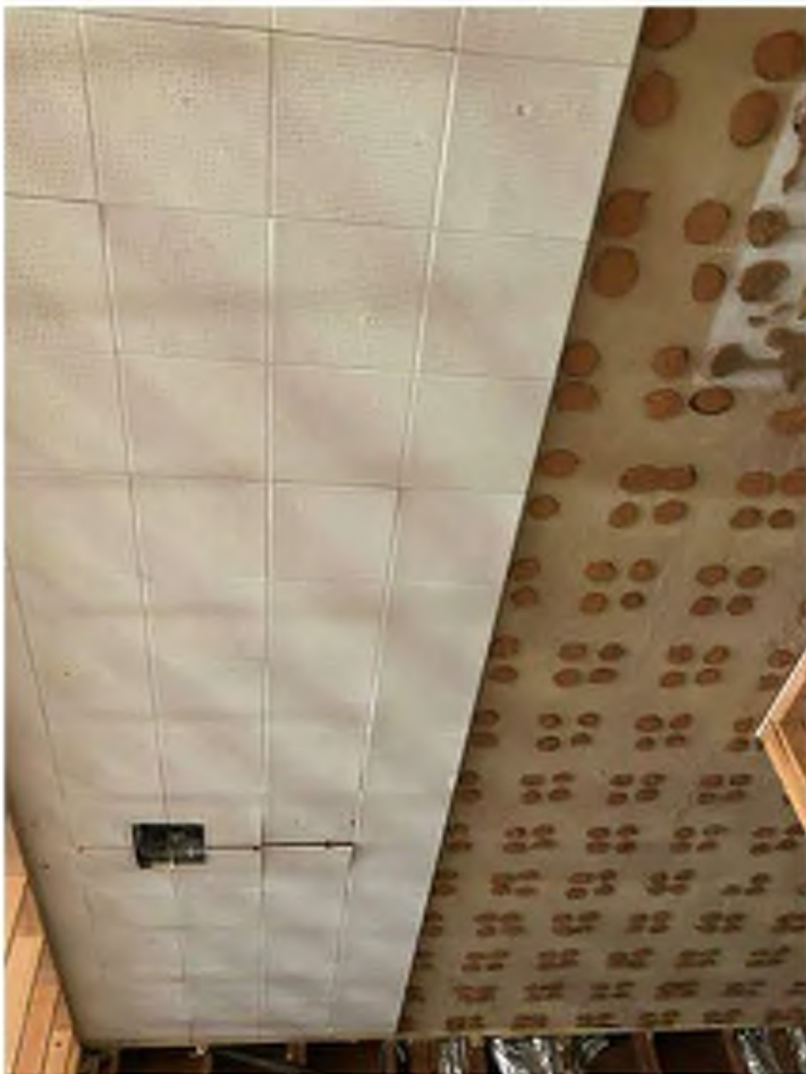
10 EXISTING ACOUSTIC TILE CEILING TO BE DEMOLISHED AT EXISTING CHURCH ADMINISTRATION AREA (NEW DAYCARE AREAS.) NEW SUSPENDED GYP CEILING TO BE INSTALLED (RE: RCP).
