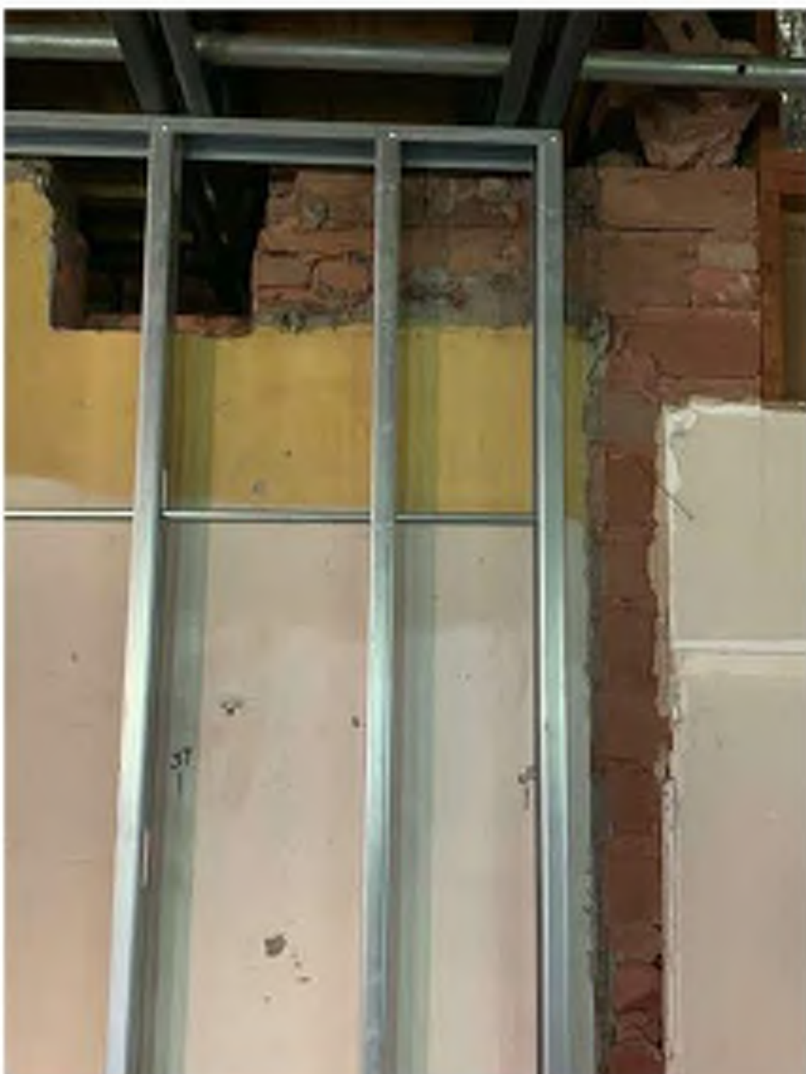
15 NON-HISTORIC METAL STUD FURRING TO BE REMOVED AT NEW RESTROOMS / NEW LOBBY (PREVIOUS CHURCH ADMINISTRATION AREA.)
