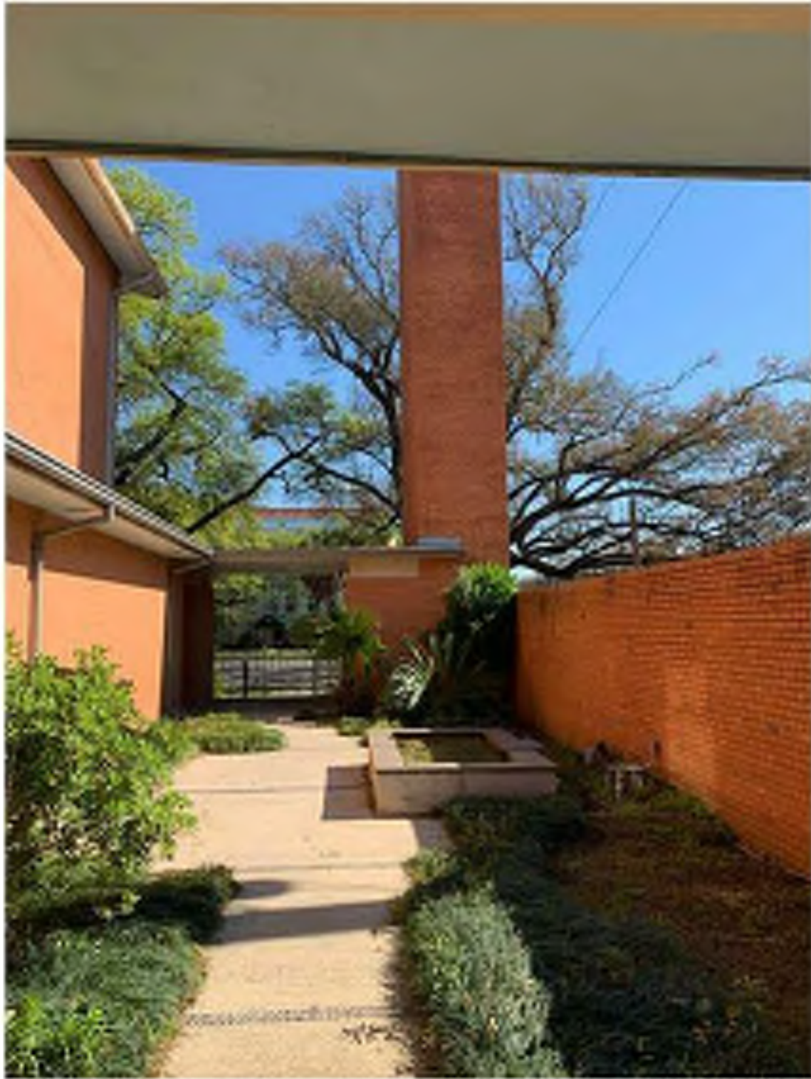
3 INTERNAL COURTYARD LOOKING TOWARD CANAL STREET. EXISTING PAVING AND WATER FEATURE TO BE DEMOLISHED. NEW RAISED PLANTING BED AND PERMEABLE PAVING TO BE INSTALLED (RE: SITE PLAN). NEW DS AND GUTTERS TO BE REPLACED IN KIND IN SAME LOCATIONS, TYP. THROUGHOUT.
