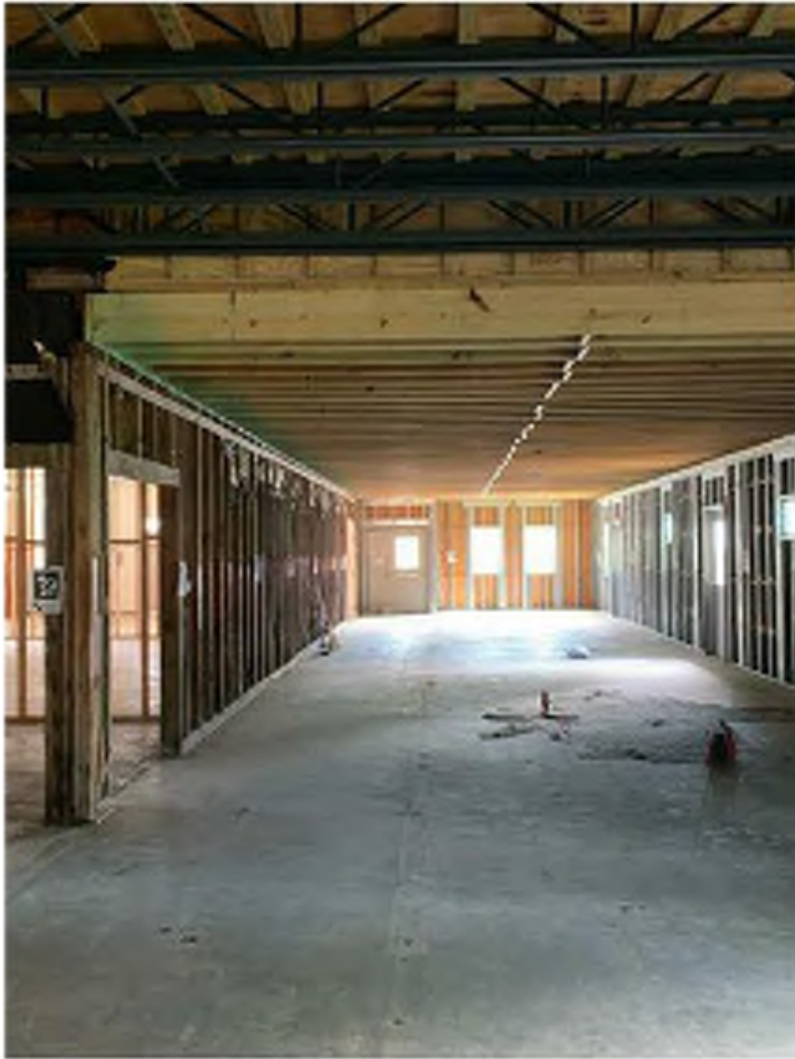
1 EXISTING CHURCH ADMINISTRATION SPACE. ROOF FRAMING TO REMAIN. SPACE TO BE SUBDIVIDED AS SHOWN IN PLAN. EXISTING WINDOWS AND DOORS TO BE REPLACED WITH IMPACT RATED GLAZING ASSEMBLIES (RE: BUILDING ELEVATIONS, SCHEDULES). NEW ENGINEERED WOOD FLOORING TO BE INSTALLED THROUGHOUT.
