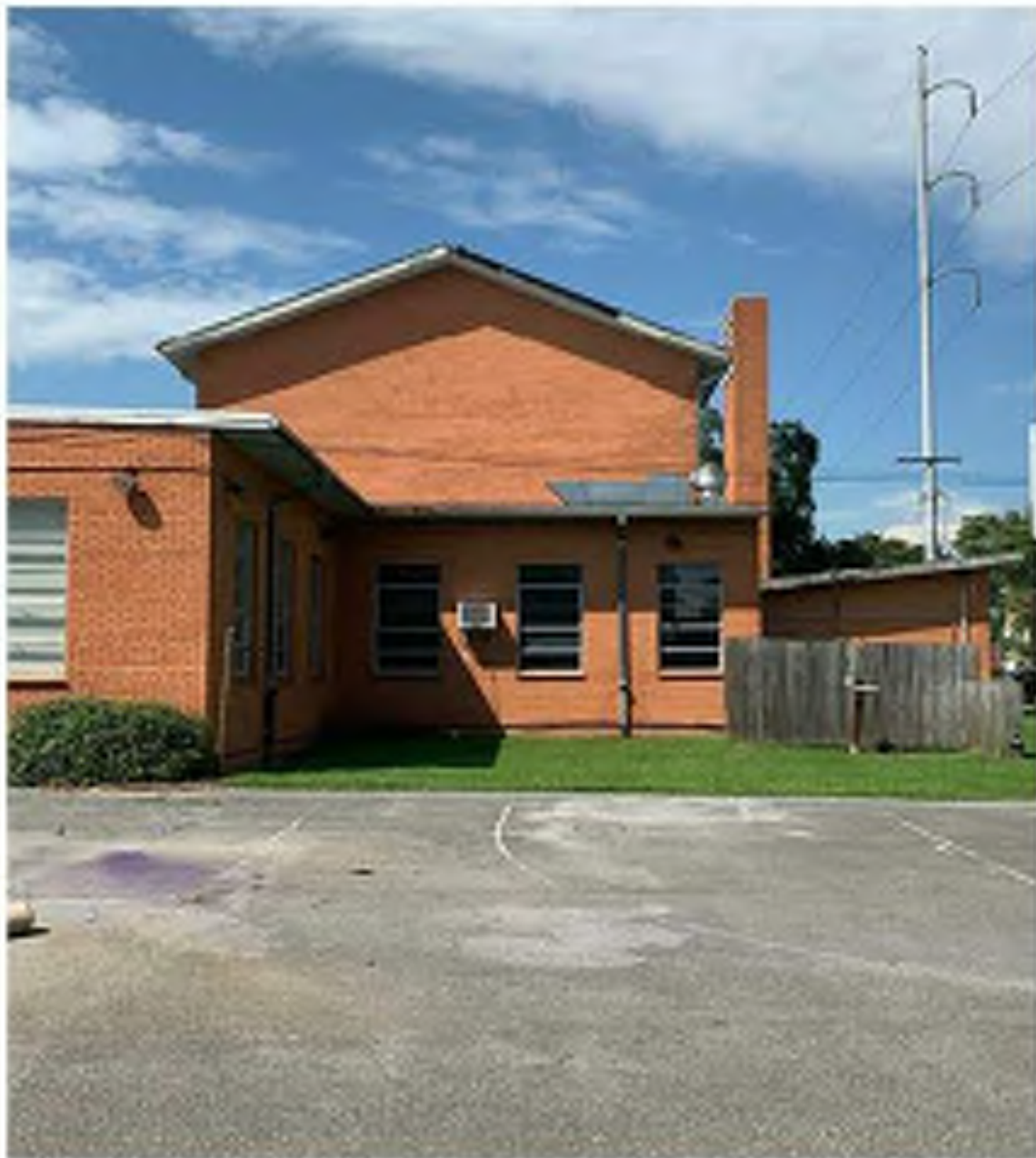
5 SECONDARY FACADE (HIDDEN FROM PUBLIC RIGHT OF WAY) ON S. CORTEZ ST. SIDE WITH NON-HISTORIC H.M. & VINYL OPENINGS. FIBER CEMENT SIDING. OPENINGS TO BE MODIFIED, RELOCATED, AND REPLACED (RE: BUILDING ELEVATIONS) WITH RECEIVE NEW WINDOWS. NEW ENTRY WALKWAY TO BE INSTALLED WITH PLANTING. ROOFS, GUTTERS, AND DOWNSPOUTS TO BE REPLACED IN KIND IN SAME LOCATIONS.
