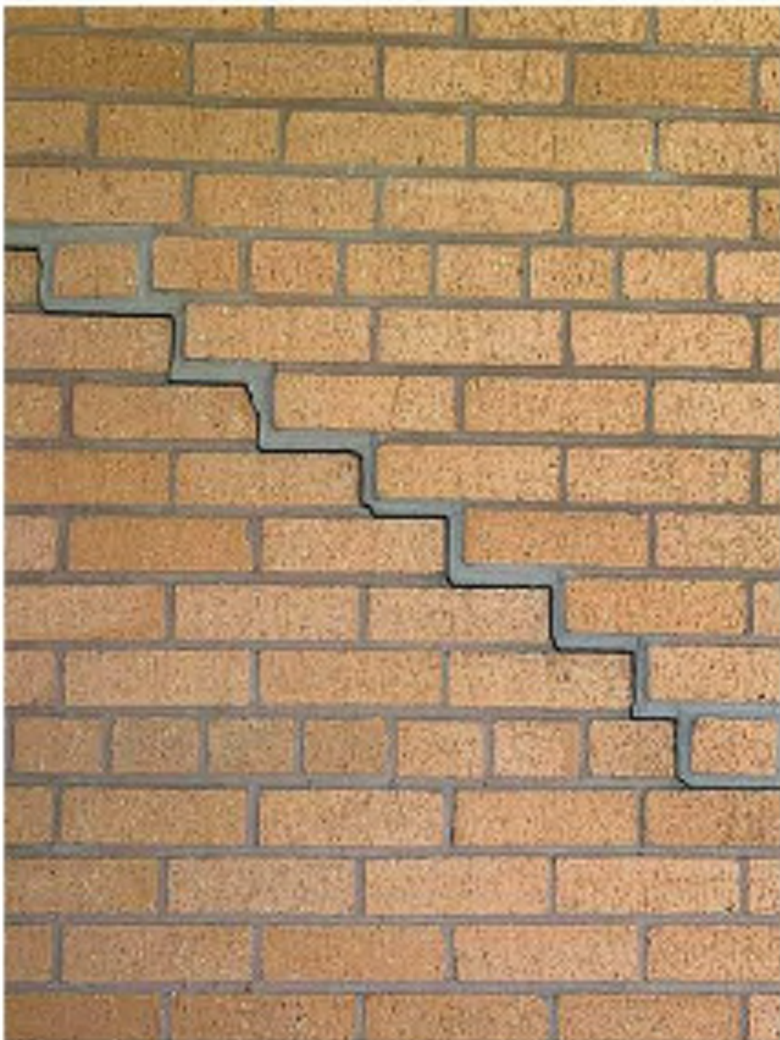
10 EXISTING STEP CRACKING DUE TO SETTLING AT LOGGIA ON CANAL STREET FACADE TO BE REPAIRED & REPOINTED.
