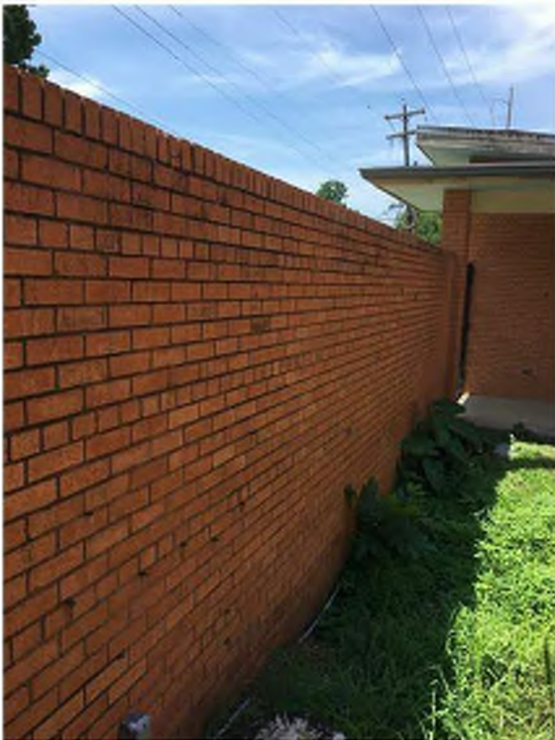
8 EXISTING INTERNAL COURTYARD WALL, LOOKING TOWARD S. TELEMACHUS STREET. EXISTING PLANTING TO BE REMOVED. NEW PAVING, GROUNDCOVER AND PLANTING TO BE INSTALLED (RE: SITE PLAN). EXISTING PLASTER SOFFIT TO REMAIN. BRICK TO BE CLEANED AND REPAIRED AS SHOWN (RE: BUILDING ELEVATIONS).
