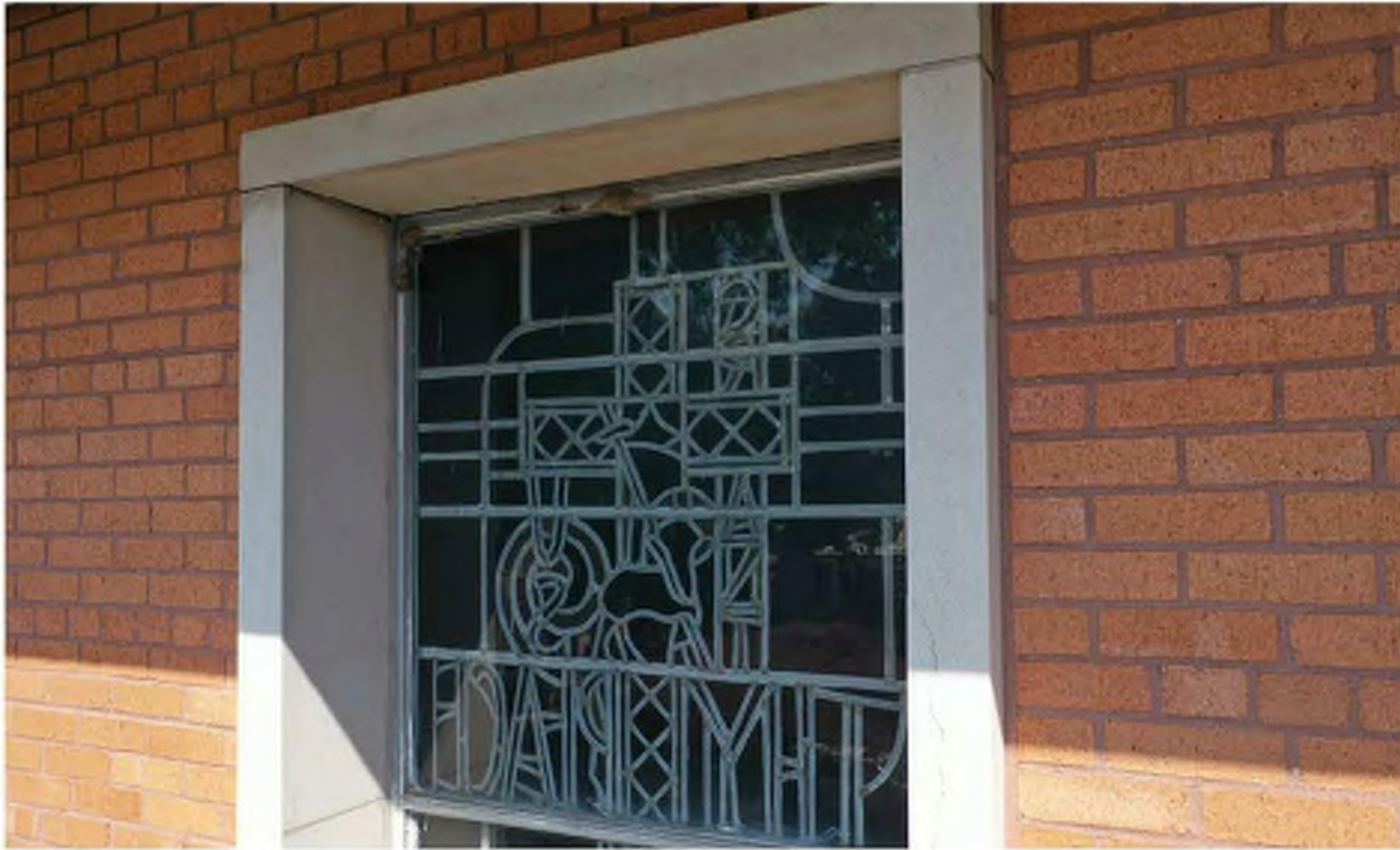
7 EXISTING HISTORICAL STAINED GLASS (SEEN FROM EXTERIOR). BRICK AND CAST STONE ELEMENTS TO BE CLEANED AND REPAIRED AS SHOWN (RE: BUILDING ELEVATIONS).
