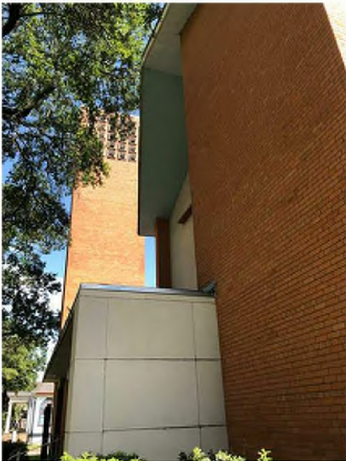
8 CANAL STREET ELEVATION SHOWING WORSHIP ENTRY AND BELLTOWER (SEEN FROM S. CORTEZ ST. SIDE). EXISTING CAST STONE AND BRICK TO BE CLEANED AND REPAIRED (RE: BUILDING ELEVATIONS).
