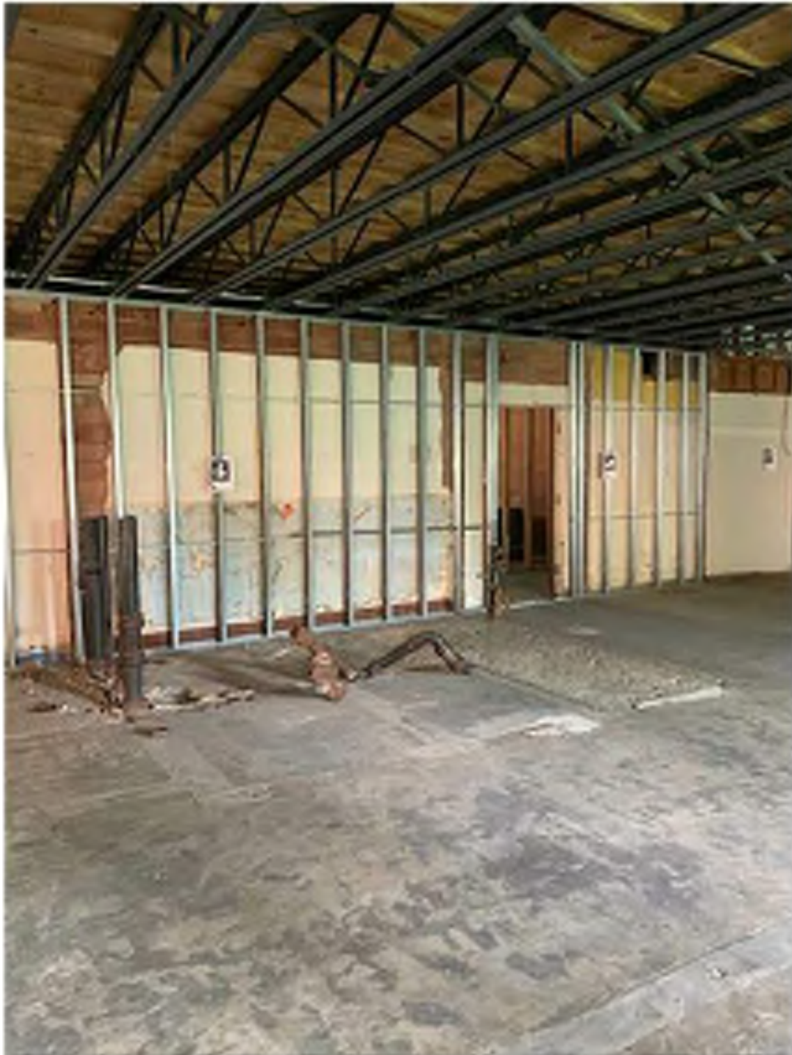
5 EXISTING CHURCH ADMINISTRATION SPACE. EXISTING PLUMBING LINES TO BE CUT TO FLOOR LEVEL, CAPPED, AND ABANDONED. NEW ENGINEERED WOOD FLOORING TO BE INSTALLED THROUGHOUT. EXISTING WALLS TO BE FINISHED (RE: ASSEMBLY TYPES, ELEVATIONS.) NON-HISTORIC METAL STUD FURRING TO BE REMOVED.
