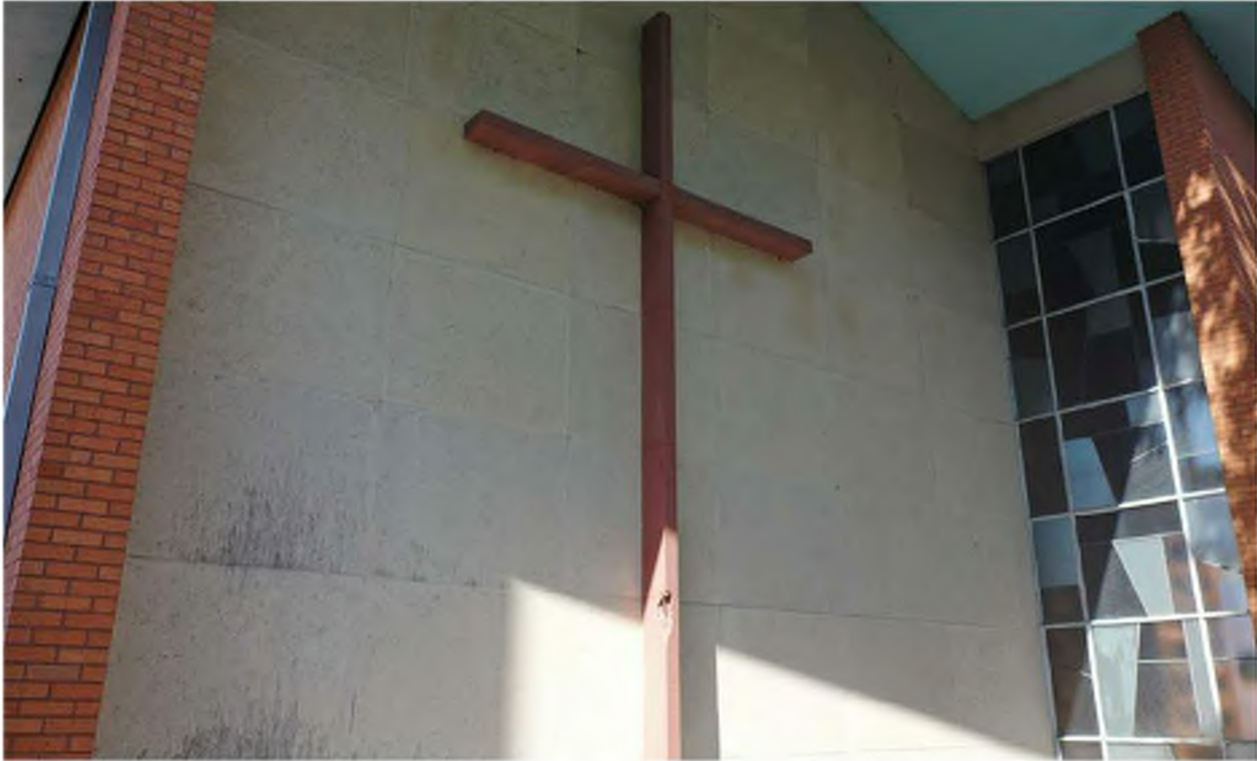
8 EXISTING CAST STONE CROSS AND LEADED GLAZING AT CANAL STREET FACADE. CAST STONE TO BE CLEANED AND REPAIRED AS NOTED IN BUILDING ELEVATIONS.
