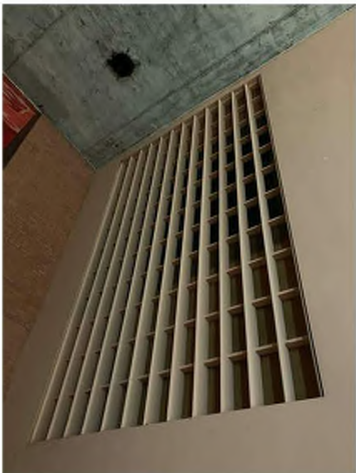
12 EXISTING BAFFLES @ ORGAN LOFT (SIM. BOTH SIDES OF CHANCEL) TO BE DEMOLISHED. OPENING TO BE INFILLED AND FINISHED WITH PLASTER TO MATCH ADJACENT EXISTING WALL.
