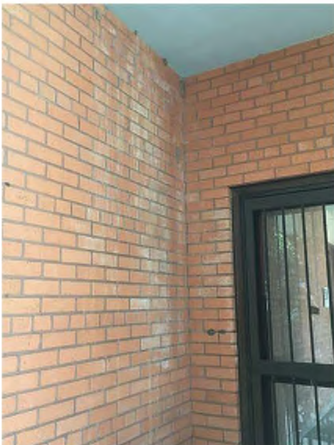
11 EXISTING EFFLORESCENCE AT BRICK IN COURTYARD LOOKING TOWARD ENTRY VESTIBULE (HIDDEN FROM PUBLIC RIGHT OF WAY). BRICK TO BE CLEANED AND REPAIRED AS SHOWN (RE: BUILDING ELEVATIONS). EXISTING PLASTER SOFFIT AND DOOR TO REMAIN.
