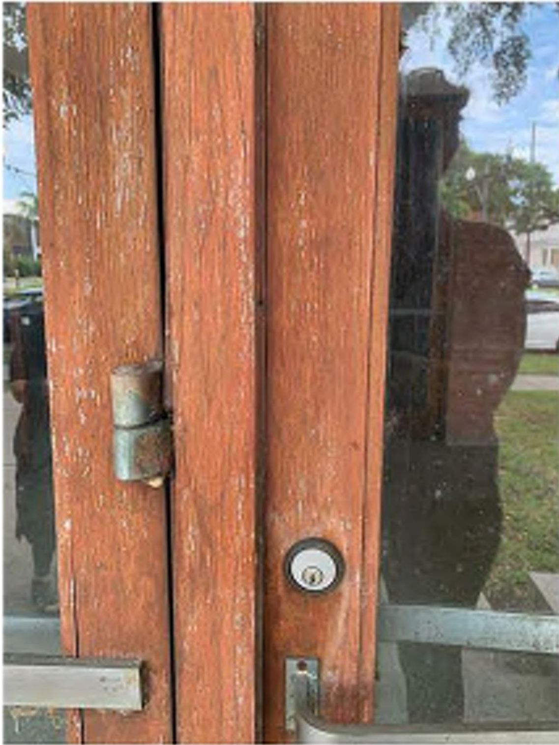
5 EXISTING WOOD STOREFRONT ASSEMBLY AT CANAL STREET FACADE. TO BE REPLACED IN KIND TO MATCH EXISTING PROFILES WITH IMPACT-RATED GLAZING AND ASSEMBLY. HARDWARE TO BE NEW TO MEET LIFE SAFETY REQUIREMENTS.
