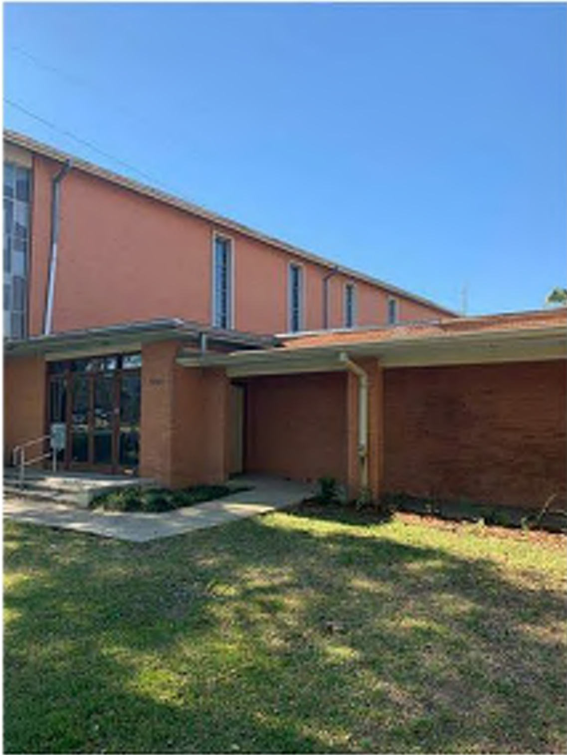
4 EXISTING FACADE SHOWING LOGGIA AND LOBBY ENTRY FROM CANAL STREET. NEW BICYCLE PARKING TO BE ADDED AT LEFT (RE: SITE PLAN). ROOFS TO BE REPLACED THROUGHOUT. NEW GUTTERS AND DOWNSPOUTS TO BE REPLACED IN KIND IN SAME LOCATIONS, TYP. THROUGHOUT. EXISTING STAINED AND LEADED GLASS TO REMAIN.
