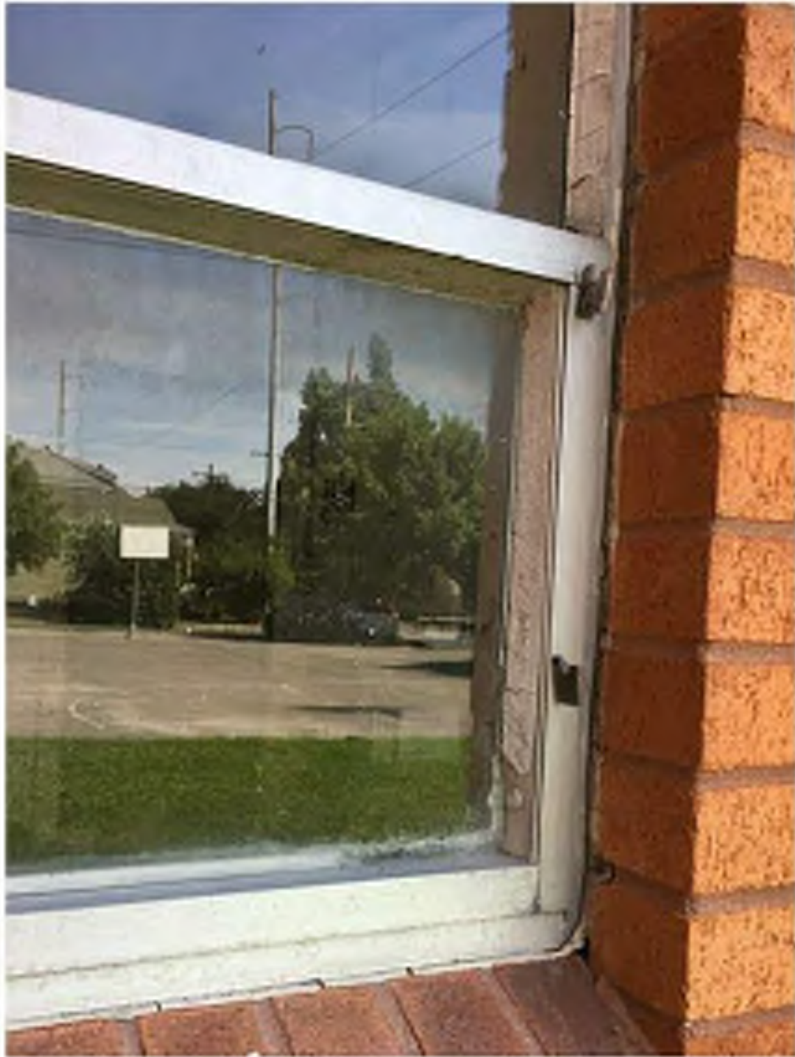
2 SECONDARY CLEVELAND AVE FACADE (HIDDEN FROM PUBLIC RIGHT OF WAY) SHOWING EXISTING HISTORIC WINDOWS. NEW IMPACT RATED GLAZING AND ASSEMBLIES TO BE INSTALLED (RE: BUILDING ELEVATIONS). BRICK TO BE CLEANED AND REPAIRED AS SHOWN (RE: BUILDING ELEVATIONS).
