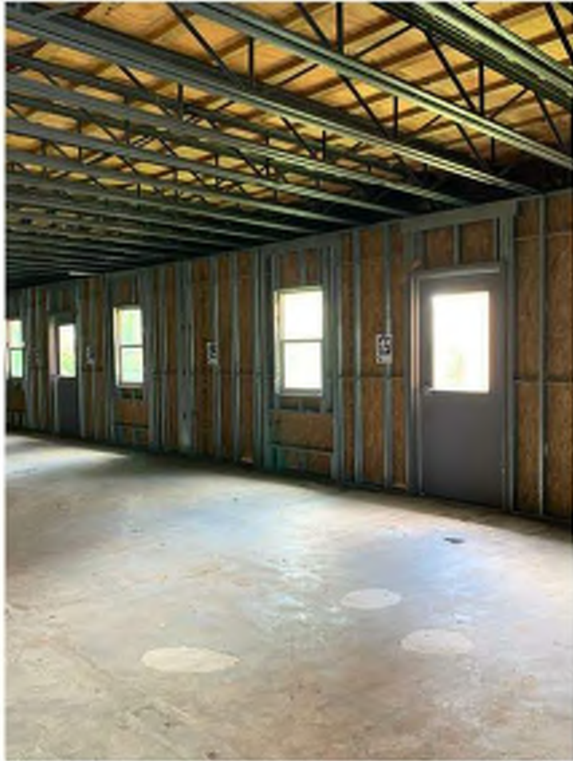
2 EXISTING CHURCH ADMINISTRATION SPACE. ROOF FRAMING TO REMAIN. SPACE TO BE SUBDIVIDED AS SHOWN IN PLAN. EXISTING WINDOWS AND DOORS TO BE REPLACED WITH IMPACT RATED GLAZING ASSEMBLIES (RE: BUILDING ELEVATIONS, SCHEDULES). NEW ENGINEERED WOOD FLOORING TO BE INSTALLED THROUGHOUT.
