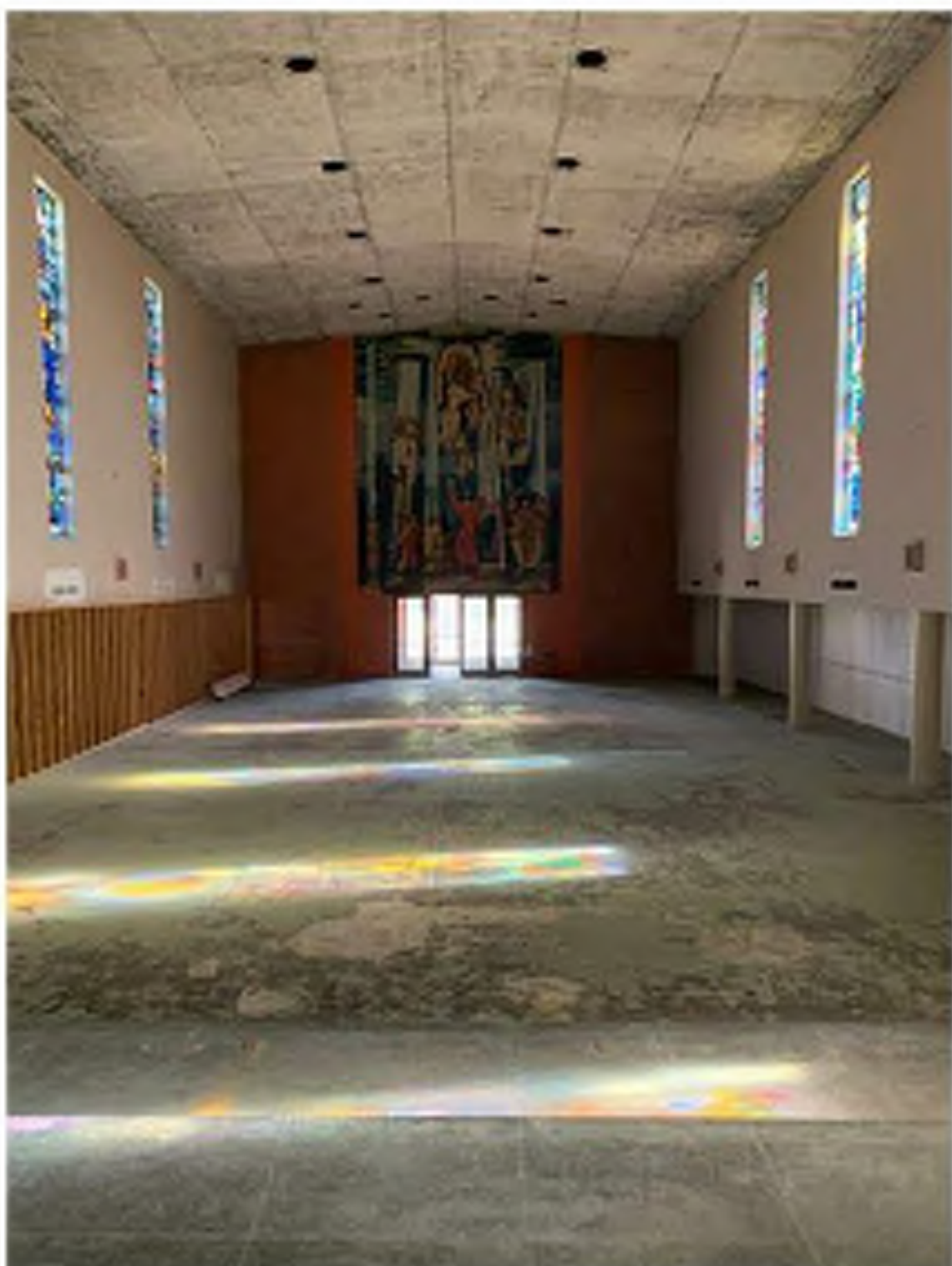
12 EXISTING WORSHIP SPACE LOOKING TOWARD CANAL STREET FROM ALTAR. EXISTING STAINED GLASS WINDOWS AND HISTORIC MURAL TO REMAIN. NON-HISTORIC STUD WALL TO LEFT AND SURFACE MOUNTED SPEAKERS TO BE REMOVED (RE: DEMO PLAN). EXISTING CEILING TO BE DEMOLISHED ABOVE SEATING (EXISTING CHEVRON CEILING TO REMAIN ABOVE ALTAR PLATFORM. RE: REFLECTED CEILING PLAN). NEW SHAPED ACOUSTIC CEILING TO BE INSTALLED. NEW CARPET TO BE INSTALLED. EXISTING TERRAZZO AT ALTAR TO REMAIN. EXISTING BRICK TO REMAIN. EXISTING PAINTED WALLS TO BE REPAINTED, ROOM.
