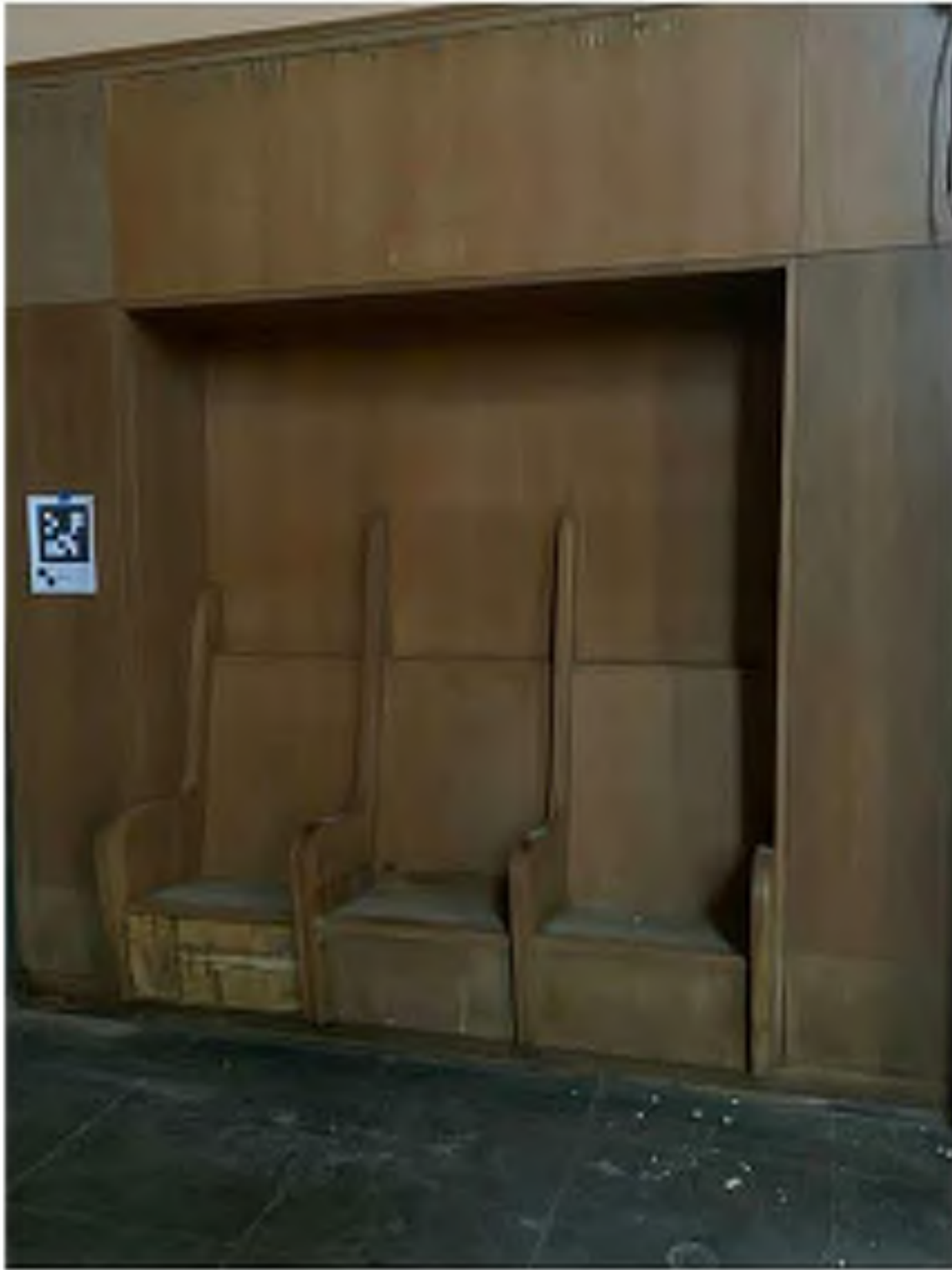
5 DAMAGED WOODEN SEDIA SEATING IN CHANCEL TO BE REMOVED AND SALVAGED TO OWNER. OPENING TO BE INFILLED TO MATCH EXISTING WALL ABOVE AND PAINTED.
