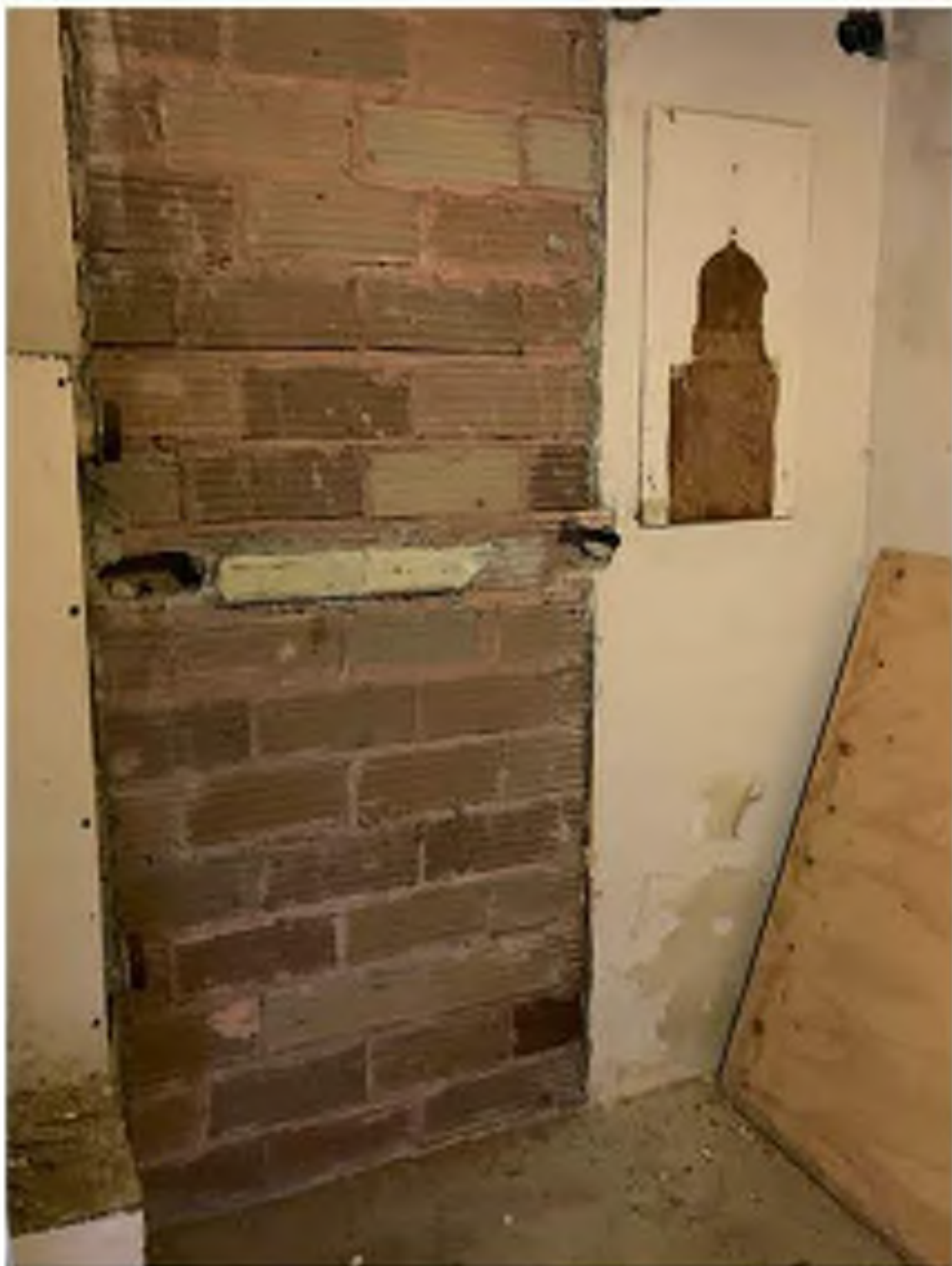
9 EXISTING STRUCTURAL TERRA COTTA CLAY TILE BEARING WALL TO REMAIN.
