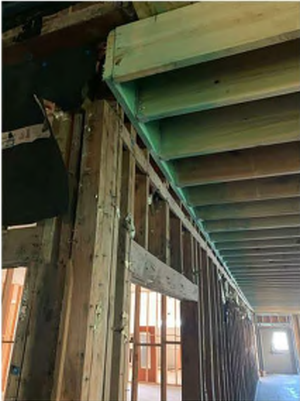
3 EXISTING STRUCTURAL FRAMING IN CHURCH ADMINISTRATION SPACE TO BE REMOVED & REPLACED WITH NEW.
