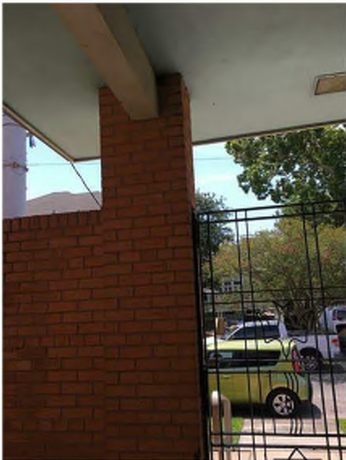
7 INTERNAL COURTYARD AND METALWORK GATE LOOKING TOWARD S. TELEMACHUS STREET. METALWORK TO BE LEAD ABATED, CLEANED AND PAINTED. EXISTING PLASTER SOFFIT TO REMAIN.
