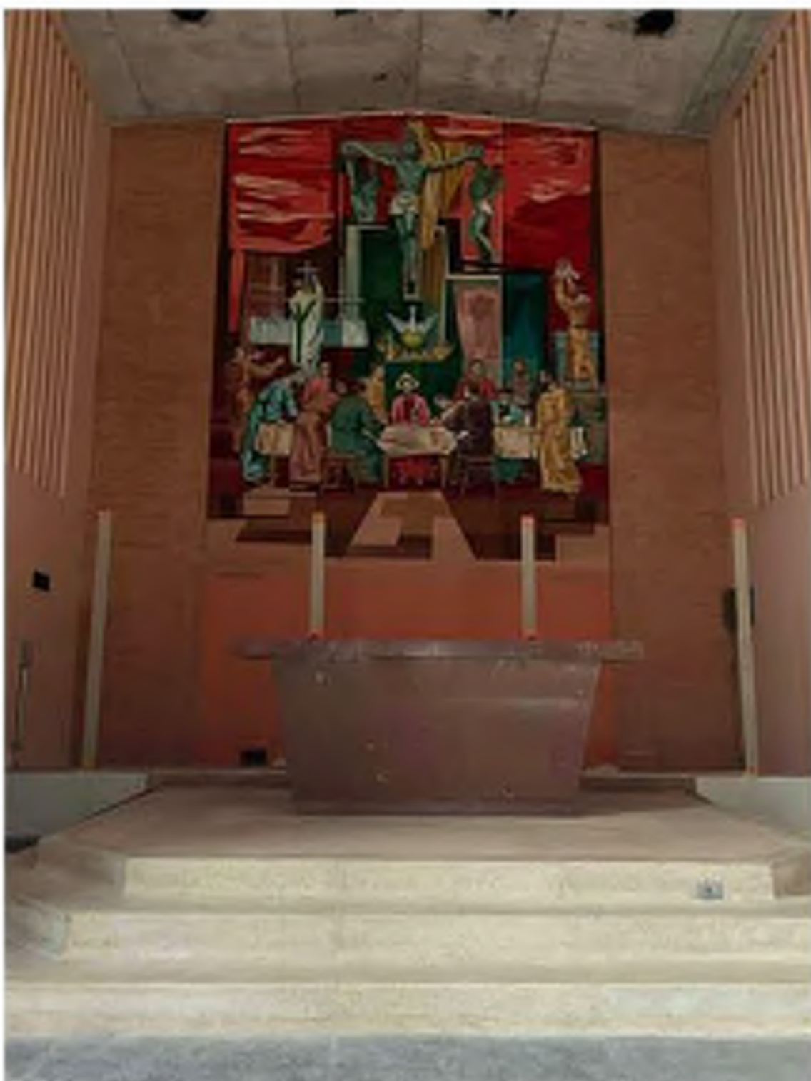
13 EXISTING SANCTUARY LOOKING TOWARD ALTAR FROM CANAL STREET. EXISTING HISTORIC MURAL TO REMAIN. EXISTING CEILING ABOVE ALTAR PLATFORM TO REMAIN (RE: RCP). EXISTING TERRAZZO ALTAR AND STEPS TO BE REMOVED AND FILLED WITH TERRAZZO FINISH TO MATCH EXISTING. REMAINING TERRAZZO PLATFORM TO BE PROTECTED. NEW SCREEN WALL, THEATRICAL SCRIM, PROJECTION SCREEN, AND THEATRICAL LIGHTING TO BE INSTALLED AS INDICATED (RE: PLAN, ELEVATIONS, RCP). EXISTING BAFFLES TO ORGAN LOFT TO BE REMOVED AND FILLED WITH PLASTER FINISH TO MATCH ADJACENT EXISTING. SIDE WALLS OF CHANCEL TO BE PAINTED.
