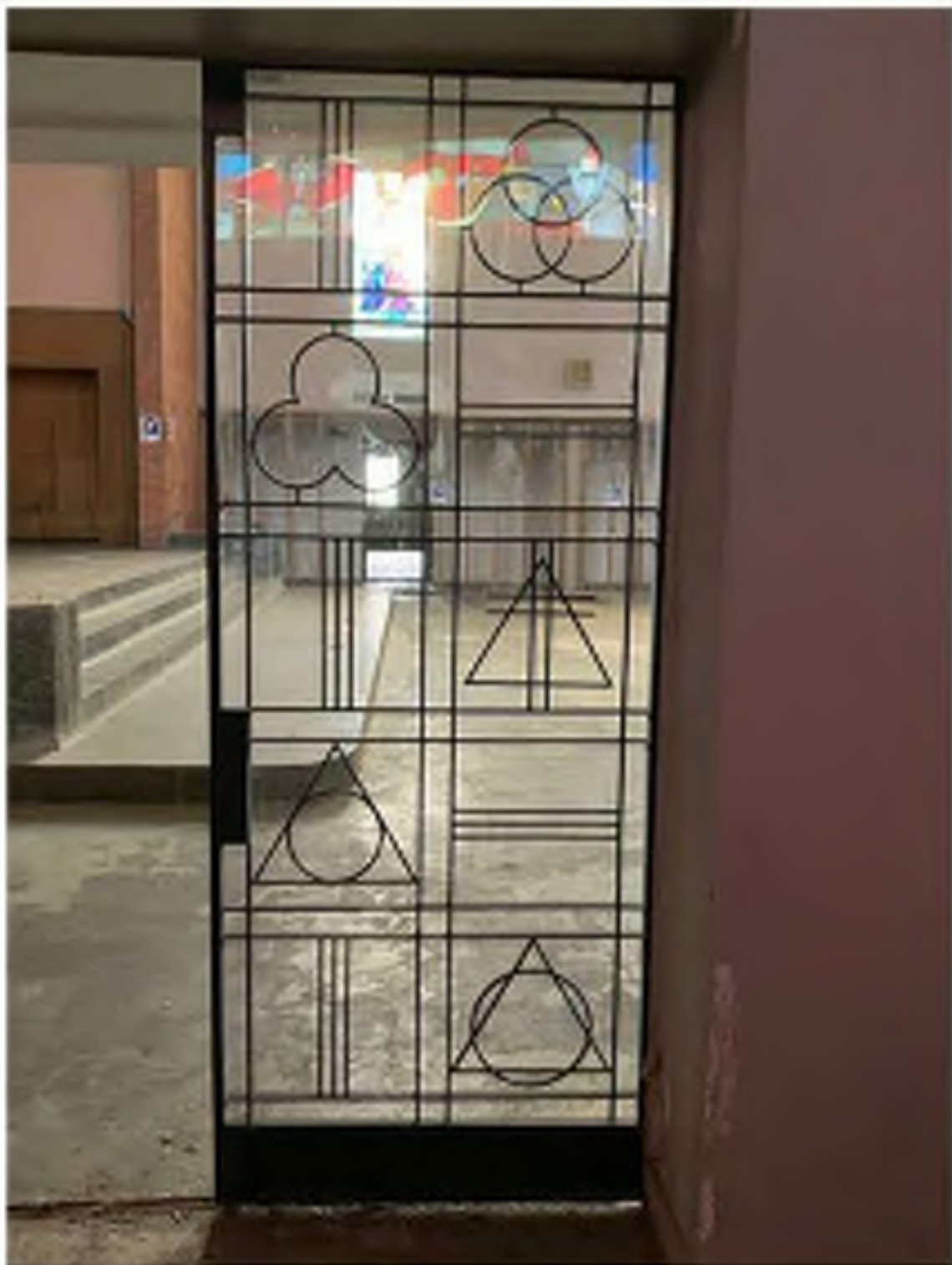
7 EXISTING GLAZED METALWORK DOUBLE DOORS AT CHAPEL TO BE ABATED FOR LEAD AND TO REMAIN. HARDWARE TO BE REPLACED TO MEET LIFE SAFETY REQUIREMENTS.
