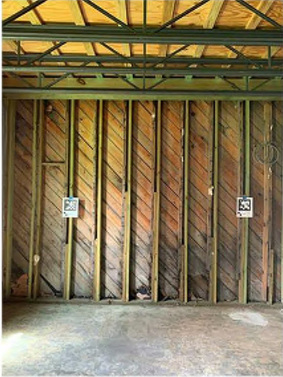
2 EXISTING STRUCTURAL FRAMING AT EXTERIOR WALL ALONG CANAL STREET IN CHURCH ADMINISTRATION SPACE. WATER DAMAGED SHEATHING AND STRUCTURE TO BE CUT OUT AND REPLACED (RE: ASSEMBLY TYPES, PLAN).
