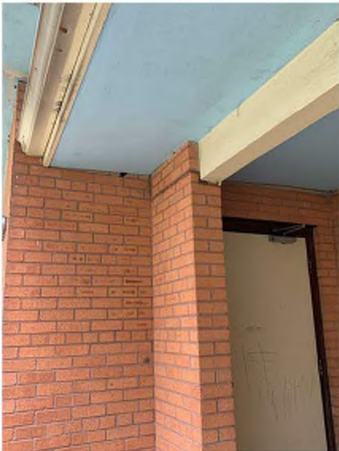
9 EXISTING LOGGIA ENTRY TO LOBBY SHOWN (CANAL STREET FACADE, LOOKING TOWARD S. TELEMACHUS STREET FROM PARSONAGE). EXISTING HOLLOW METAL DOOR TO BE REPLACED WITH IMPACT RATED STOREFRONT SYSTEM AND GLAZING (RE: DOOR SCHEDULE).
