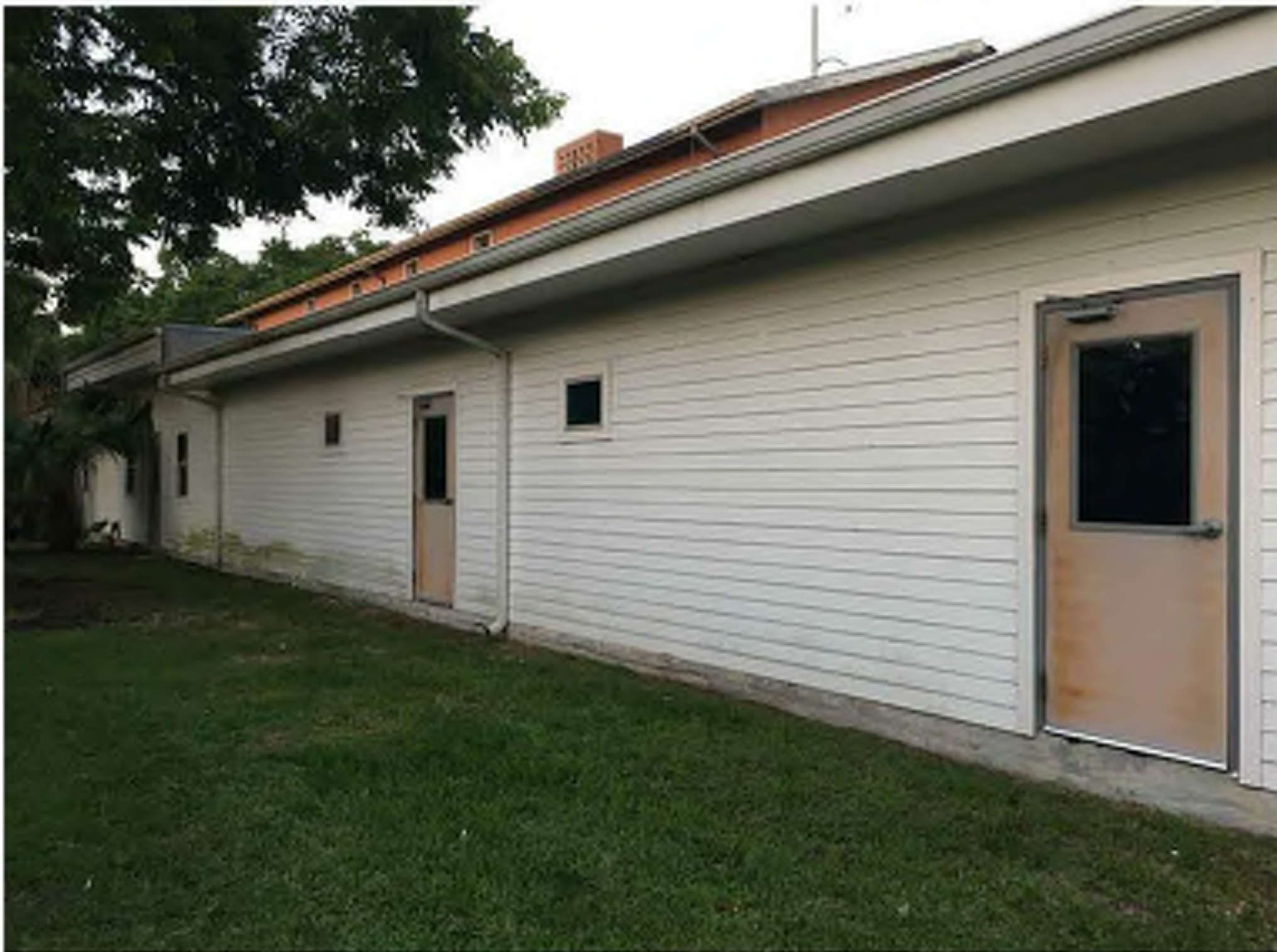
5 SECONDARY FACADE (HIDDEN FROM PUBLIC RIGHT OF WAY) ON S. CORTEZ ST. SIDE WITH NON-HISTORIC H.M. & VINYL OPENINGS. FIBER CEMENT SIDING. OPENINGS TO BE MODIFIED, RELOCATED, AND REPLACED (RE: BUILDING ELEVATIONS) WITH RECEIVE NEW WINDOWS. NEW ENTRY WALKWAY TO BE INSTALLED WITH PLANTING. ROOFS, GUTTERS, AND DOWNSPOUTS TO BE REPLACED IN KIND IN SAME LOCATIONS.
