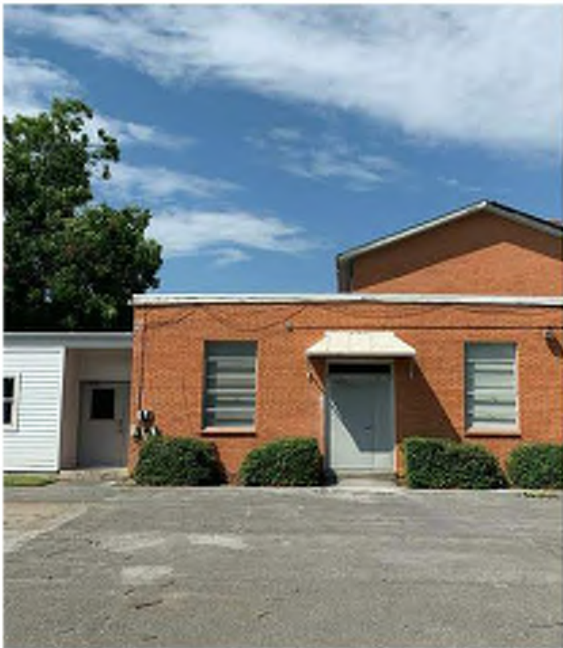
5 SECONDARY FACADE (HIDDEN FROM PUBLIC RIGHT OF WAY) ON S. CORTEZ ST. SIDE WITH NON-HISTORIC H.M. & VINYL OPENINGS. FIBER CEMENT SIDING. OPENINGS TO BE MODIFIED, RELOCATED, AND REPLACED (RE: BUILDING ELEVATIONS) WITH RECEIVE NEW WINDOWS. NEW ENTRY WALKWAY TO BE INSTALLED WITH PLANTING. ROOFS, GUTTERS, AND DOWNSPOUTS TO BE REPLACED IN KIND IN SAME LOCATIONS.
