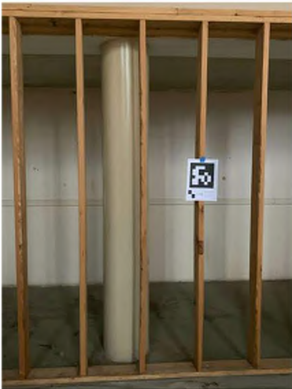
6 EXISTING NON-HISTORIC STUD FRAMING IN SANCTUARY TO BE DEMOLISHED (RE: DEMO PLAN).
