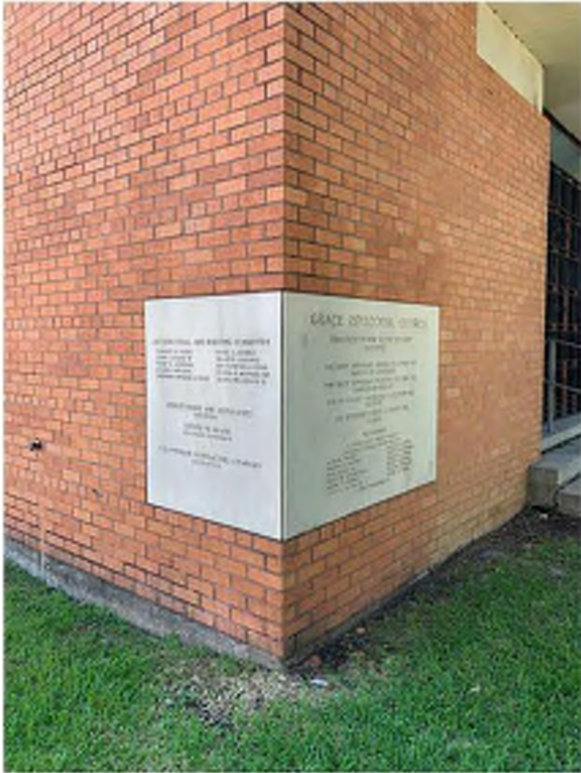
4 CORNER OF CANAL STREET FACADE AND S. TELEMACHUS STREET FACADES. EXISTING HISTORIC CAST-STONE CORNERSTONE TO REMAIN. BRICK AND CAST STONE TO BE CLEANED AND REPAIRED AS NOTED (RE: BUILDING ELEVATIONS).
