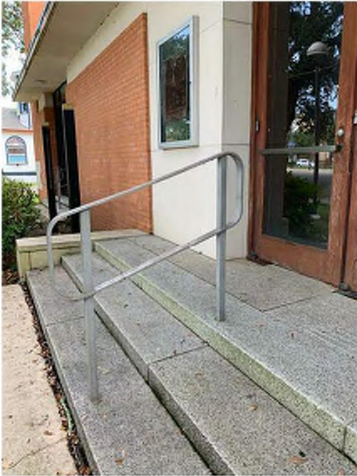
3 CANAL STREET ENTRY TO WORSHIP SPACE. BRICK AND CAST STONE TO BE CLEANED AND REPAIRED AS SHOWN (RE: BUILDING ELEVATIONS). EXISTING HANDRAILS TO REMAIN. DAMAGED WOOD STOREFRONT ASSEMBLY TO BE REPLACED IN KIND TO MATCH EXISTING PROFILES.
