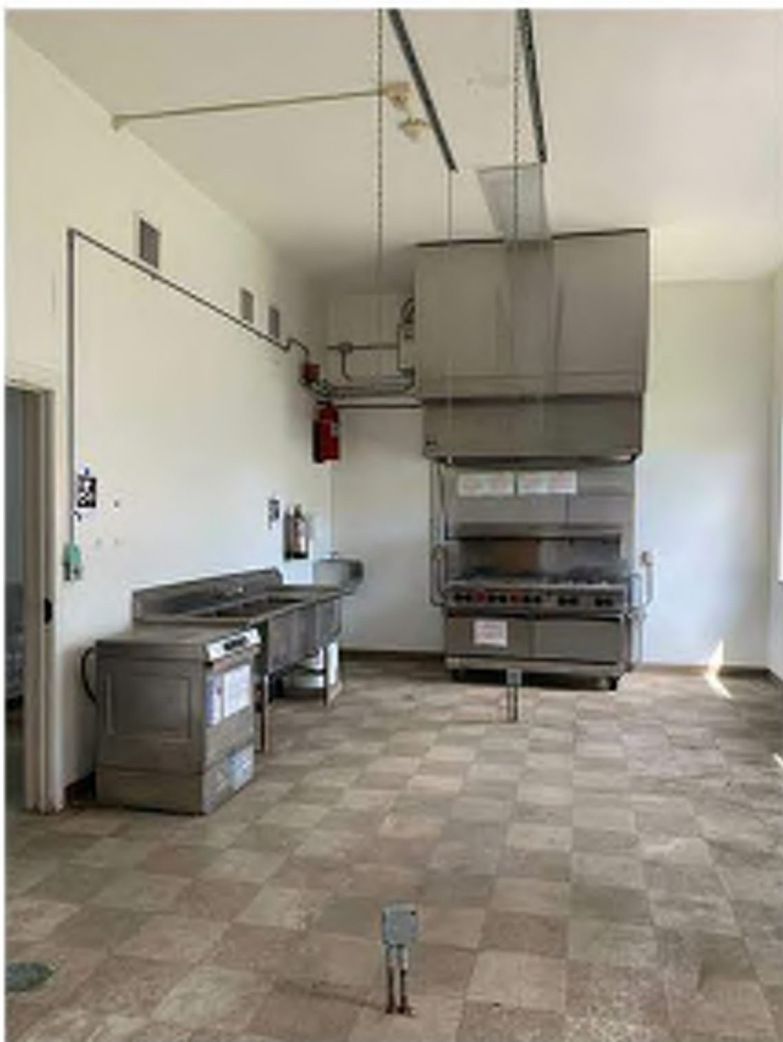
14 EXISTING KITCHEN RANGE, STOVETOP, HOOD TO BE RESERVED FOR REUSE. EXISTING 3 COMPARTMENT SINK, SINGLE HAND SINK, AND DISHWASHER TO REMAIN. EXISTING CEILING TO BE REMOVED AND REPLACED WITH NEW KITCHEN ZONE ACT CEILING (RE: RCP). EXISTING VINYL TILE TO BE REMOVED AND CONCRETE SLAB TO BE REFINISHED AS FINISHED FLOOR.
