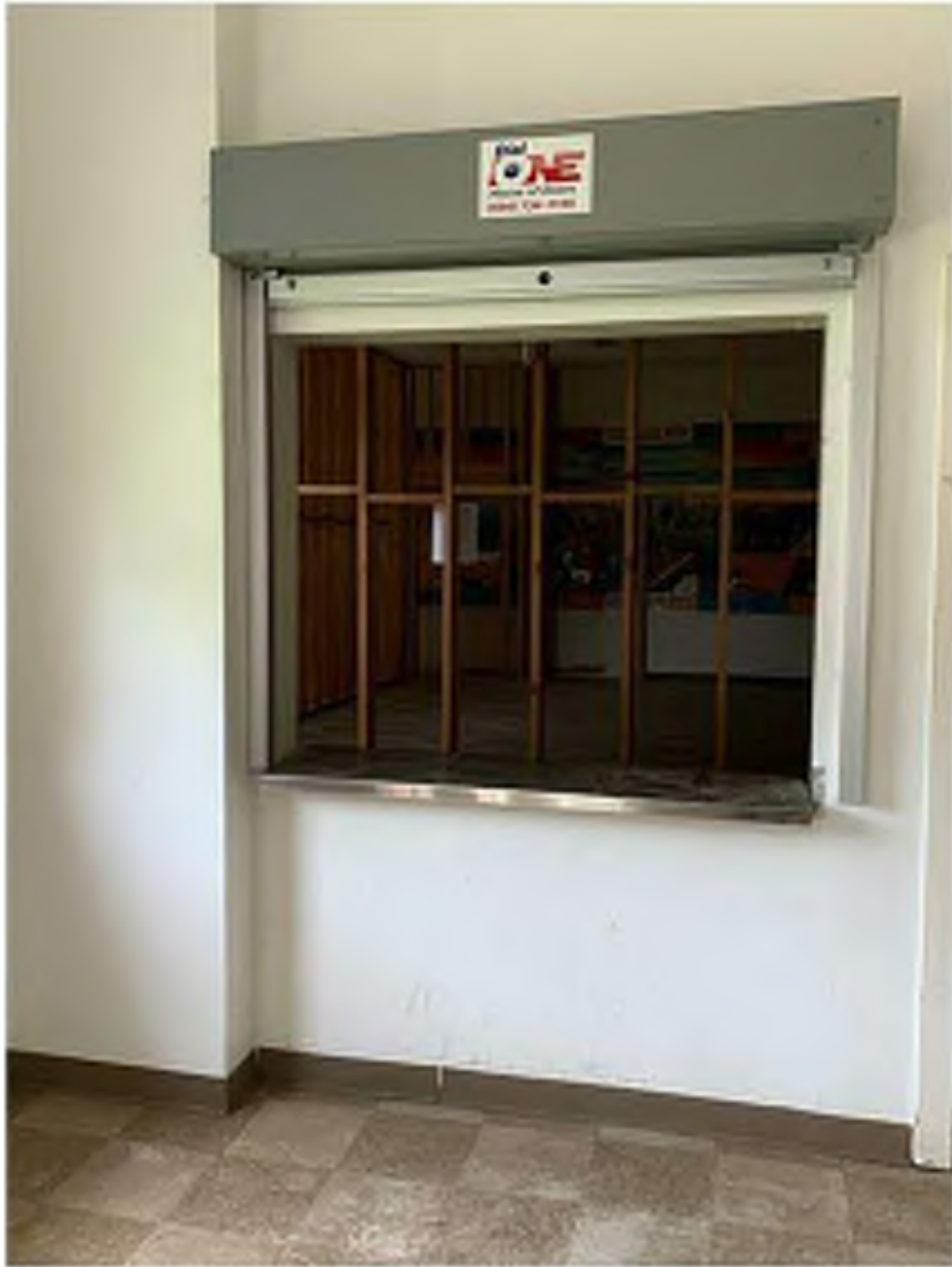
4 EXISTING PASS-THROUGH WINDOW AT KITCHEN TO BE SALVAGED. OPENING TO BE FILLED IN TO MATCH ADJACENT EXISTING.
