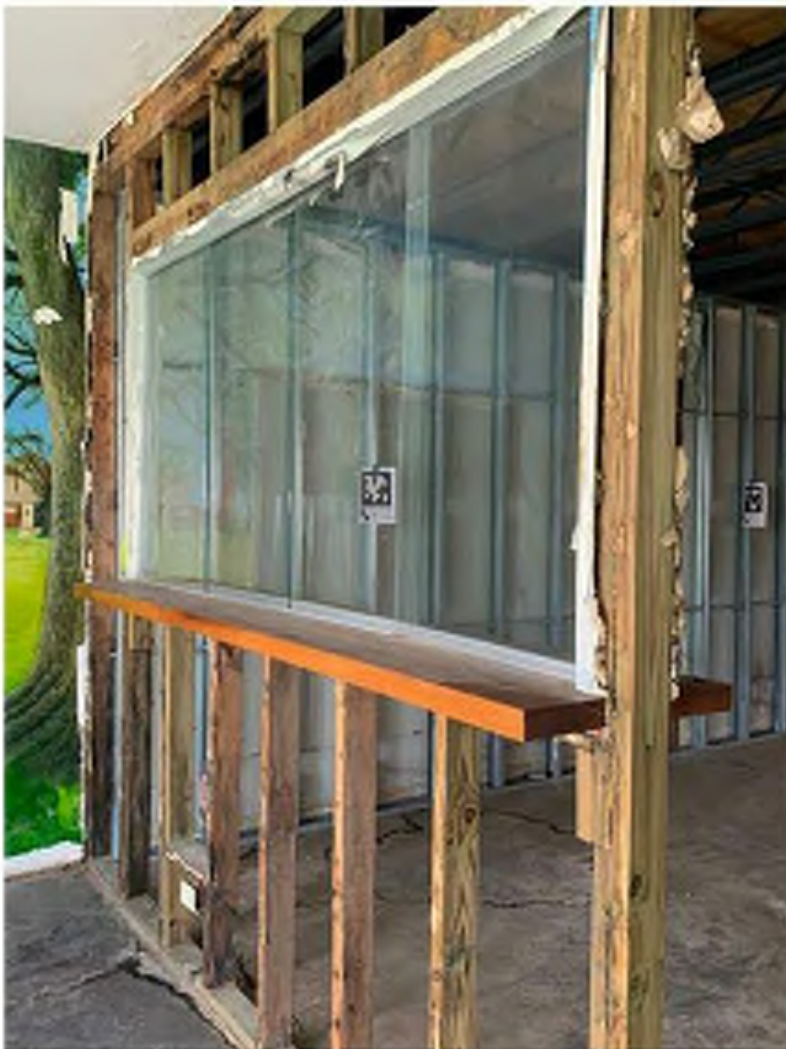
8 EXISTING NON-HISTORIC INTERIOR FRAMING AND GLAZING IN LOBBY ENTRY VESTIBULE TO BE DEMOLISHED. (RE: PLAN)
