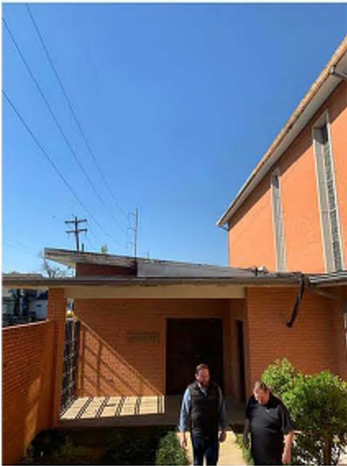
2 INTERNAL COURTYARD LOOKING TOWARD CLEVELAND AVENUE. NEW LANDSCAPING / PAVING @ INTERNAL COURTYARD. METALWORK GATE TO BE LEAD ABATED, CLEANED AND REPAINTED. EXISTING CHAPEL DOOR TO BE REPLACED WITH GLAZED DOOR IN EXISTING OPENING. MECHANICAL SYSTEMS AT RIGHT TO BE REROUTED, BRICK TO BE PATCHED TO MATCH EXISTING ADJACENT.
