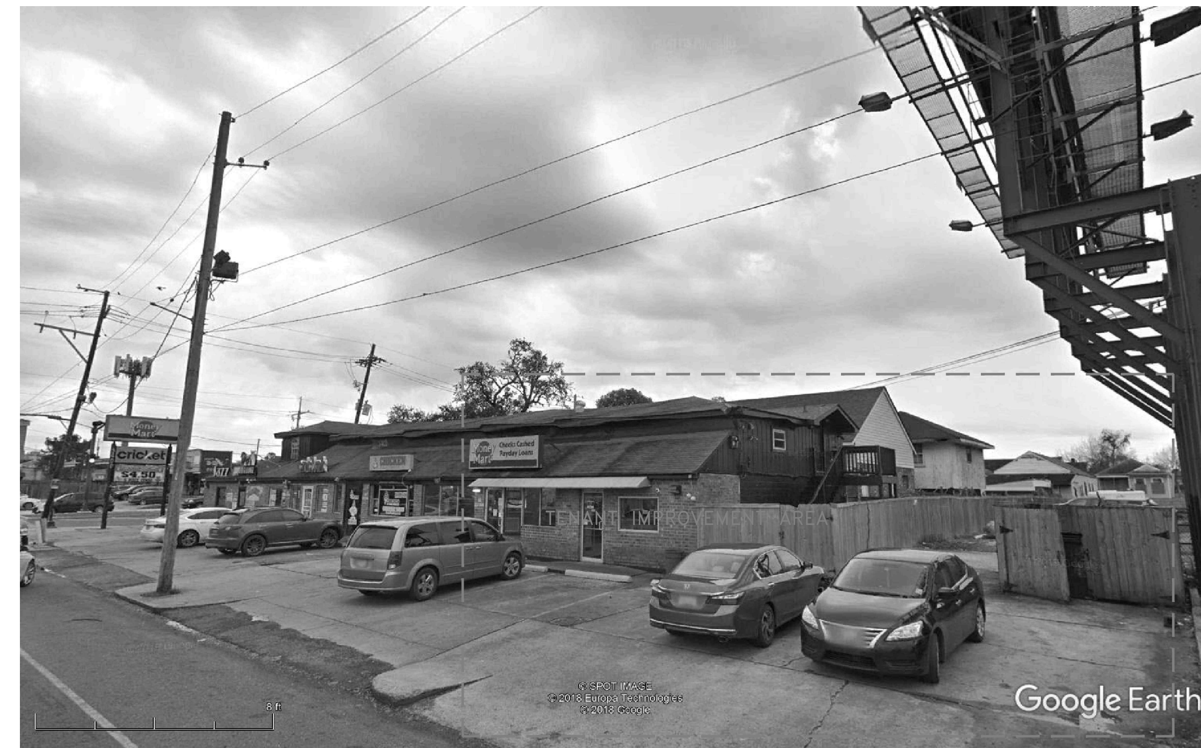
EXISTING BUILDING-AREA FOR TENANT IMPROVEMENT
