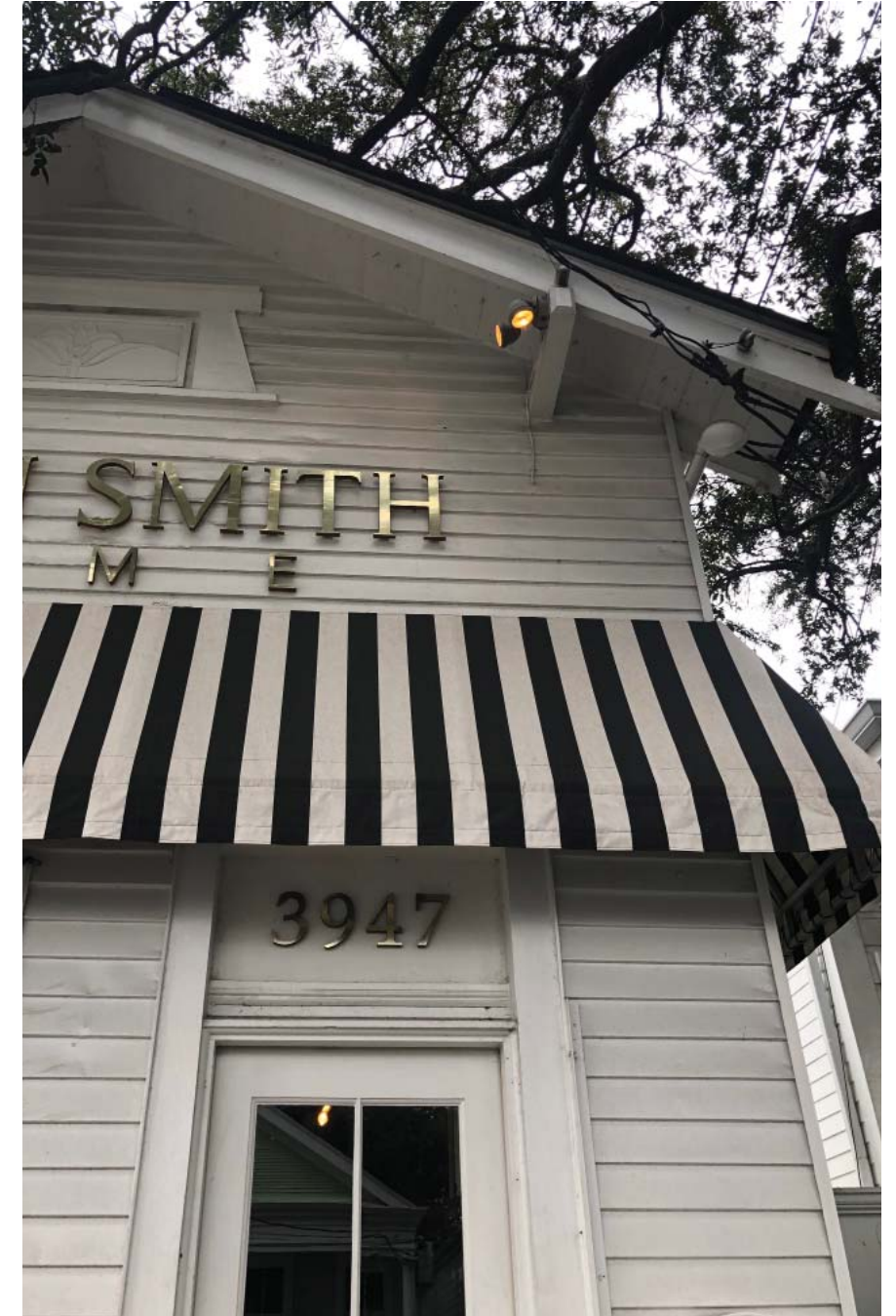
VIEW OF ROOF OVERHANG FROM MAGAZINE STREET
