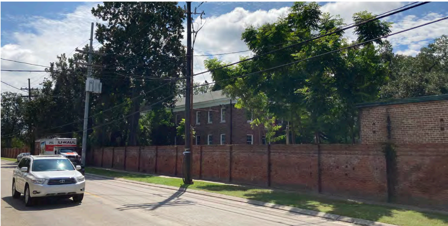
EXISTING BUILDINGS - B4 AND B5 TCHOUPITOULAS SIDE
