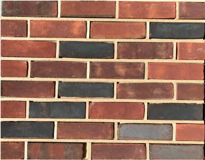
BRICK MATCH - GLEN GERY 35% - RED 35% - PURPLE 20% - BLACK 10% GREY MORTAR JOINTS TO MATCH
