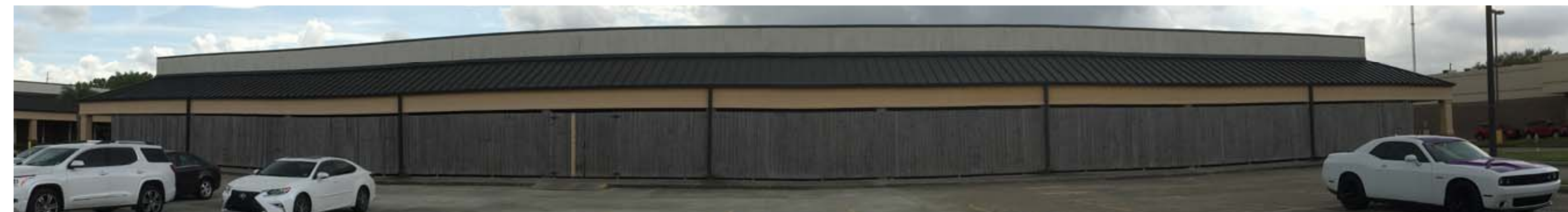
3 PH1 BUILDING 'B' REAR
