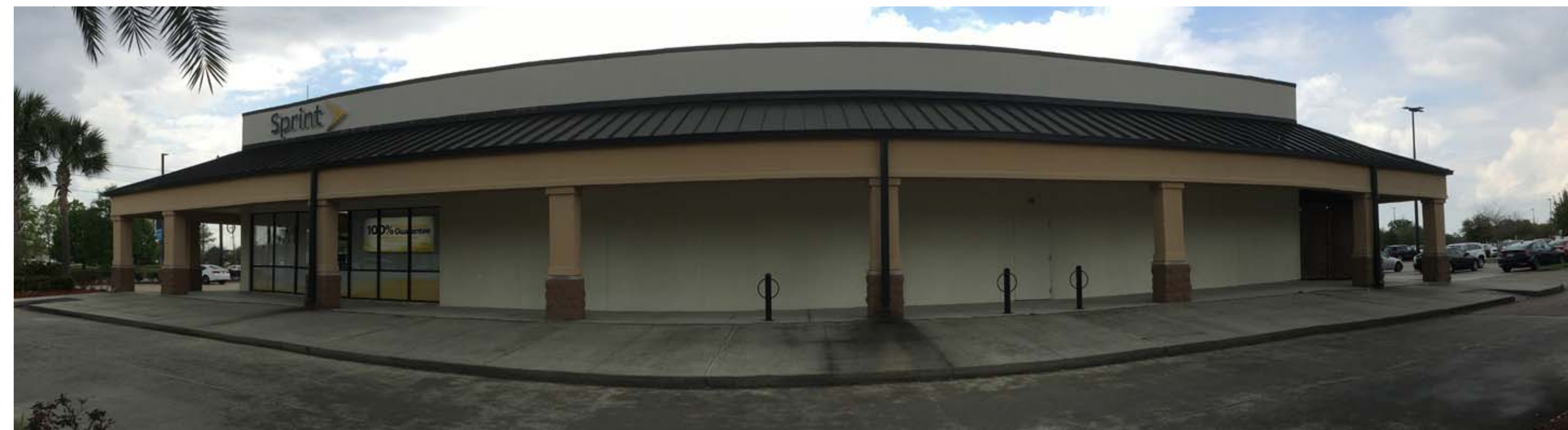
4 PH1 BUILDING 'B' RIGHT SIDE
