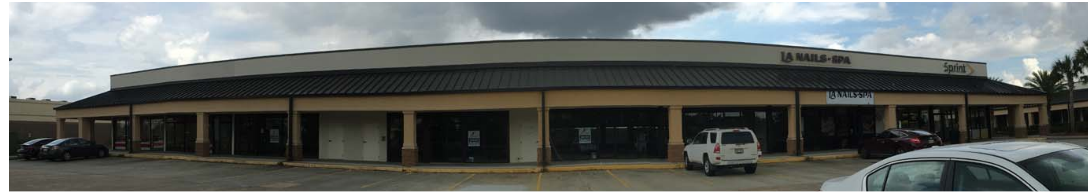
1 PH1 BUILDING 'B' FRONT
