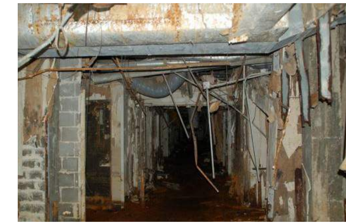
1 INTERIOR - BASEMENT - ORIGINAL HOSPITAL: EAST CORRIDOR MASONRY WALLS TO REMAIN. STRUCTURAL FRAMING TO REMAIN. REMOVE ALL GYPSUM BOARD FINISHES, SUSPENDED CEILING, PIPING, CONDUIT, DUCTWORK, PLUMBING, EQUIPMENT, LIGHTING, ETC. REMOVE ALL DEBRIS.
