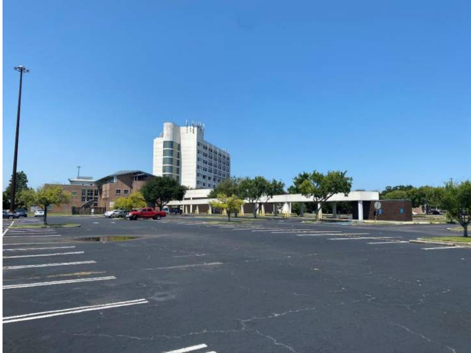
View of existing breezeway towards the northwest.
