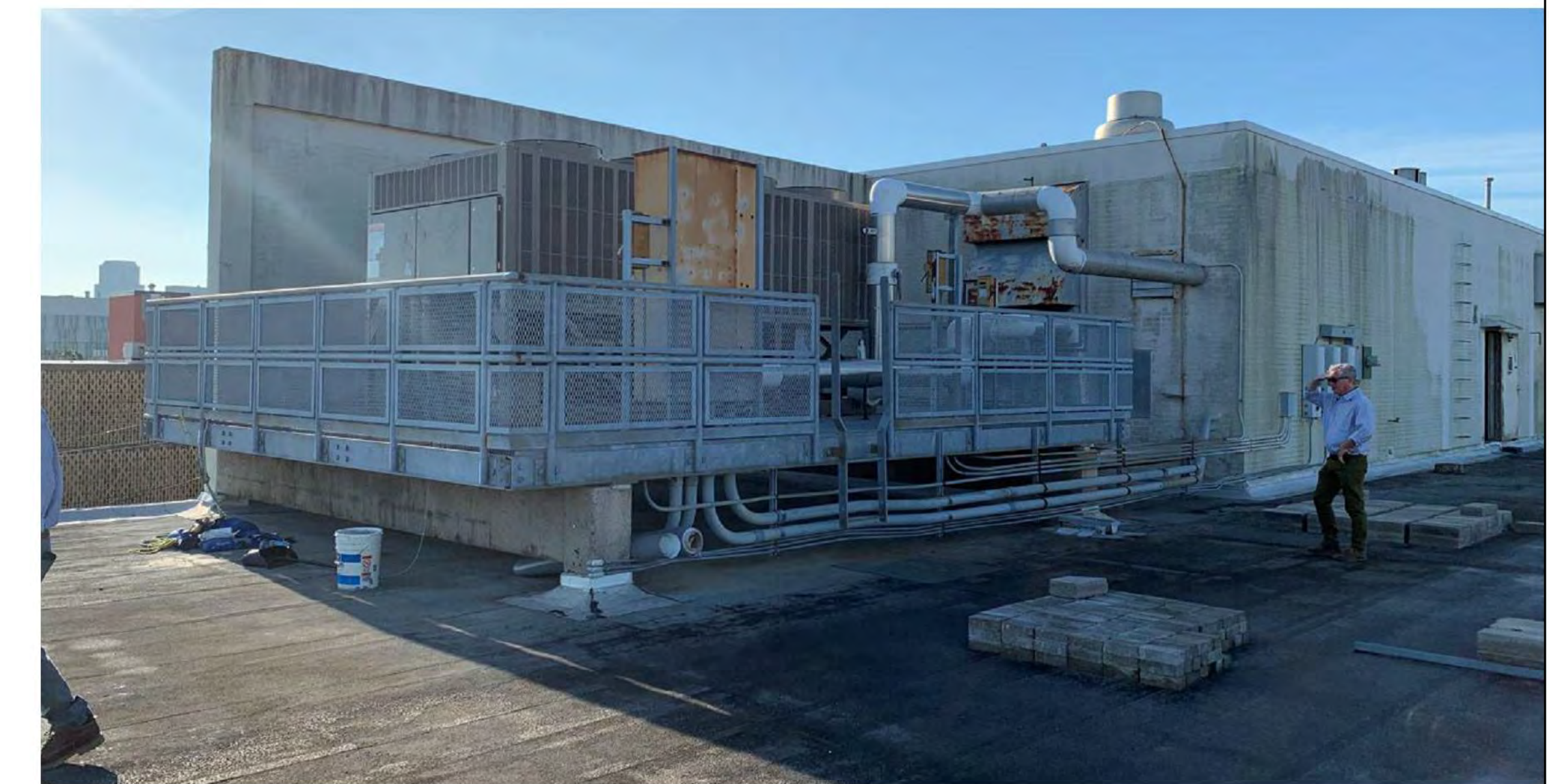
6. EXISTING ROOF MECHANICAL PENTHOUSE AND PLATFORM
