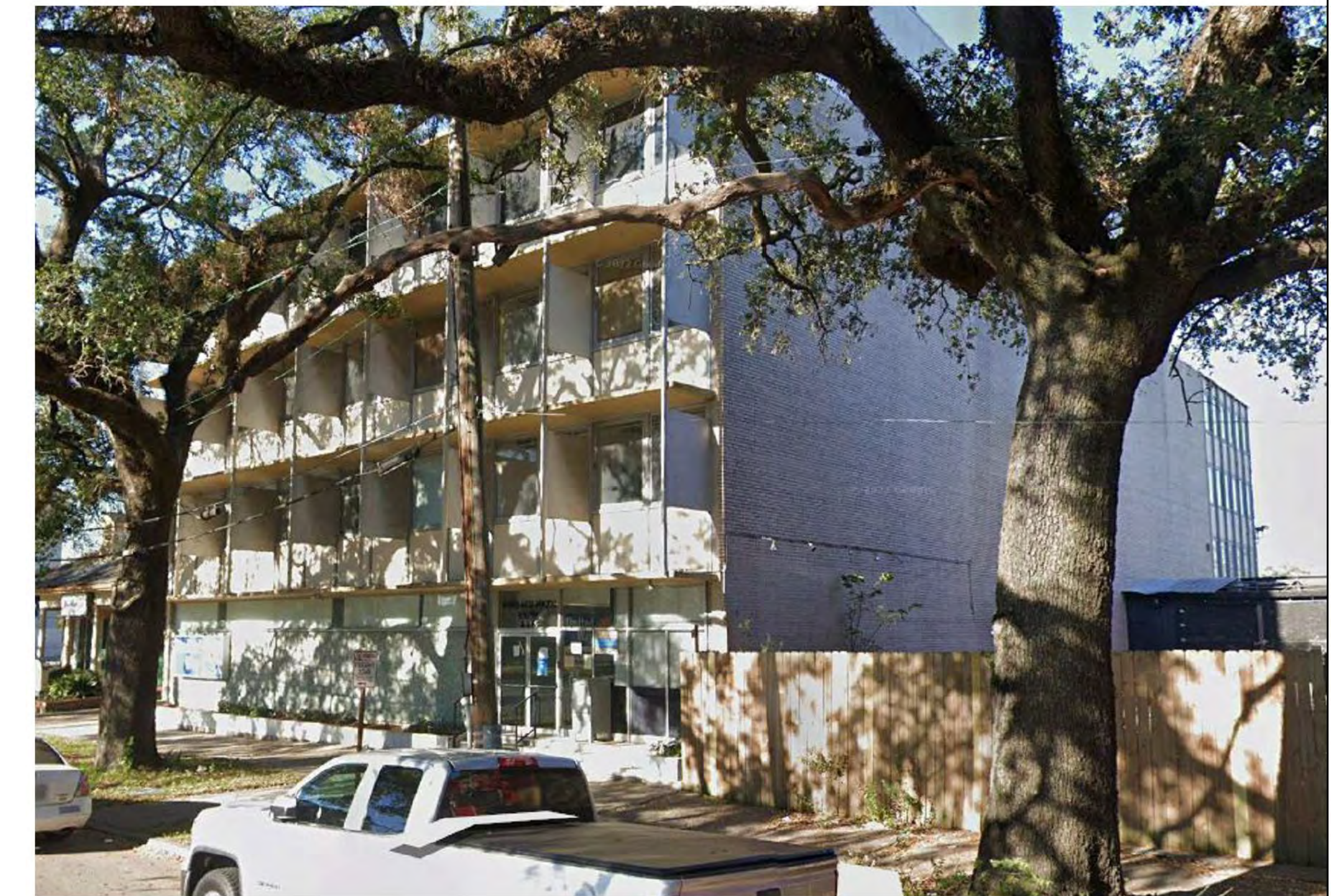
3. VIEW LOOKING NORTH FROM CANAL ST
